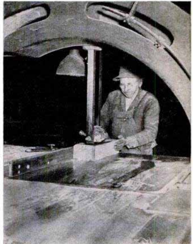
Bandsaw cuts edges of bearing pieces so they will form Vs for salt-water circulation around the tube
