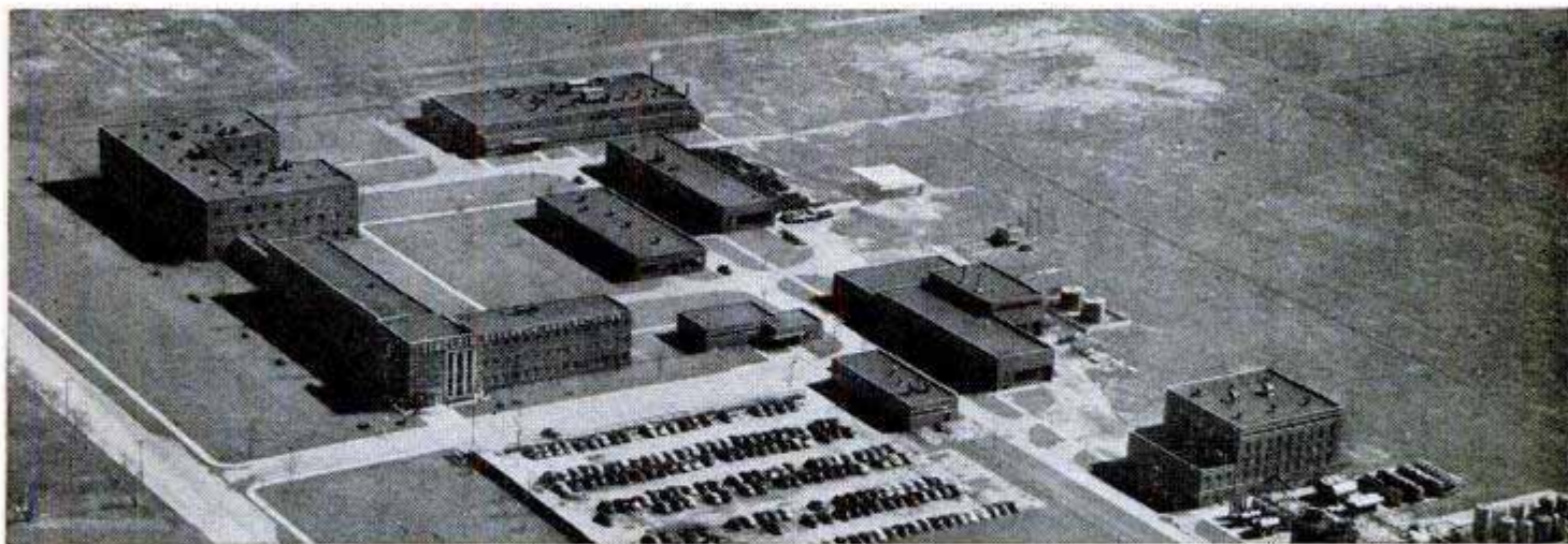
Nine buildings of the Sinclair Research Laboratories at Harvey, Ill.
