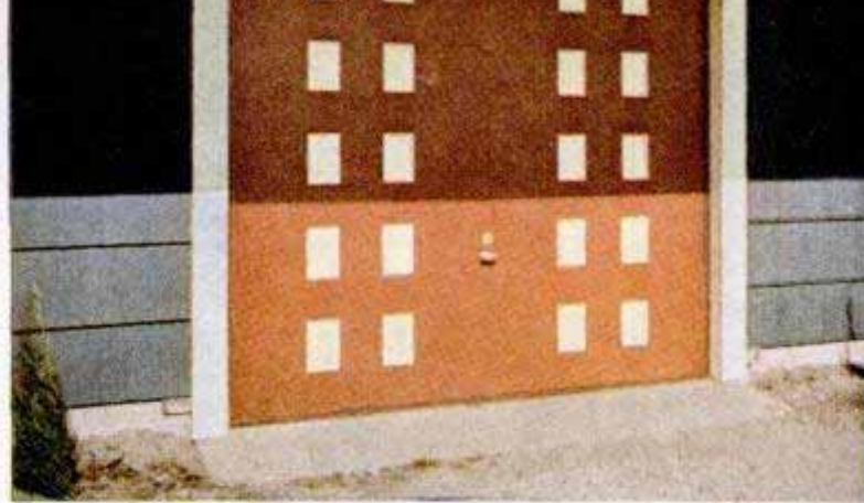
Two vertical groupings of bevel-edge blocks provide another simple and attractive garage-door treatment
