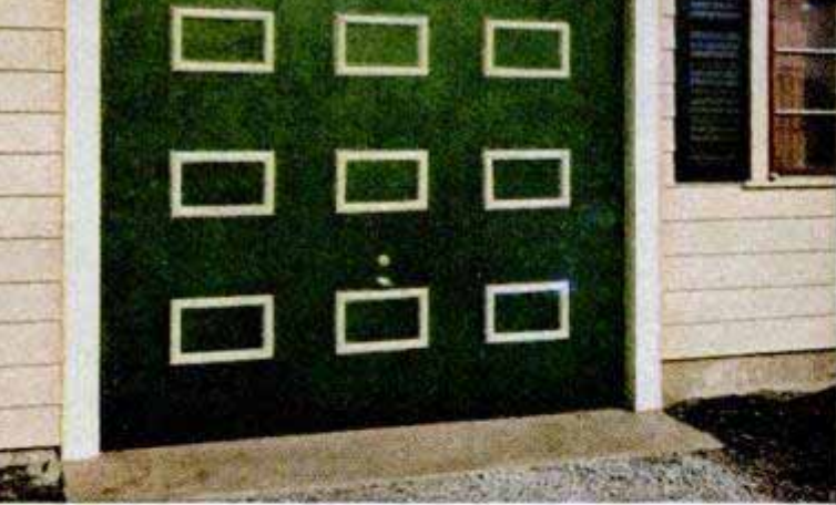
Nine "picture frames" add the final decorative touch to this plain one-piece, upward-acting, garage door
