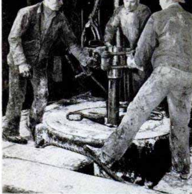
One of the big natural-resource quests of today is for oil. Here a drilling crew is working into night
