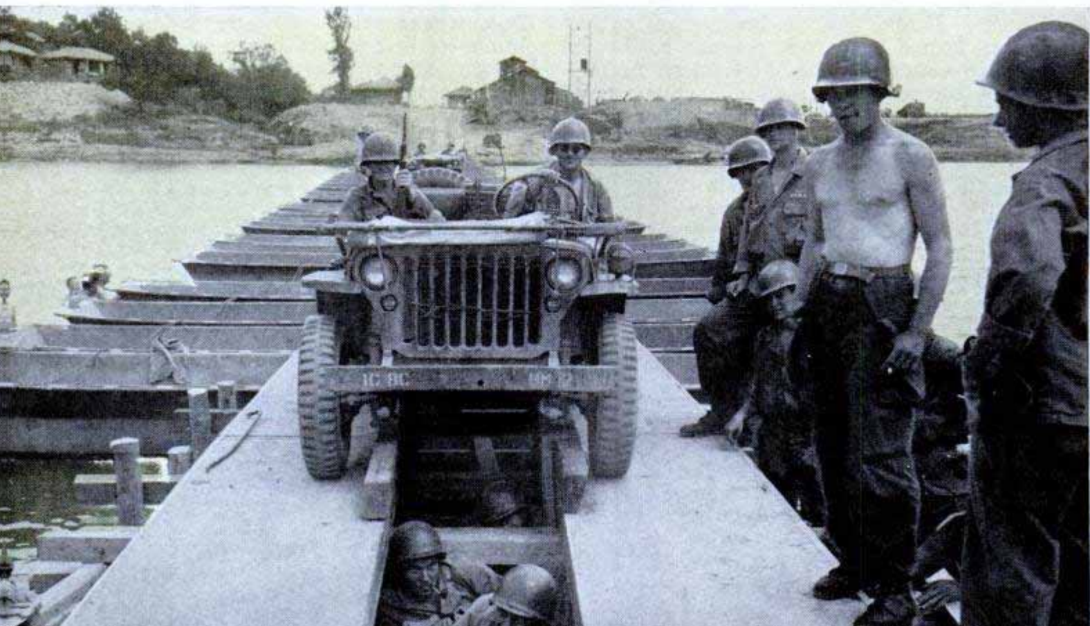
Jeep advances over aluminum treadway paths bolted to steel assault craft with timber supports near shore
