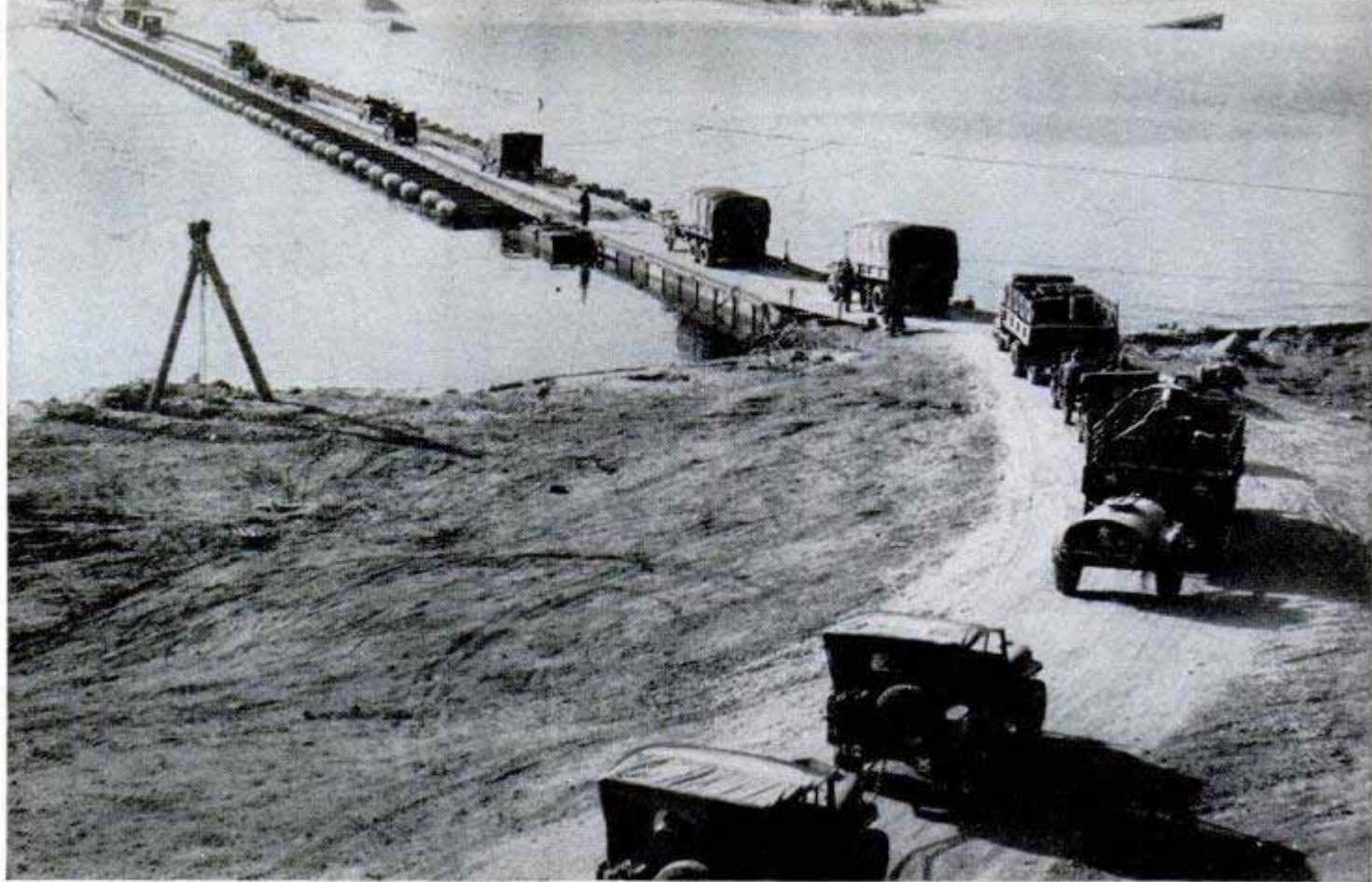
This pontoon bridge across the wide Han River in Korea was built in a few hours by U. S. Army engineers
