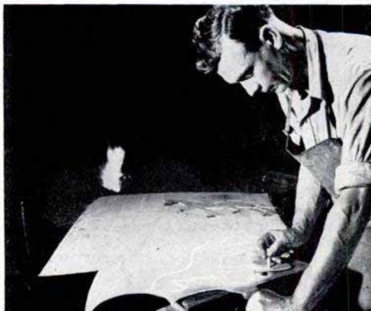
Below, the special chalk that Boone uses to trace the pattern will not disappear in the high heat of the forge
