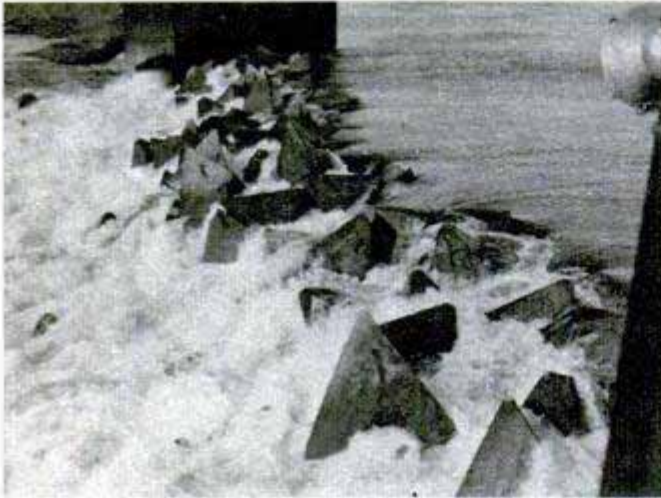
Above, close-up of the four-faced concrete castings in position across the gap. Below, the tetrahedrons were cast at the dam site in forms like this one. Below right, one of the "tets" on its way to the dam
