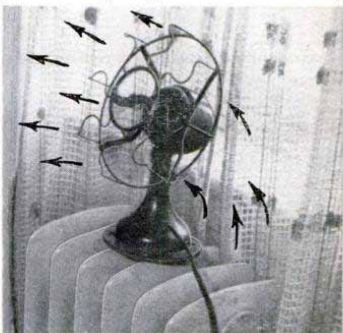
Placed on radiator, the fan in photo below serves much the same purpose as fan on warm-air register. Even though directed upward, fan keeps room temperature even by forcing warm air down from ceiling
