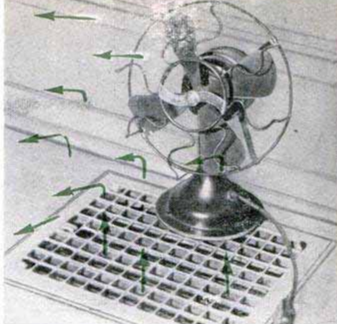
Fan set on warm-air register gives occupants full benefit of heated air by directing it across room at "living level." Fan pictured below speeds gravity circulation by blowing air into cold-air register
