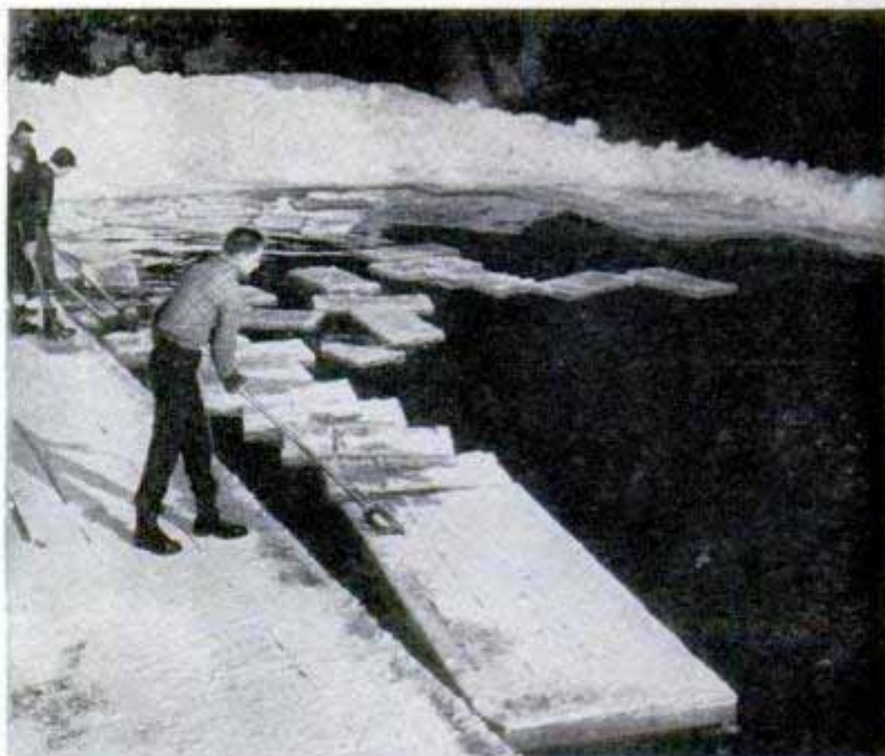
Large sections are broken into blocks by driving a heavy chisel into score cuts made by the power saw
