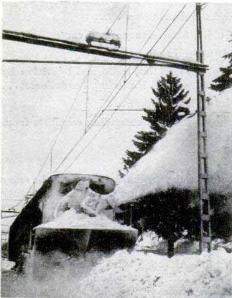
Novel snowplow is mounted on a turntable, which in turn is mounted on a single truck. No need for a "Y" in the tracks to reverse the plow—two men merely revolve it on turntable
