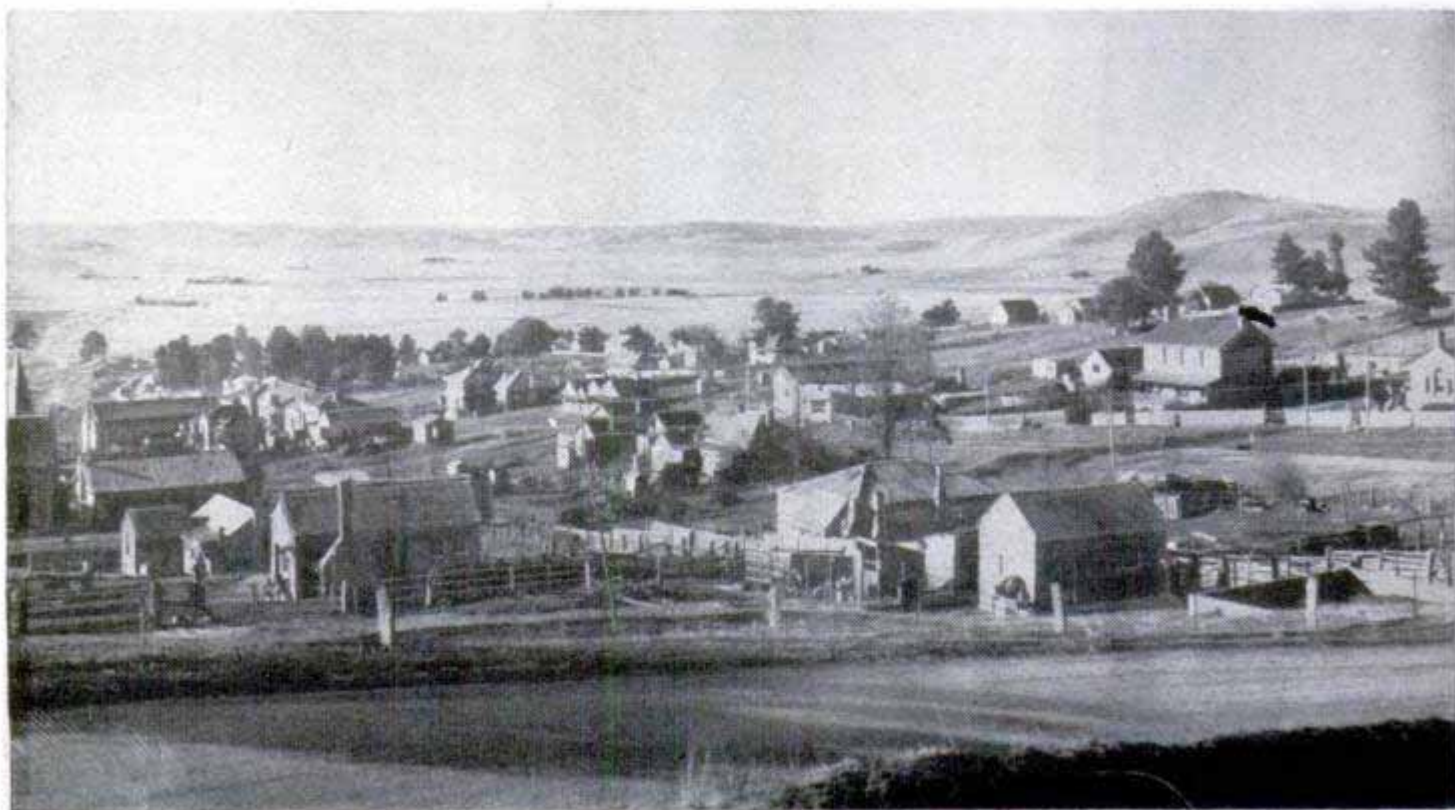
West end of the Tumut project is Adaminaby Reservoir which will submerge part of this 400-inhabitant village
