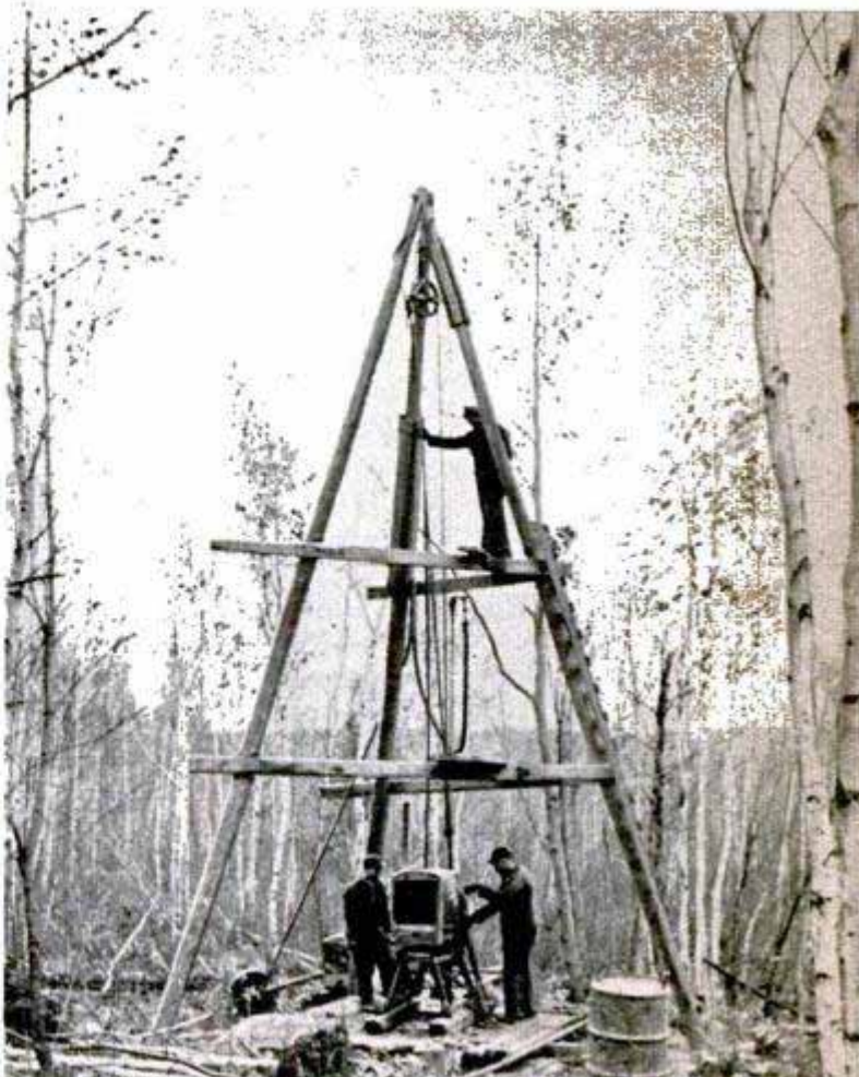
With these rigs, miners are test-drilling all over the iron range to learn extent of the taconite deposit
