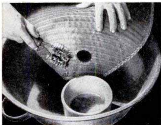
Hood and body of woven fiber are scrubbed thoroughly with soap and water, as above. Rinse off soap and, while fiber is still wet, remove any dents. After fiber dries, paint it the desired color by coating with well-thinned auto lacquer or model-airplane dope
