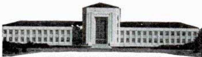
EZEKIEL W. CULLEN BUILDING
