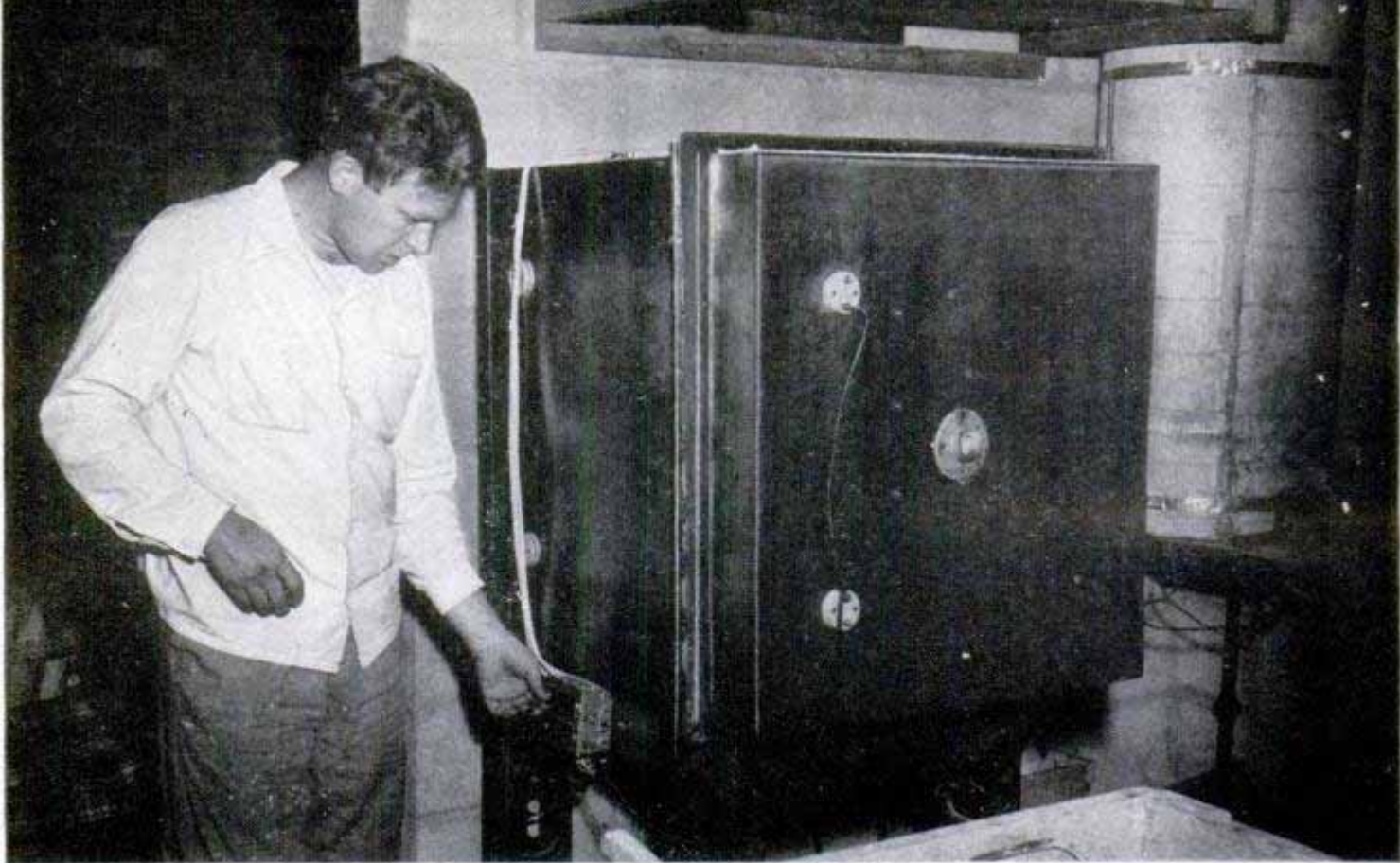
Kiln made of junked parts cost $70, now is valued at $1000. Six electric switches give precise heat control
