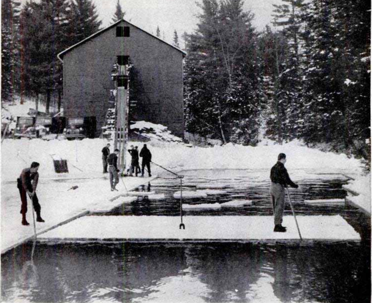
Ice is floated to the loading end in large sections, which are broken into blocks before going up the chute
