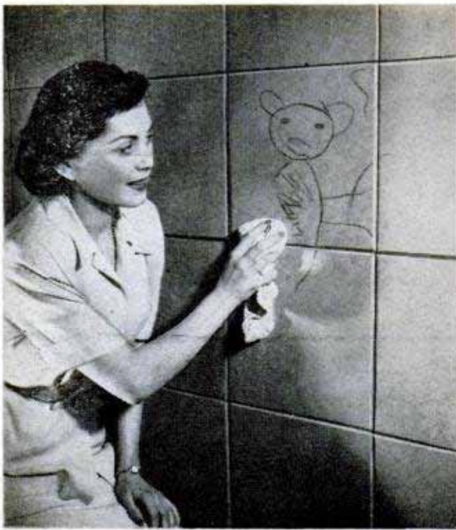
Crayon marks, food stains and grease spots can be wiped off the plastic covering with soap and water
