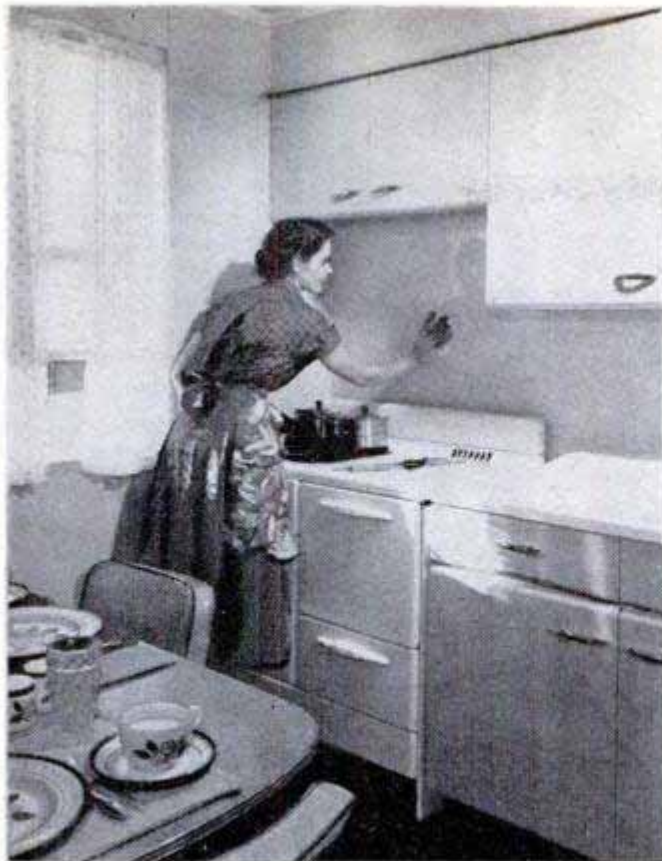
Panels resist stains, wipe clean with a damp cloth. Above right, plastic-surfaced molding frames windows. Right, molding strip holds panels, covers joint
