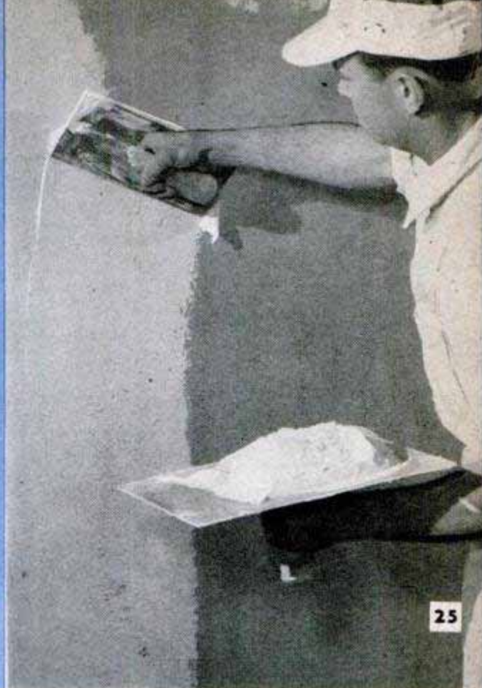
LONG FLOAT, OR DARBY, FOR LEVELING LARGE AREAS OF PLASTER
