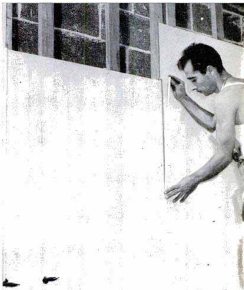
Panels resist stains, wipe clean with a damp cloth. Above right, plastic-surfaced molding frames windows. Right, molding strip holds panels, covers joint
