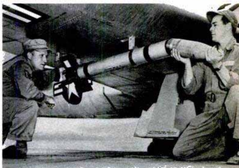
Attaching warhead to a 5-inch rocket under the wing of an F-84. These and napalm are two of the most deadly agents used in close support of troops
