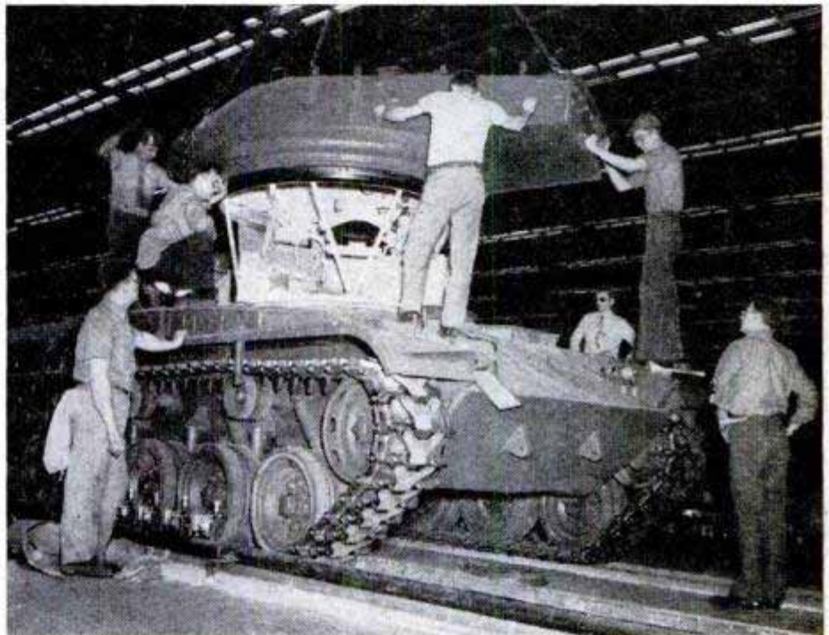
Dropping the turret and its "basket" into the lower part of the tank. A skilled producer of tanks in World War II, Cadillac is making the T-41 at its plant on the edge of Cleveland. Below, mud, deep ruts, steep inclines or sand do no more than slow down the Bulldog's 51,000 pounds
