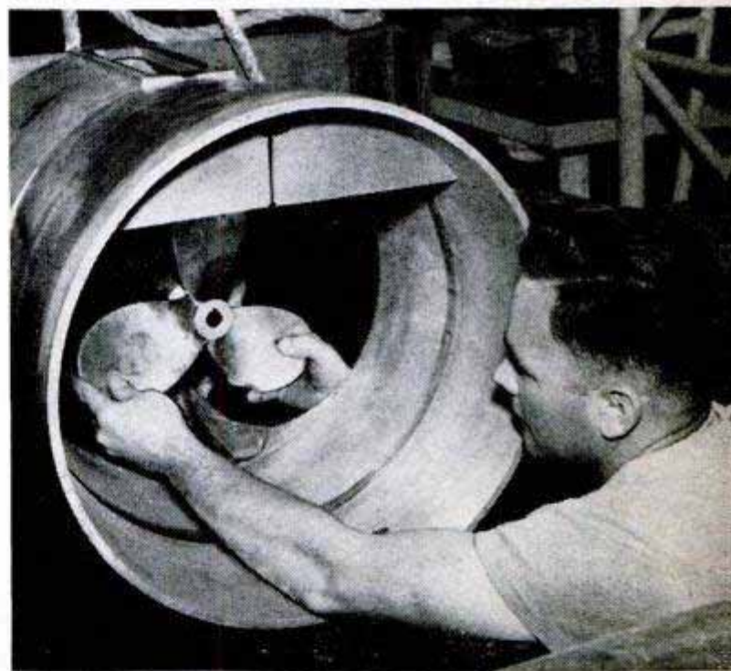
Nylon-rubber fabric pops out from under the cylinder cover, expands around cylinder to form rescue craft
