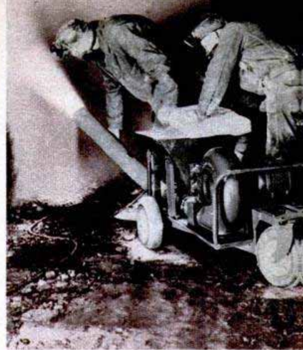
At the bureau's test mine, engineers duplicate the frightening spectacle of a live coal-mine fire. Instruments record temperatures up to 3000 degrees. Right, dusting machine spouts powdered limestone into burning mine
