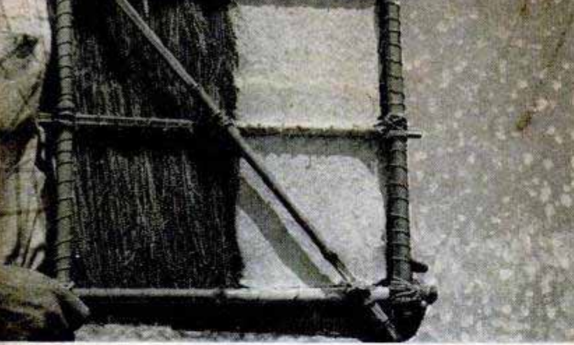
Since Plasmoite sticks to anything, it will make an ideal coating for cheap tropical housing. Half of straw-thatch panel is coated. It's now waterproof, bugproof, stronger
