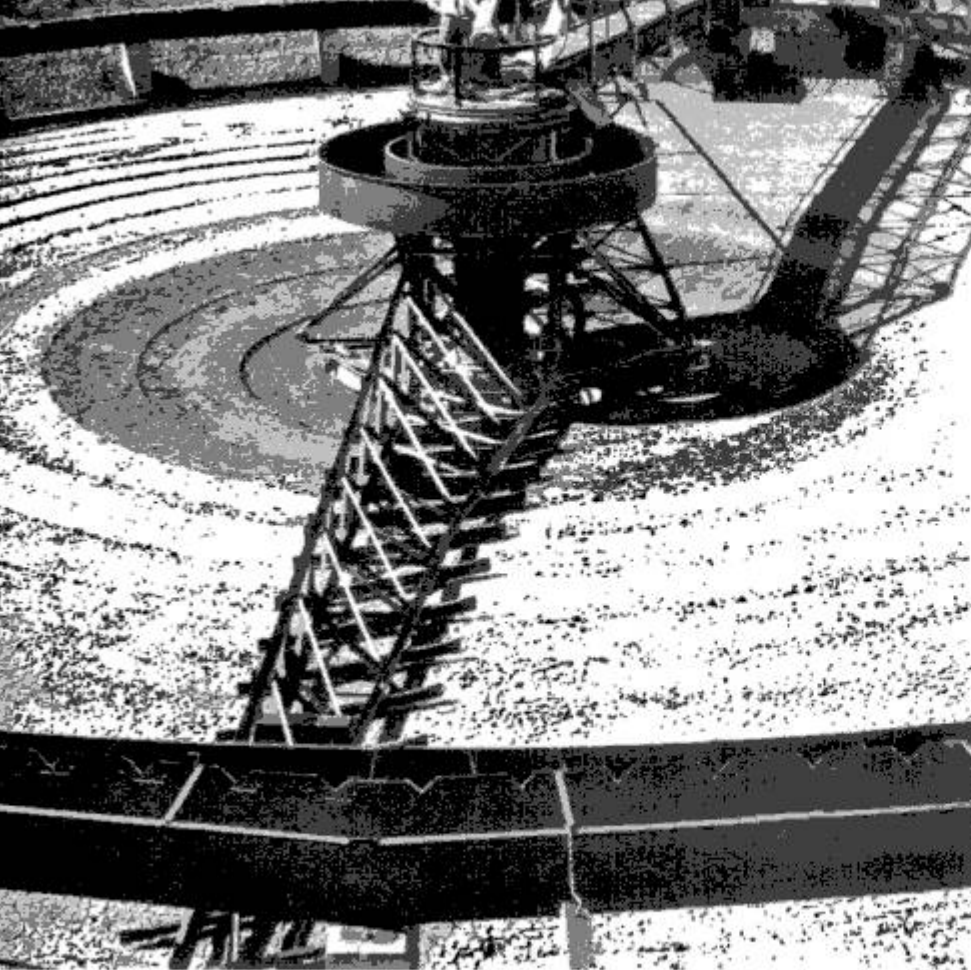
With basin dry, blades of a rake arm can be seen. They scoop the mud to the center of the big basin
