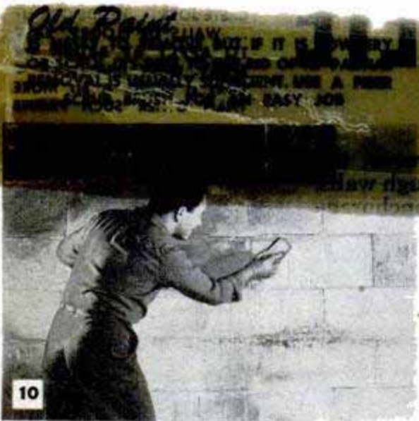
REMOVE WHITWASH AND CALCIMINE WITH HOT WATER. USE 20-PERCENT SOLUTION MURIATIC ACID FOR WATER-RESIN PAINT
