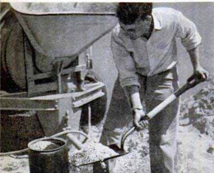
For \frac{1}{2} -bag mixes, a bag of portland cement can be divided equally by using two pails of the same size. With a ruler, measure from the rim to the top of the cement to be sure that the level is the same in both pails. Then mark one for use as a measure
