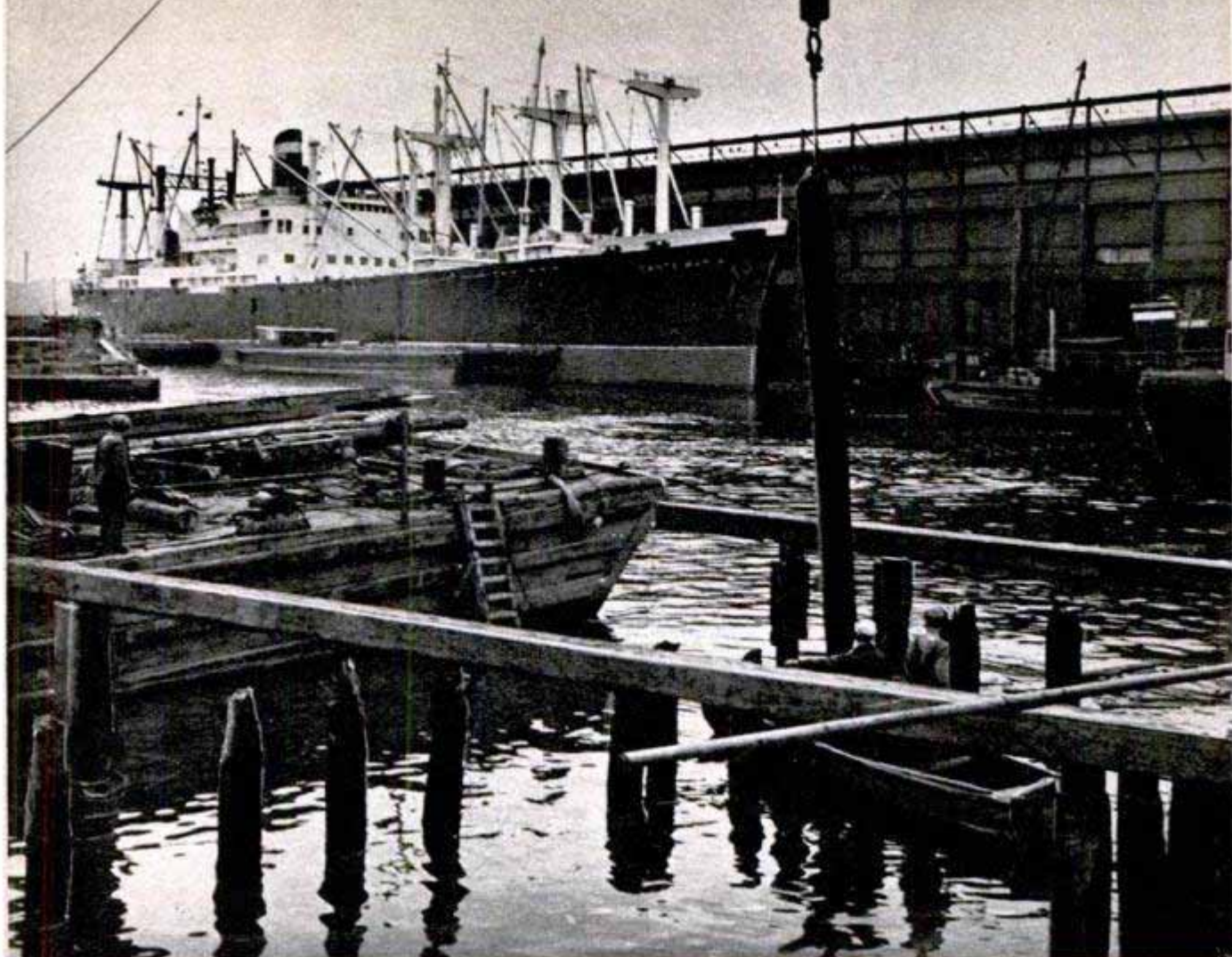
"Timber!" Working in boats, these lumberjacks cut timber, but it doesn't fall — it's hauled up by crane
