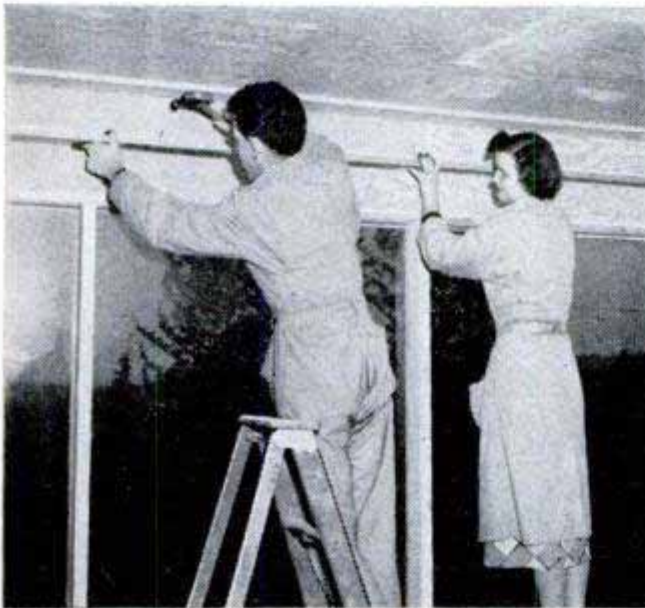
One of the final steps is the dual-purpose valance boards over the large windows in the living room and dining area. Here, Vinita gives me a hand in nailing the shelf which supports fluorescent bulbs
