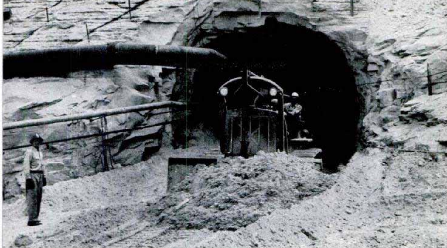
Bulldozer excavates a huge cave which will be one "target" of a mammoth TNT charge exploded above it
