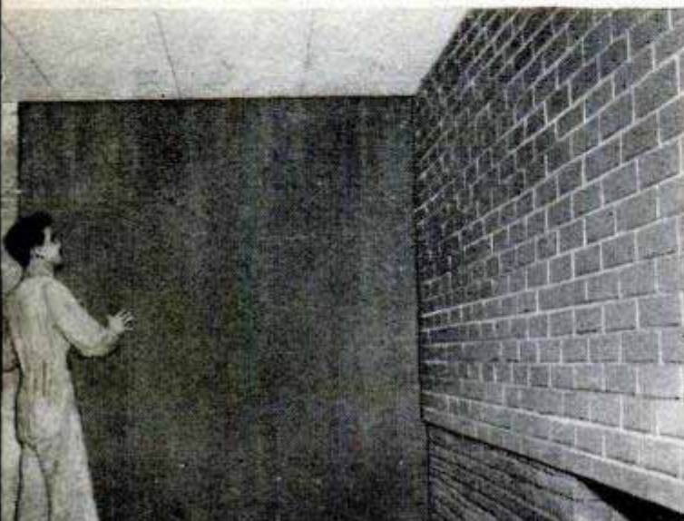
Above, the ceilings were finished with a thick coat of texture paint, stippled with a flat sponge. Below, walnut-faced plywood on one wall of the living room gives pleasing contrast to vertical-grain fir paneling
