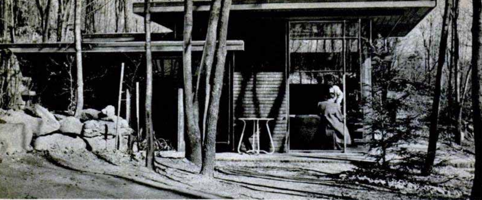
Two full walls of the living room are plate glass. Overhang passes sunlight in winter but not in the summer
