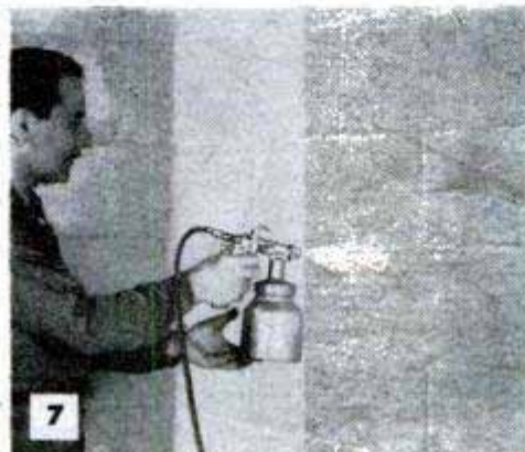
KEEP THE PAINT WET
