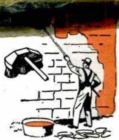
ROOF BRUSH IS HANDY FOR OUTDOOR PAINT APPLICATION
