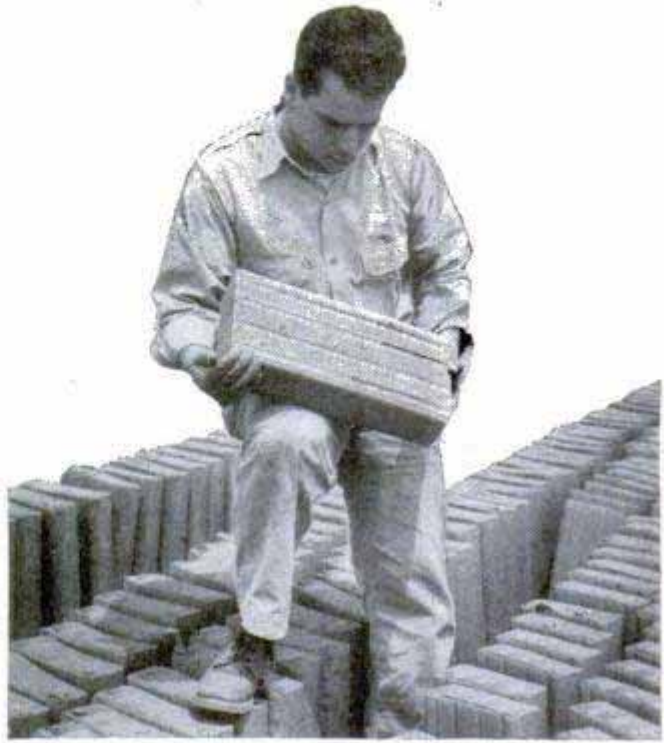
Above, Mission San Gabriel, near Los Angeles, is an adobe structure that was built more than 150 years ago. Right, each adobe brick (weight: 30 pounds) is examined for cracks. These bricks are drying, a process that takes 10 days. Below, a modern relative of mission, above, is a present-day adobe-brick home
