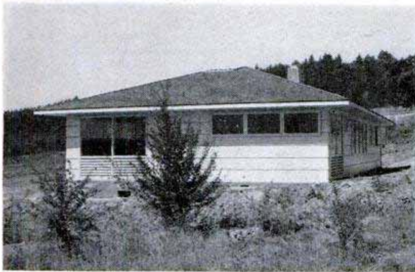
Here is a view of the bedroom end of the house. Note that the window louvers are larger than those in the living room. Both bedrooms feature three "clerestory" windows on one wall which allow beds to be located under them. Right, roof-truss plan is used to lay out the assembly jig on the subfloor. Below, this plan gives location of trusses and shows how hip rafters are tied in
