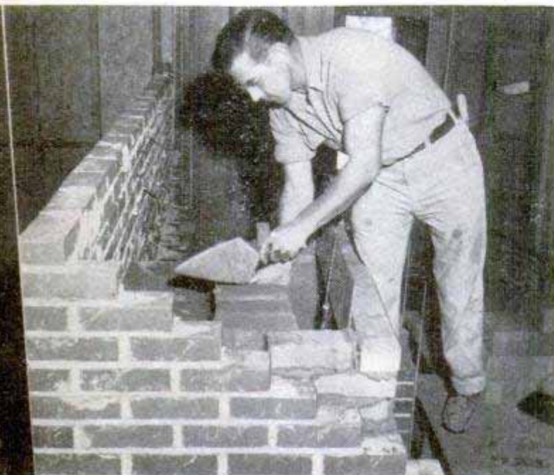
Sheathing the outside with 4 x 8-ft. sheets of plywood goes fast and results in a wall 50 percent stronger than shiplap. Below, R. J. Coffman, Portland brickmason, is laying the "island wall" fireplace
