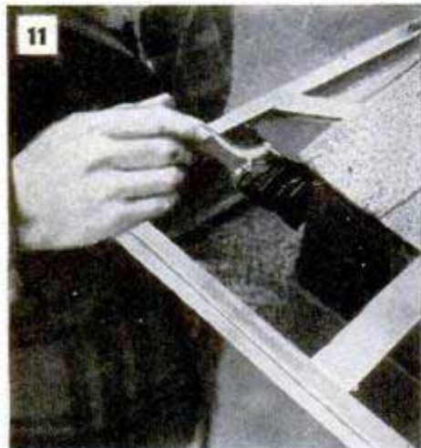
Small breaks in the metal can be closed by a fabric patch. First, apply compound with a brush as in Fig. 11, then press the canvas patch in place as in Fig. 12. Apply final coat over the fabric, including edges
