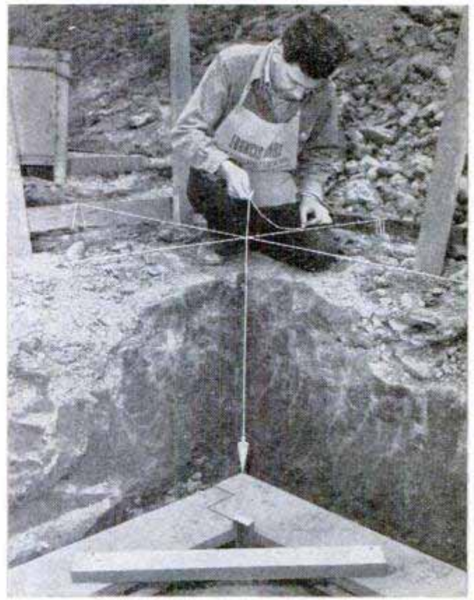
Above, this is the next step after pouring the footings. Here I am checking the inside corner of the anchor plates for the foundation forms. Below, using sheets of \frac{5}{8} -in. plywood, Norman Chapman and I are beginning to erect the forms along rear of house
