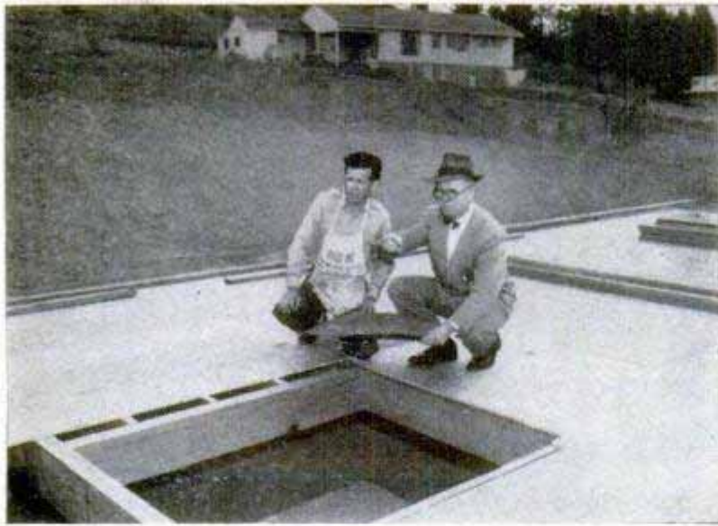
Above, architect Whelan, right, explains how trimmings from plywood subfloor are economically used later as truss gussets. Below, see how fast and easy the subfloor goes down. Plywood sheets previously used for forms are cleaned off and laid so that the joints are staggered four feet on the floor joists
