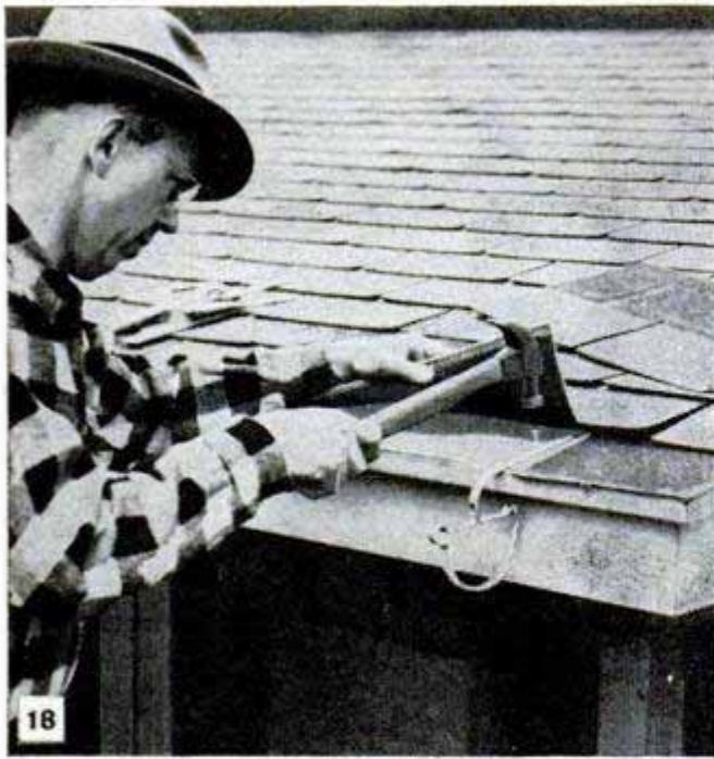
When applying new gutter hangers on old roofs, shingles should be lifted so that hanger can be nailed directly to the roof boards. On asphalt-shingle roofs, the individual shingles are easily removed for this job
