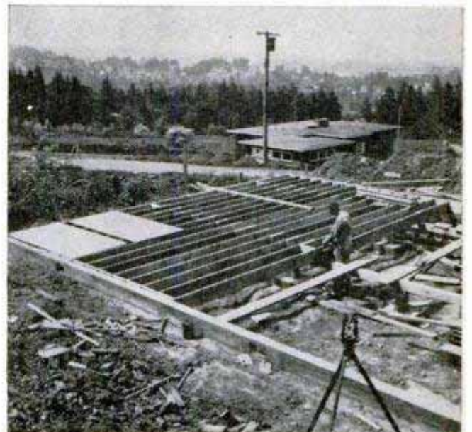
Footings for the beam posts and the "island wall" fireplace, which are 12 in. thick, are poured at the same time as the foundation footings. Below, Norman Chapman, my helper, is spiking the joists
