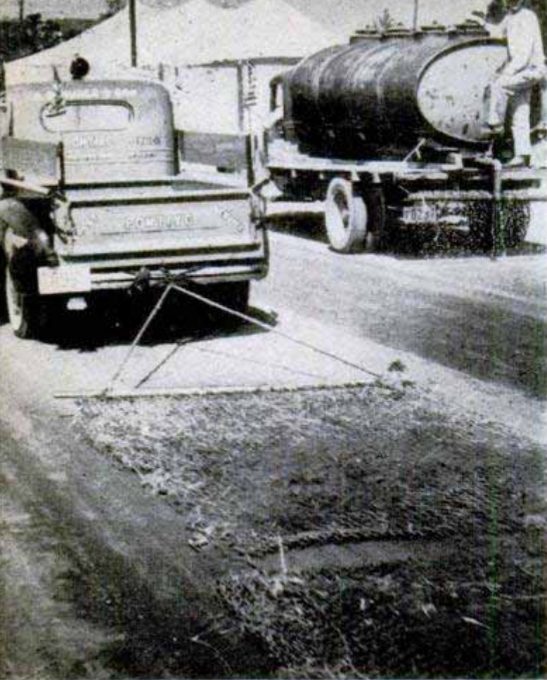
Drags made of wire fencing keep the surface smooth. The sprinkler was made from a dilapidated oil truck
