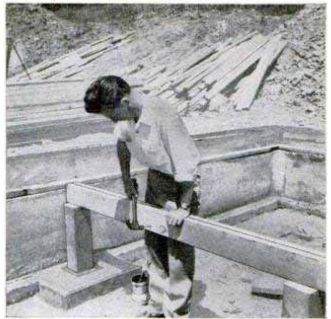
Each beam on which the floor joists rest is built up by spiking together three 2 x 6s on edge. As the joist plan indicates, two separate beams are required
