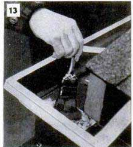
Small breaks in the metal can be closed by a fabric patch. First, apply compound with a brush as in Fig. 11, then press the canvas patch in place as in Fig. 12. Apply final coat over the fabric, including edges
