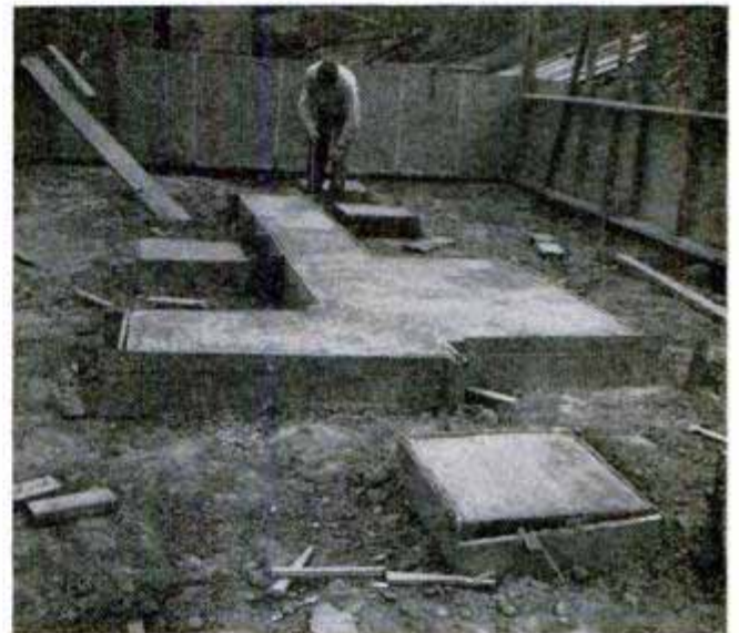
Footings for the beam posts and the "island wall" fireplace, which are 12 in. thick, are poured at the same time as the foundation footings. Below, Norman Chapman, my helper, is spiking the joists
