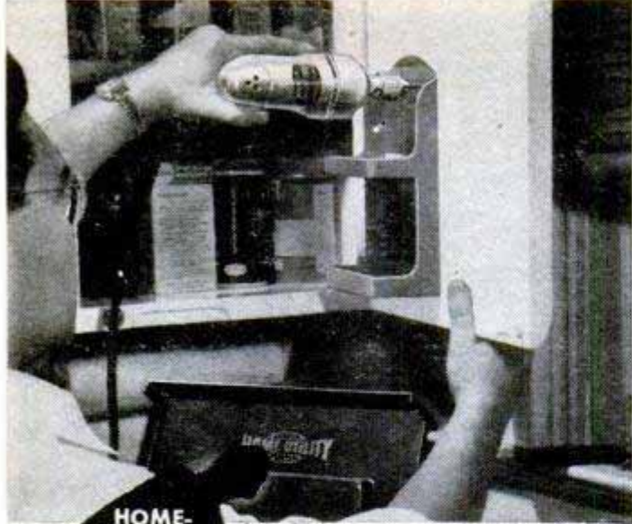
Installing kitchen accessories!
