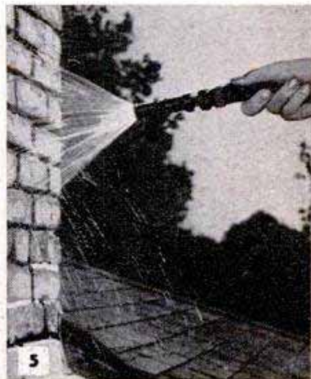
Above, before chimney is tuck pointed, the cap is examined and all cracks are sealed to keep out water. Below, remove all loose and crumbling mortar, brush away the dirt and saturate the brickwork thoroughly
