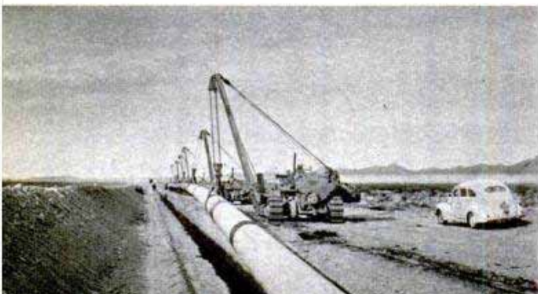
Battery of compressors at pumping station repressures gas to overcome the friction "drag" inside the pipe. Below, side-boom tractors working as a team gently lower welded and wrapped pipe into the deep trench
