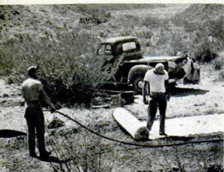
Top of water tank is leveled before sealing and installation of drain. Below, glass mat apron is laid on slope above tank with low dirt border around it. Three inches of rainfall will fill 400-gallon tank
