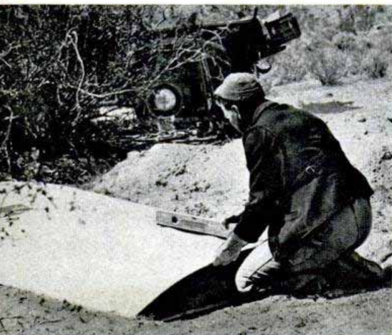
Top of water tank is leveled before sealing and installation of drain. Below, glass mat apron is laid on slope above tank with low dirt border around it. Three inches of rainfall will fill 400-gallon tank
