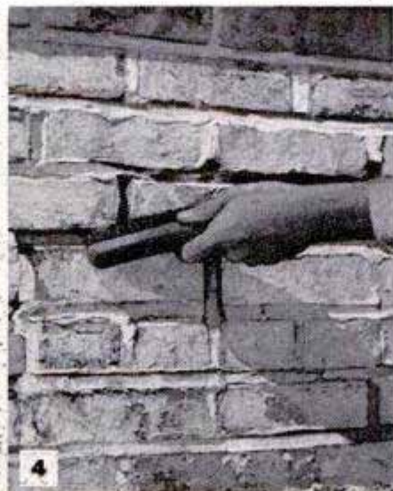
Above, before chimney is tuck pointed, the cap is examined and all cracks are sealed to keep out water. Below, remove all loose and crumbling mortar, brush away the dirt and saturate the brickwork thoroughly
