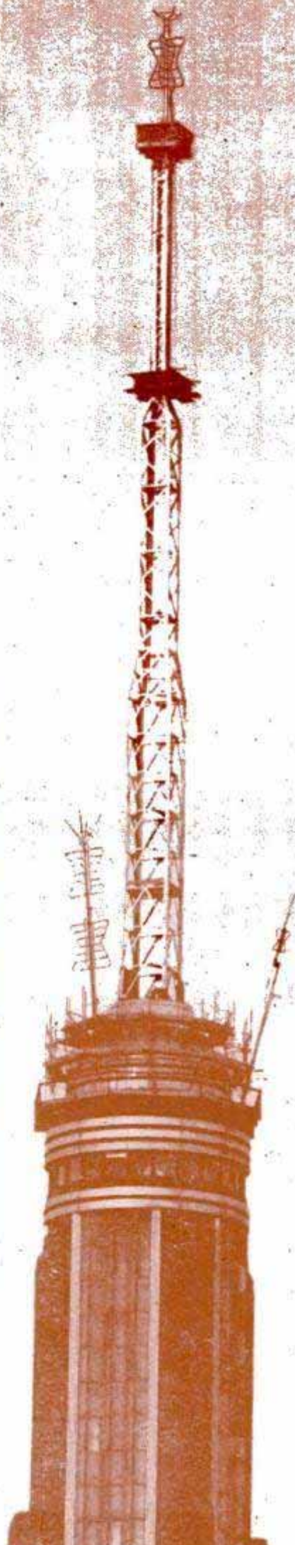
Above, Old Glory flies on man's highest work: Empire State Building mast, 1472 feet high. Over-all view of mast, right, shows the first element for Channel 4 being installed at top
