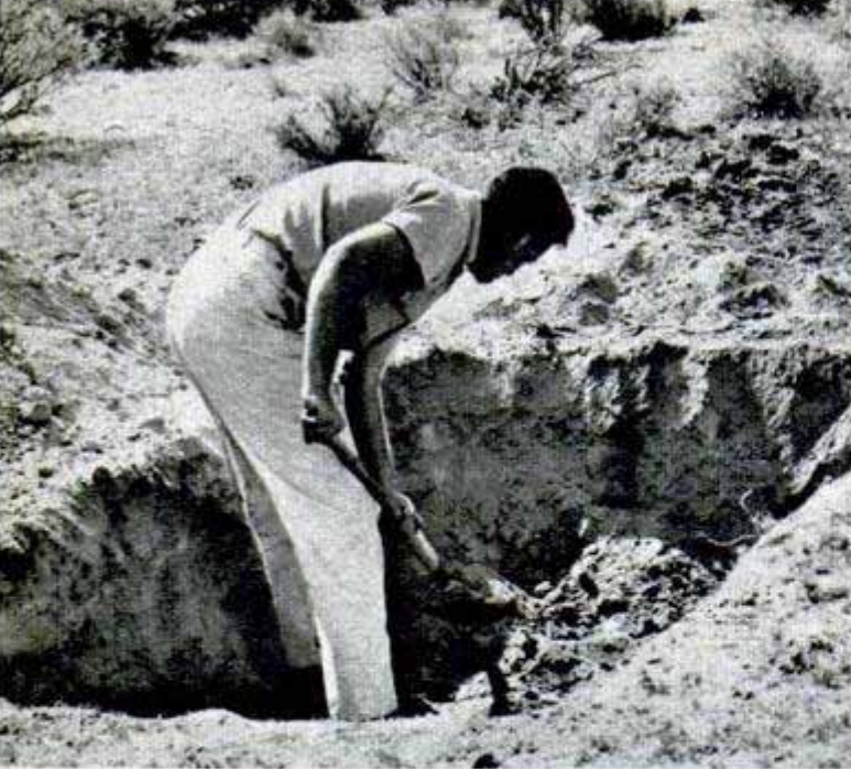
Field worker digs hole for quail "guzzler" tank. An apron for catching rain will be spread on slope above. Protective brush is left around the fountain
