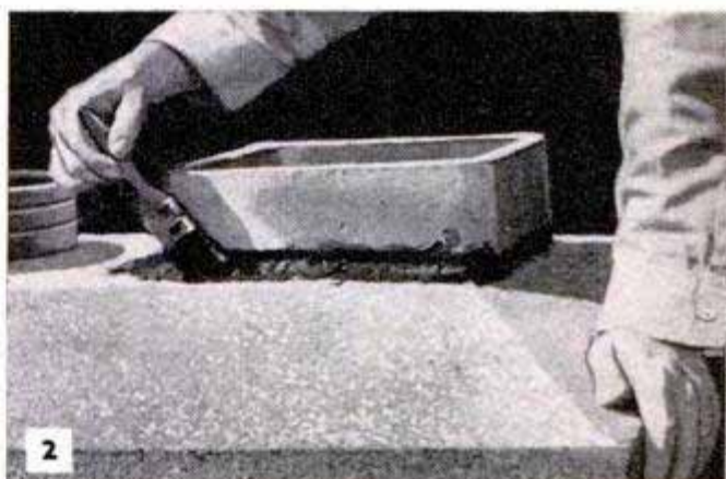
Above, before chimney is tuck pointed, the cap is examined and all cracks are sealed to keep out water. Below, remove all loose and crumbling mortar, brush away the dirt and saturate the brickwork thoroughly
