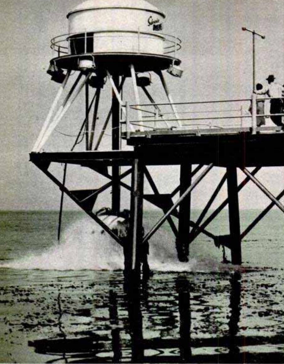
Left, the buoyant bell shoots up from the bottom, breaking through the surface, when the cable is released. Above, ports in the wall provide a view of ocean-bottom scenes
