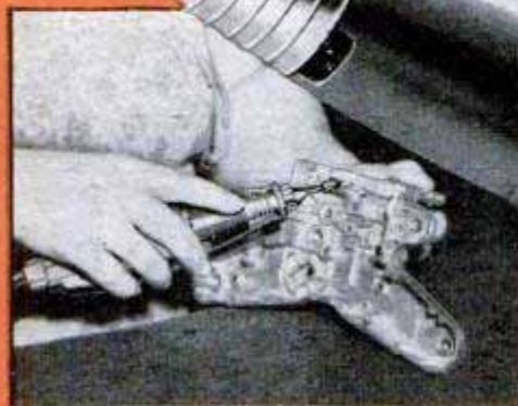
DEBURRING. CRAFTSMAN Rotary Electric Tool, on the "line", deburring castings. It also cleans, wire-brushes, sands.
