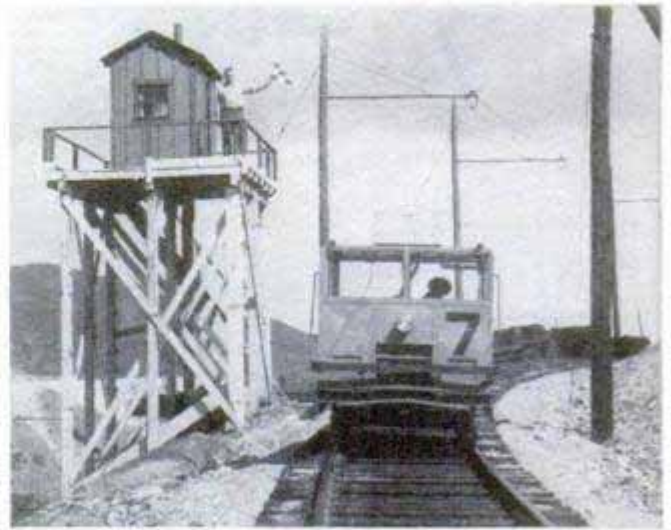
Mine executives ride on a motor-driven rail scooter as they check various workings in the Bingham area
