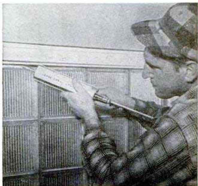
Above, lay the blocks in mortar joints troweled to a uniform thickness of ¼ in. Below, run a line of calking compound all around the completed panel
