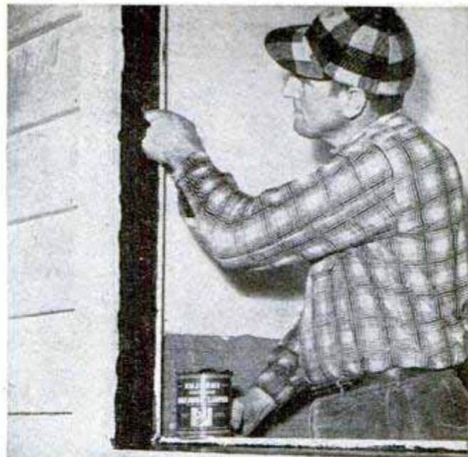
Apply a heavy coating of asphalt emulsion to the sills and jambs. The coating should be at least 3½ in. wide
