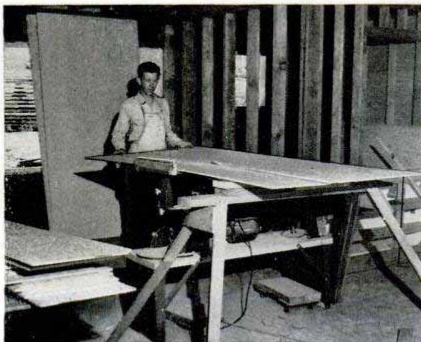
Above, setting end rafters for the two-car garage. To the right of the garage, the enclosed breezeway can be seen. Below, Riley uses a power saw to cut the plywood sheets into lengths of lapped siding
