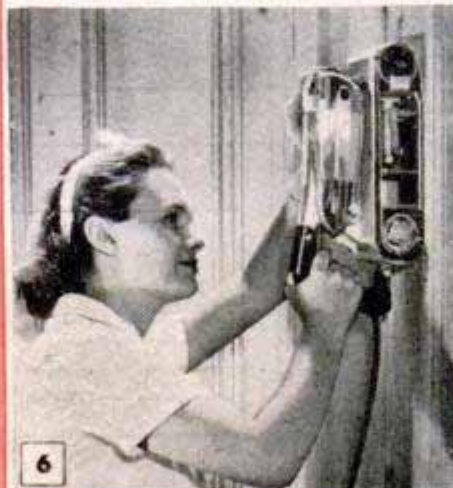
6 9-LB. PORTABLE SANDER IS EASY TO HANDLE ON VERTICAL WORK
