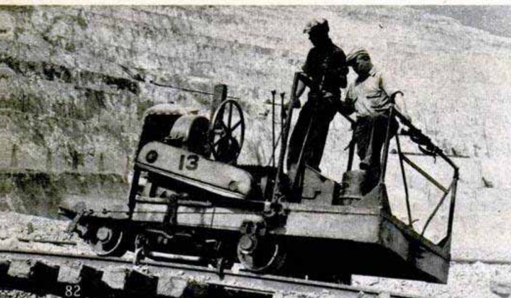
As canyon walls are gnawed away, this machine shifts the rails with them
