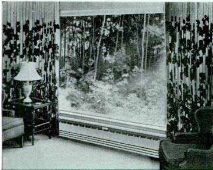
CONVECTOR for the picture-window living room is a long, low model that hides as it heats the room
