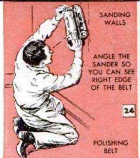
VERTICAL SURFACES ARE SANDED BY STARTING STROKE AT THE TOP
