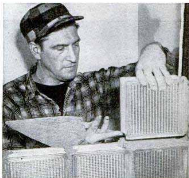
Above, lay the blocks in mortar joints troweled to a uniform thickness of ¼ in. Below, run a line of calking compound all around the completed panel
