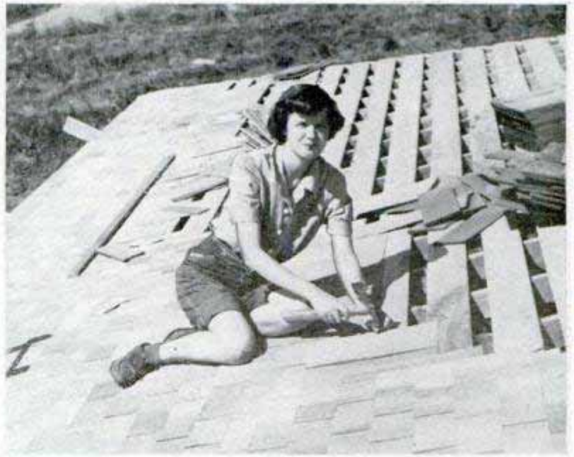
Vinita Riley helps with shingling—a big job on the long house
