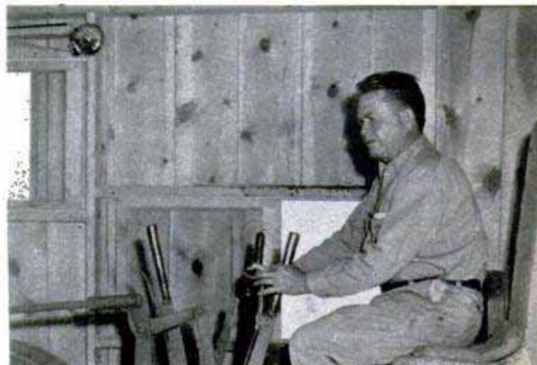
Hoist man operates levers to control the engine. He's connected by telephone with the engineers far below
