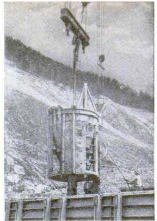
Left, fly ash is also used to make concrete pipes on this machine. Right, dumping concrete at Hungry Horse
