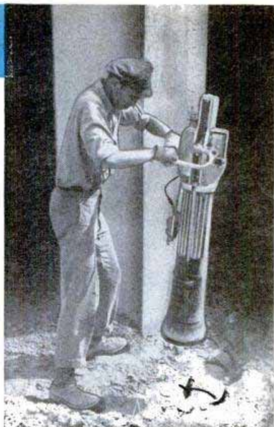
SELF-CONTAINED TAMPER for earth and gravel fills is pictured above in operation. It is actuated by a piston sliding in a cylinder in which a fuel mixture is fired by magneto ignition. Thrust from piston can be adjusted to lift tamper from 12 to 20 in. It falls by its own weight. The tamper is operated by one man and will compact from 10 to 20 cubic yards of earth per hour on a quart of fuel, a gasoline-oil mixture similar to that used in two-cycle engines
