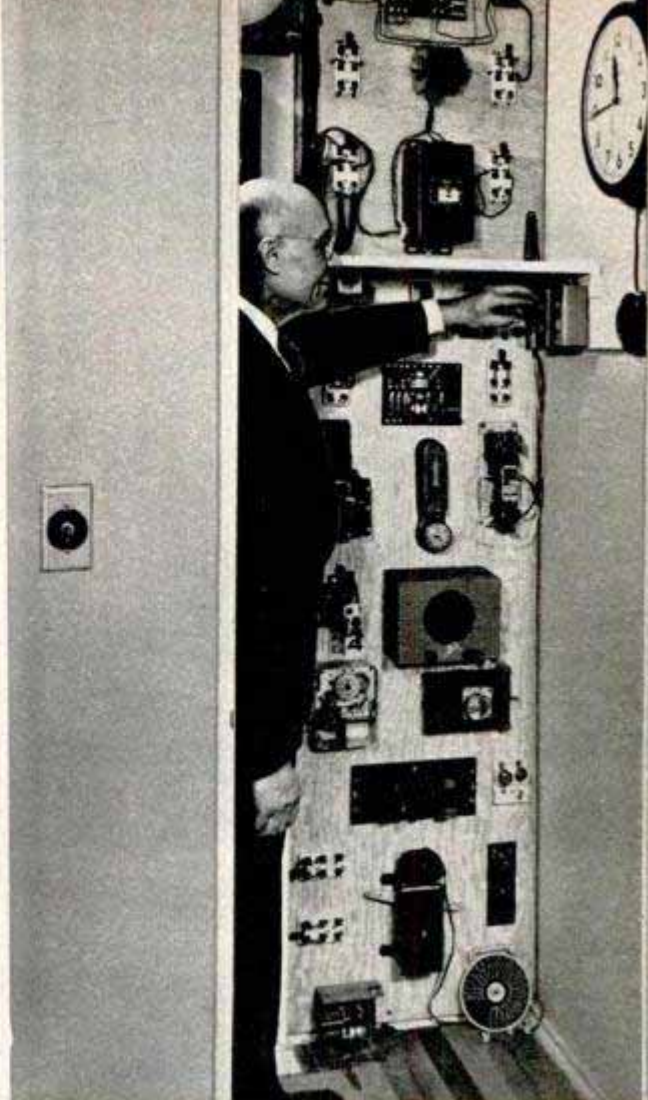
Once an ordinary closet, the master-control room is lined with many switches, timers and relays
