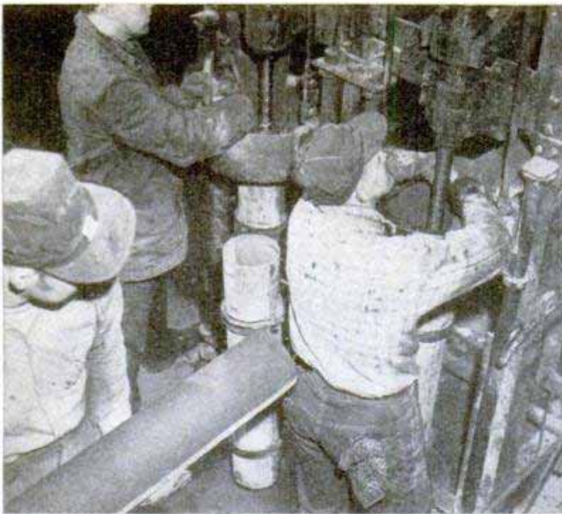
Left, fly ash is also used to make concrete pipes on this machine. Right, dumping concrete at Hungry Horse
