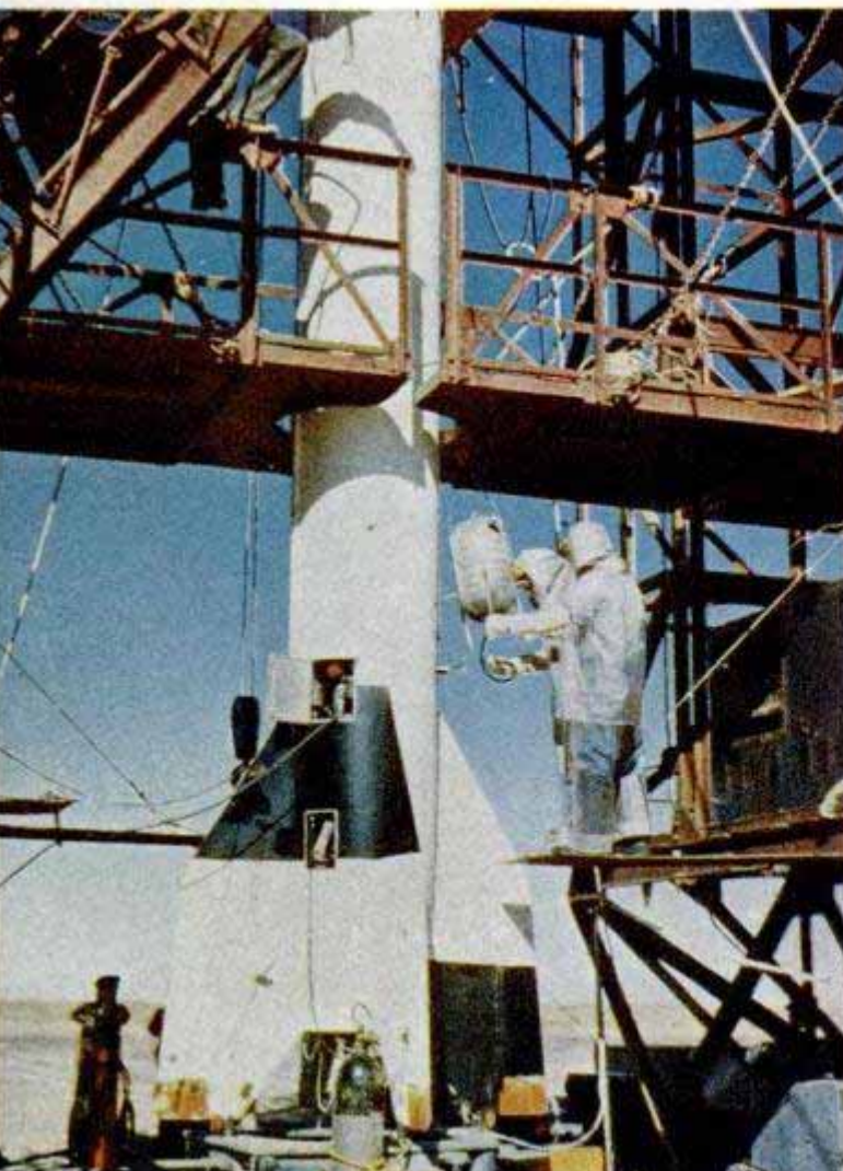
Elaborate tubular scaffold holds the Lark as it is prepared for firing. Below, fuel experts load a big rocket with hydrogen peroxide. Chemical, which will explode if touched, rolls off plastic suits
