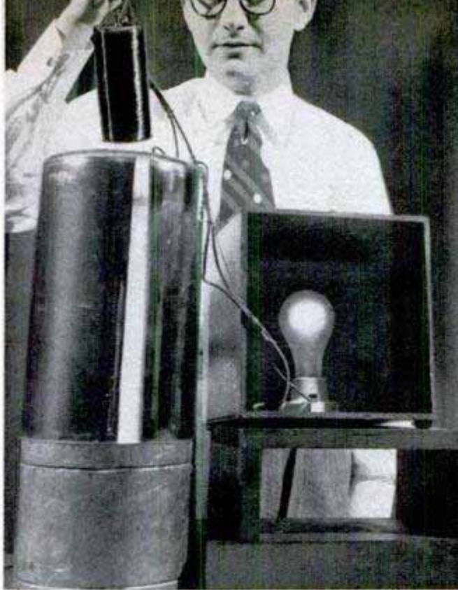
Experiment shows how supercold reduces electrical resistance. Bulb burns dimly, left, but when copper coil, carrying current to bulb, is dropped in some liquid nitrogen, right, the light output increases many times
