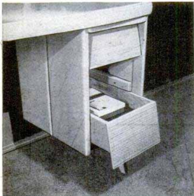
Drawer fronts of striated plywood are inclined at an angle of 10 deg., making rails unnecessary
