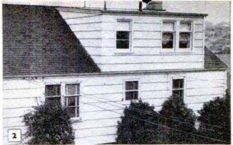
Here's how the finished dormer looks from the outside. Adding a dormer greatly increases the usable area of attic rooms under a low-pitched roof. Double windows admit light and air
