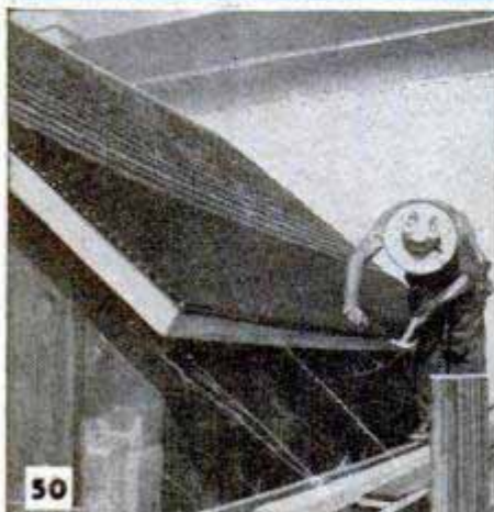
Edges of the roll roofing can be folded over and nailed as in Fig. 50. Measure and snap a chalk line to show the amount of lap as in Fig. 51. Finish the ridge as in Fig. 52, using a 10 or 12-in. strip of roll roofing
