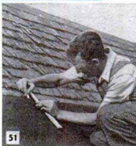
Edges of the roll roofing can be folded over and nailed as in Fig. 50. Measure and snap a chalk line to show the amount of lap as in Fig. 51. Finish the ridge as in Fig. 52, using a 10 or 12-in. strip of roll roofing
