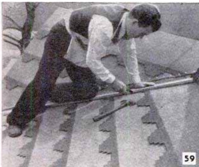
Pattern-edge roll roofing is available in a variety of patterns and makes an attractive, inexpensive roof
