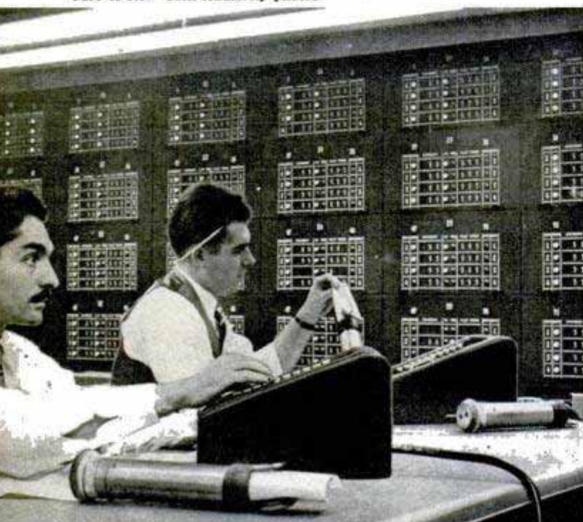
In platform control section, operators trace movement of every box in the building by watching numbers flash on panels. Below right, cylinders which hold shipping papers drop out of pneumatic tubes onto a moving belt
