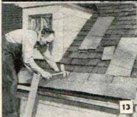
Lay a row of inverted shingles at eaves to form the starter course
