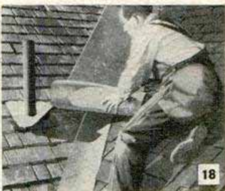
Two layers of roll roofing used in valley, same color as shingles
