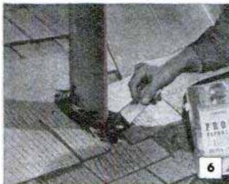
6 ROOF CEMENT IS VERY ESSENTIAL FOR TIGHT FLASHINGS AND VALLEYS
