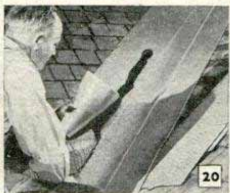
Shingle ends at valley are bedded in roofing cement to turn water
