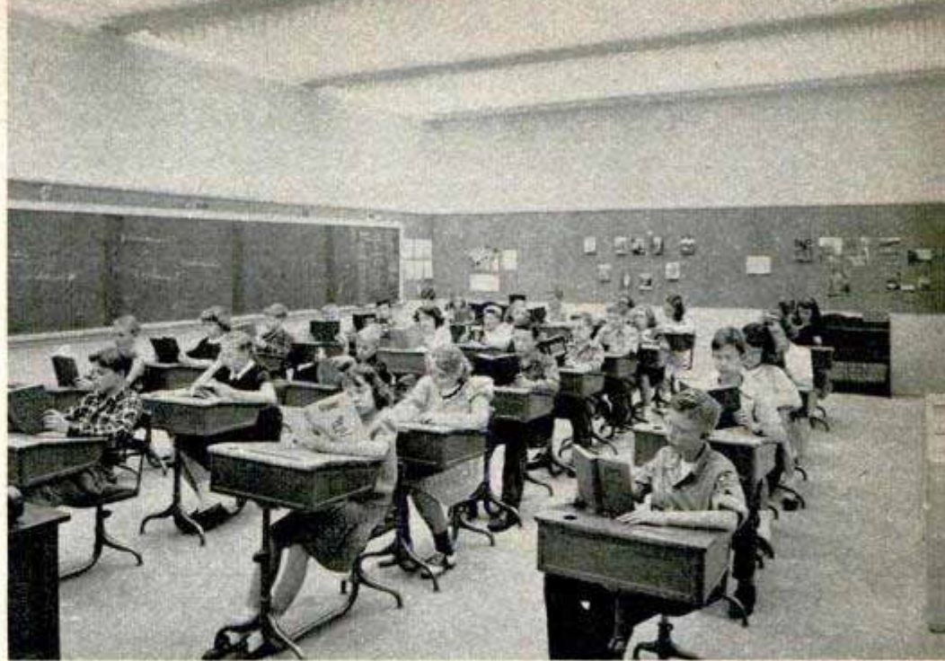
General Electric photo "Ceiling of light" sheds an even, almost natural light over the entire classroom, yet none of the fluorescent tubes can be seen. "Egg carton" panels made of metal do the trick. Below, modern high schools have several up-to-date kitchens where future homemakers learn to prepare meals St. Charles Manufacturing Co. photo
