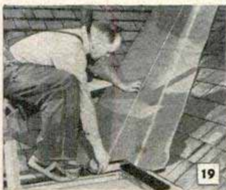
Chalk lines are snapped on valley to indicate trim line for shingles
