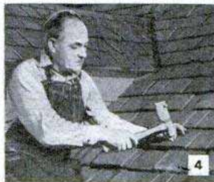
4 GOOD BASE IS ESSENTIAL. SPLIT AND NAIL DOWN WARPED SHINGLES
