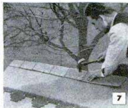
7 RIDGES CAN BE FINISHED WITH CUT SHINGLES OR ROLL ROOFING
