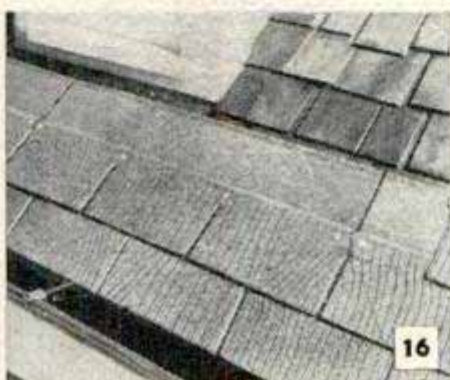
Four nails fasten each shingle. Nail straight to avoid cutting
