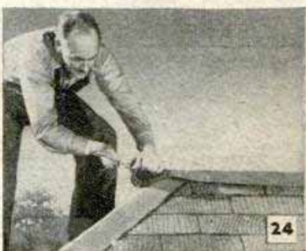
Ridges and hips can be finished with 12-in. strips of roll roofing
