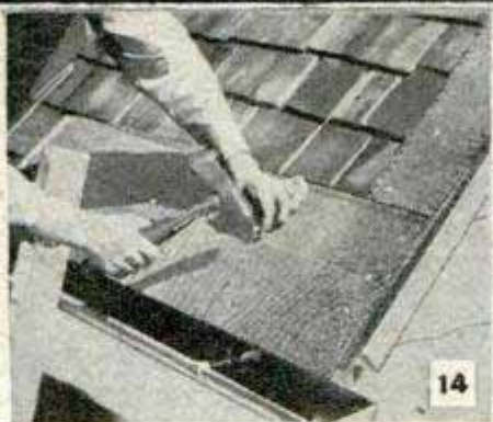
First course starts with full shingle with the edge flush at eaves
