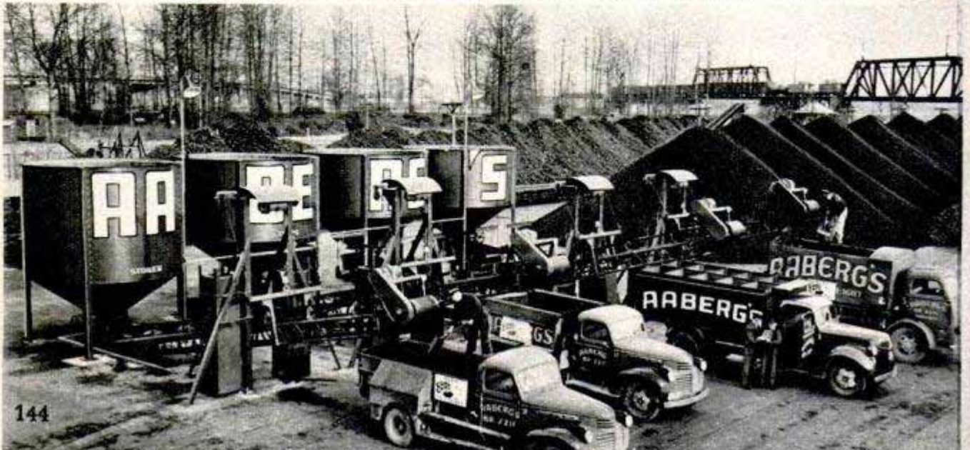
Below, empty trucks rumble up to the four bins, buttons are pushed in the office and the selected types of coal pour into the trucks. No one touches the coal after it leaves rail car
