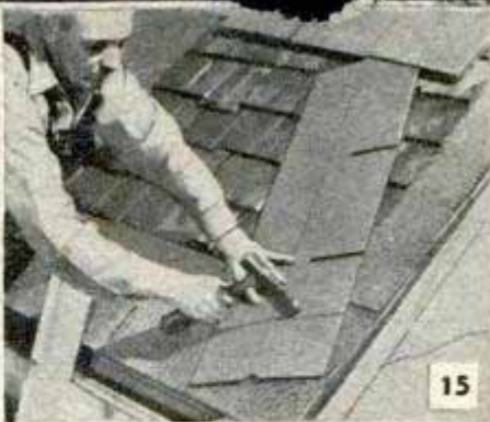
Begin second course with full shingle less 6 in. Cut shingle from back
