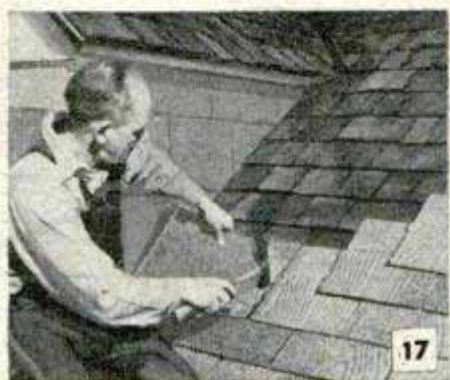
Shingles are cut and flashed to all parts projecting above roof
