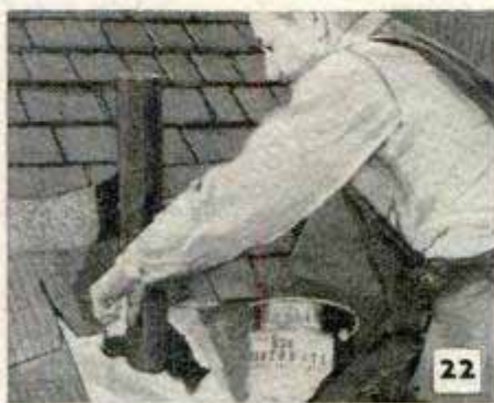
Plastic roof cement assures tight joints at vent pipes and chimney
