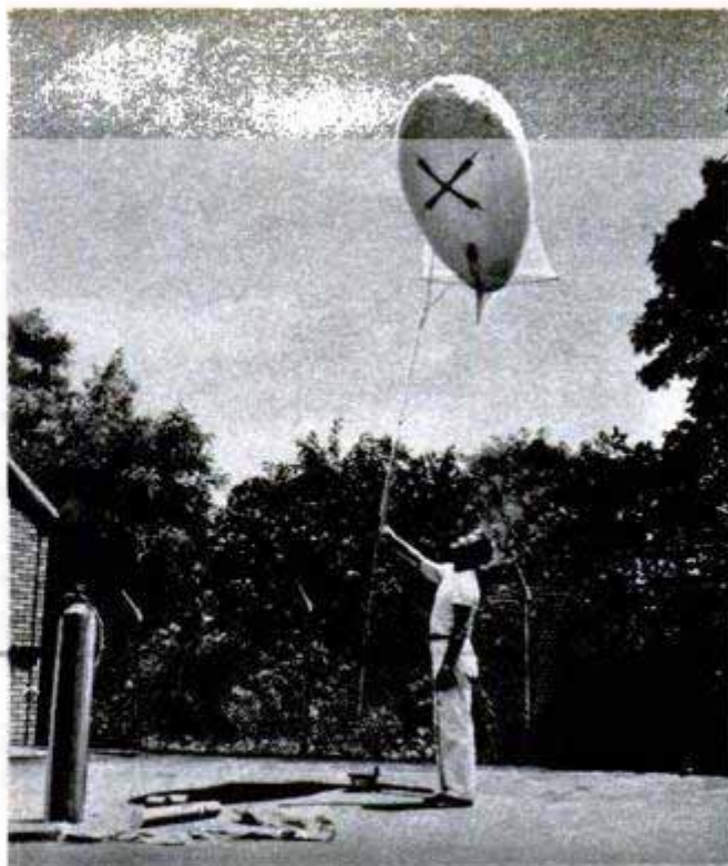
Live in a TV fringe area? A Kytoon will raise your antenna (the cross on underside) for good reception
