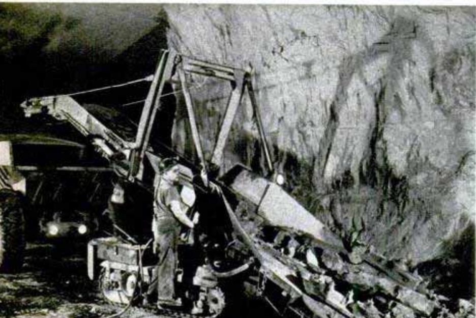
To the cable on this hoist are attached the two skip buckets that each carry up 10 tons of rock at a time to the surface. Below, the two mechanical arms on this Joy loader gather rock and place it on a moving belt that takes it to dump trucks
