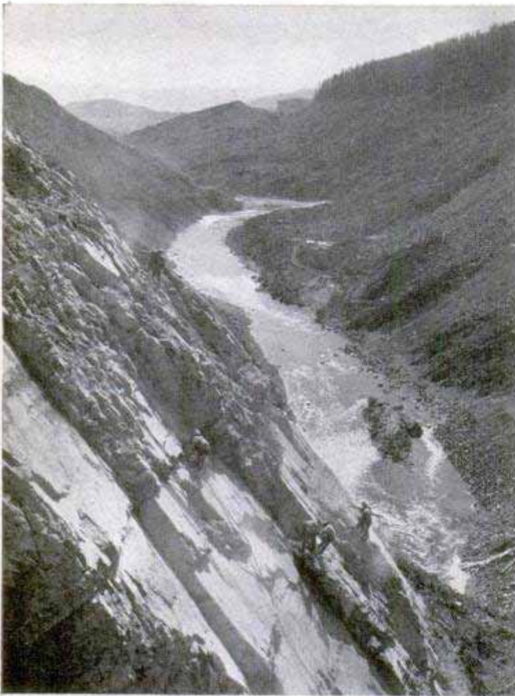
Drillers wearing life lines knock down broken bits of surface rock on wall of canyon to which one side of dam will be anchored. Below, general view of the site shows the river, earth cofferdam and beginning of concrete foundation
