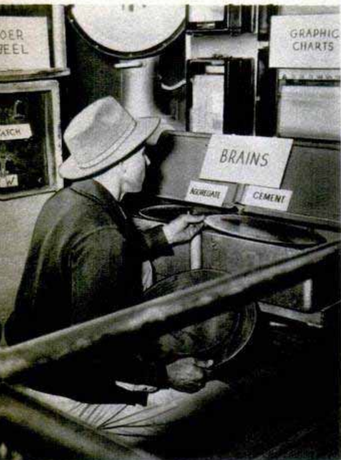
Operator selects a disk to match the kind of concrete ordered and places it on a turntable. Disk makes electrical contacts to release material and water into mixers in the proper ratio. Above, right, diagram shows the multilevel mixing tower
