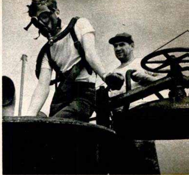
In emergency, when there's no time to clear tanks of gas, crewmen wear fresh-air masks for repair work
