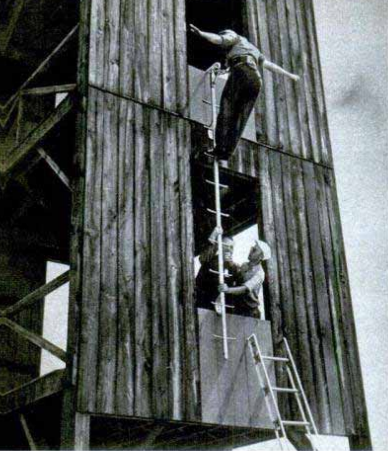
It takes courage to go up the outside of a building on a slender scaling ladder and volunteers have it
