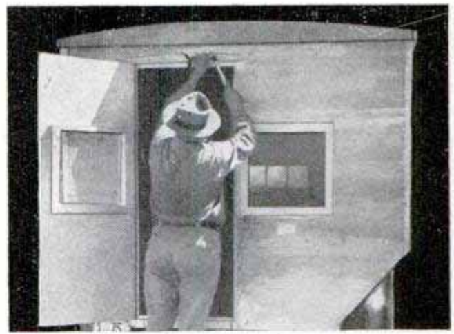
Above, top edges of the door and window lintels are beveled to form drip caps. Below, prime-coat the roof, sides and ends with one coat of aluminum paint
