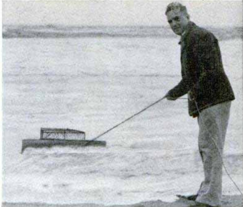
Smallest wave sled can carry several baited hooks 800 yards offshore. Right, sled drags lobster trap to sea
