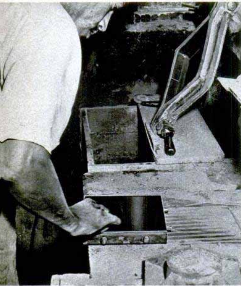
To prevent the tiles from sticking, the steel faceplate for the form is carefully polished and oiled
