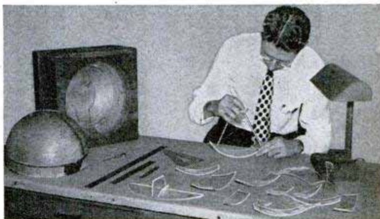
Workmen assemble pieces of the sphere and tack-weld them in position. Patterns for the sections of the tank, called an icosasphere, were cut from a model made of plastic with a "memory" shown in the photograph below
