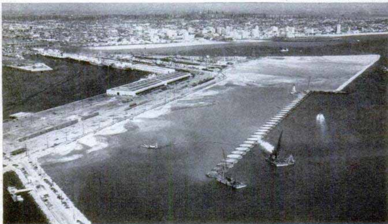
Lined up like plates on a banquet table, these sea-wall barrels will hold in 136 acres of fill
