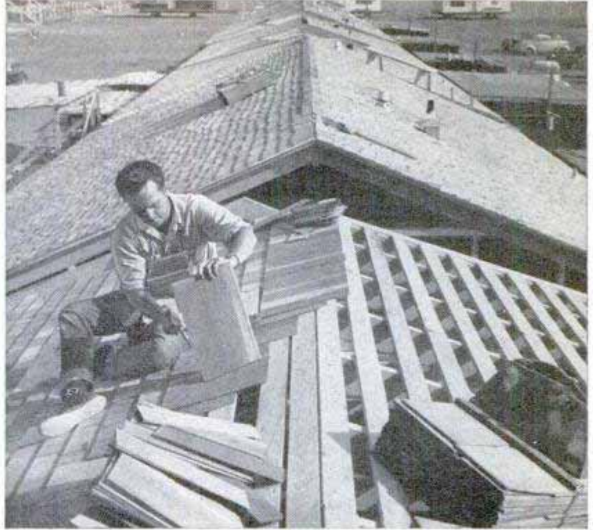
Wooden shingles are nailed in place by an experienced workman, who does the same job on every house as it rolls down the line. Below, metal straps, installed diagonally, keep the interior walls rigid
