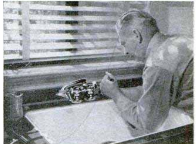
2 First step is to unscrew cap nut from faucet
