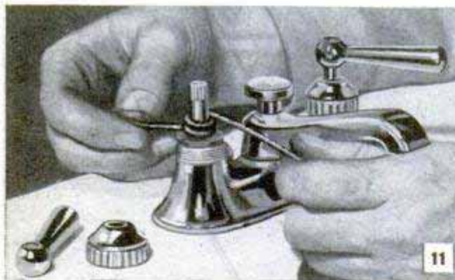
Leaks due to worn or frayed packing can be easily stopped with a packing washer or with a graphite-asbestos wicking especially made for this purpose
