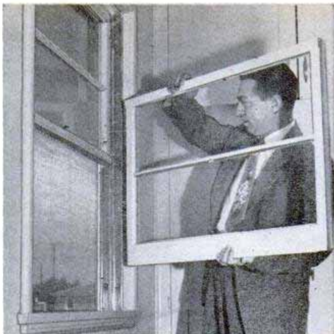
Among the new fixtures built into the homes are windows that can be removed from frames for cleaning
