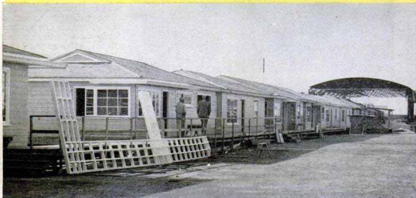
Resting on rollers, 13 homes move toward completion at once. Above, two of five plans offered in San Diego
