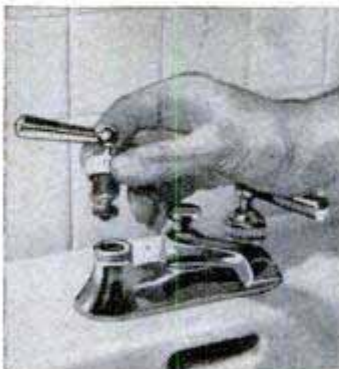
4 Lift out the spindle
