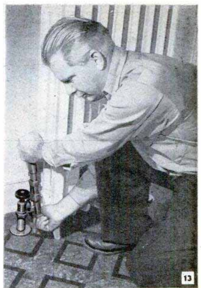
Two types of shutoff valves that are commonly used in water lines to shut off the supply to fixtures. The main shutoff valve usually is placed near meter
