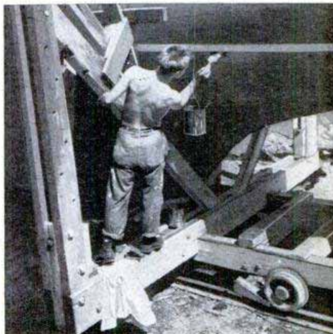
It's regular practice to apply a nonfouling copper bottom paint, especially if boat is used in salt water
