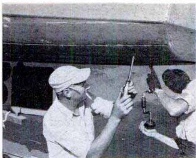
Where large screws must be used, set them with a hand screwdriver, then drive home with brace driver
