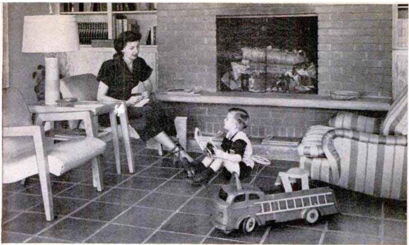
Above, the entire floor is a radiator when hollow tiles are used as radiant-heating panels. Below, diagram of a complete system. Arrows show the flow of warm air through the tiles
