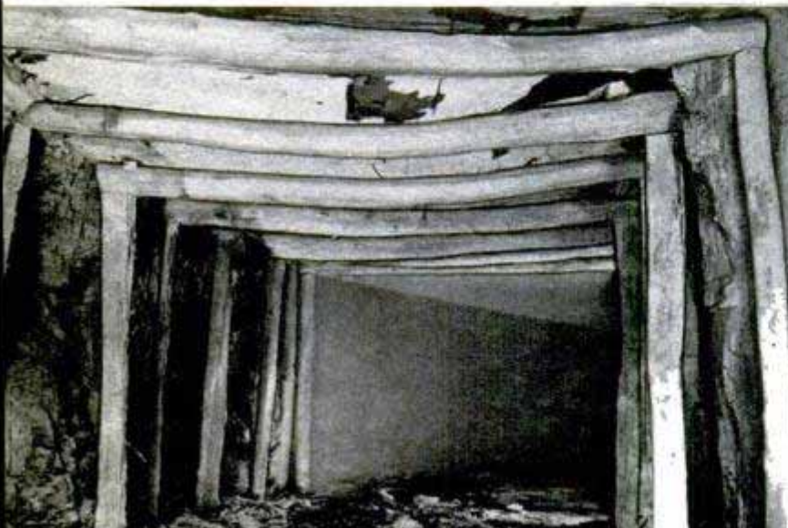
Above, two pin-up methods, showing expansion wedges. Below, foreground, the old system; beyond, pin-ups hold roof
