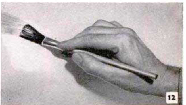
Above, sand off paint blisters and feather the edges. Below, seal the exposed plaster with sealer or paint
