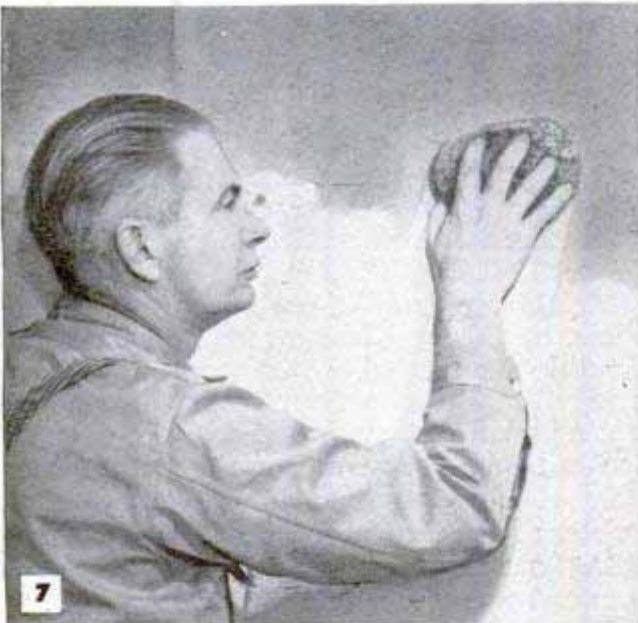
A thorough washing with cleaning solution assures surfaces that are entirely free from dirt and grease
