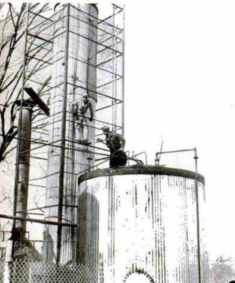
Below, the acid tank at the Worthington plant. Oil is mixed with acid to settle out sludge shown above
