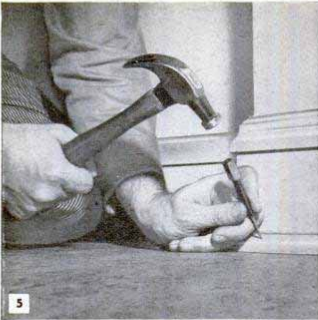
Reposition the base shoe molds at the floor level if there are wide gaps as shown in details at right
