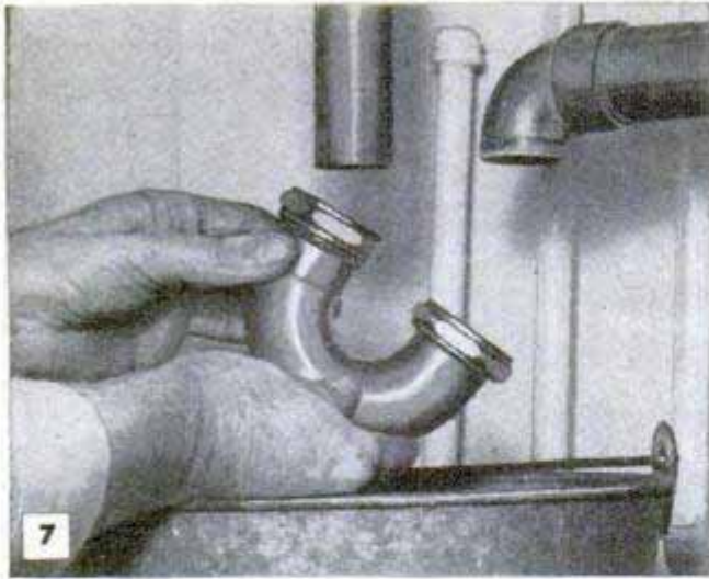
7 Removing the sink trap and pipe elbow makes it considerably easier to run a drain auger through pipe
