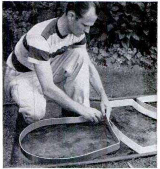
2nd. The sheet-metal bands which form the molds are made "endless" and then bent into irregular shapes, no two being alike. The ends of the bands are wired together and molds are placed as desired 2 in. apart
