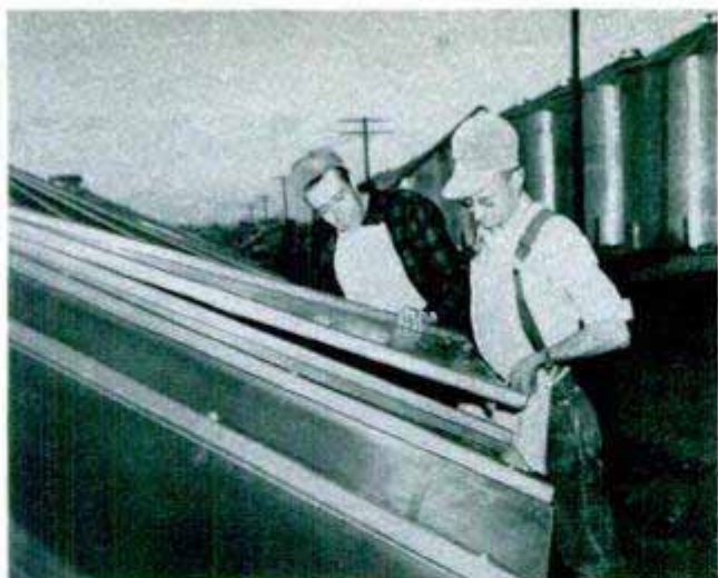
Workmen in photo at left install roof of grain bin while in picture at right conveyors fill bins as soon as they are finished. Below, roof of bin is built first and tiers are added below it to form structure
