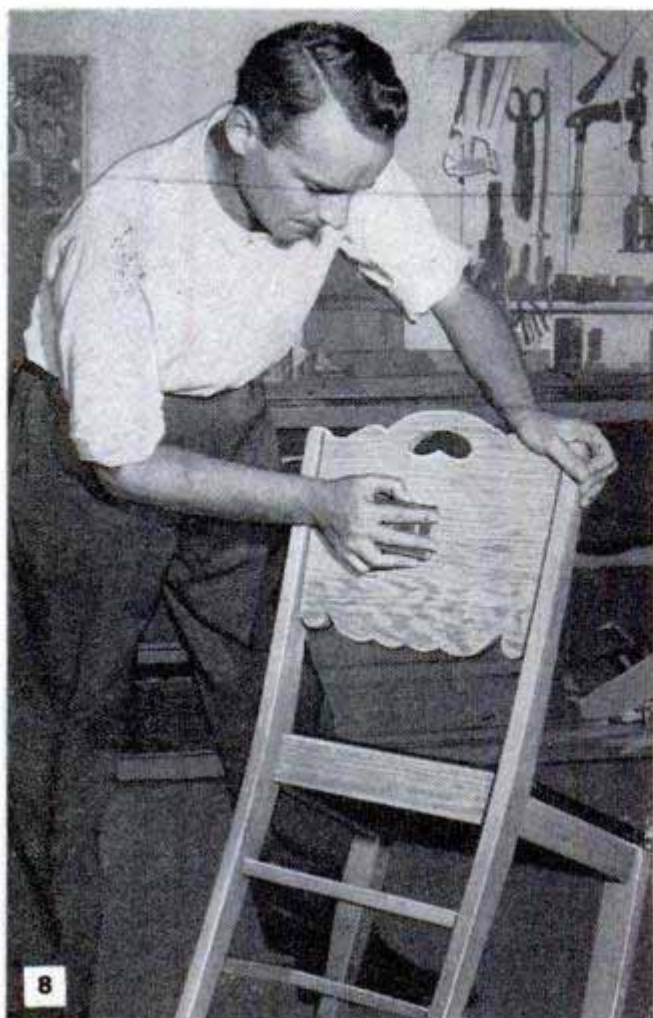
Above, abrasives rather than scrapers are now commonly used in preparing old work for refinishing. Below, on some types of work a felt backing is used
