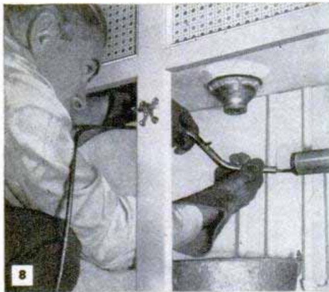
8 Push the auger into the pipe and turn the crank. The crank is moved back as the auger is advanced
