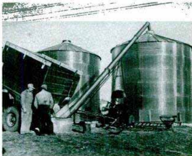
Workmen in photo at left install roof of grain bin while in picture at right conveyors fill bins as soon as they are finished. Below, roof of bin is built first and tiers are added below it to form structure
