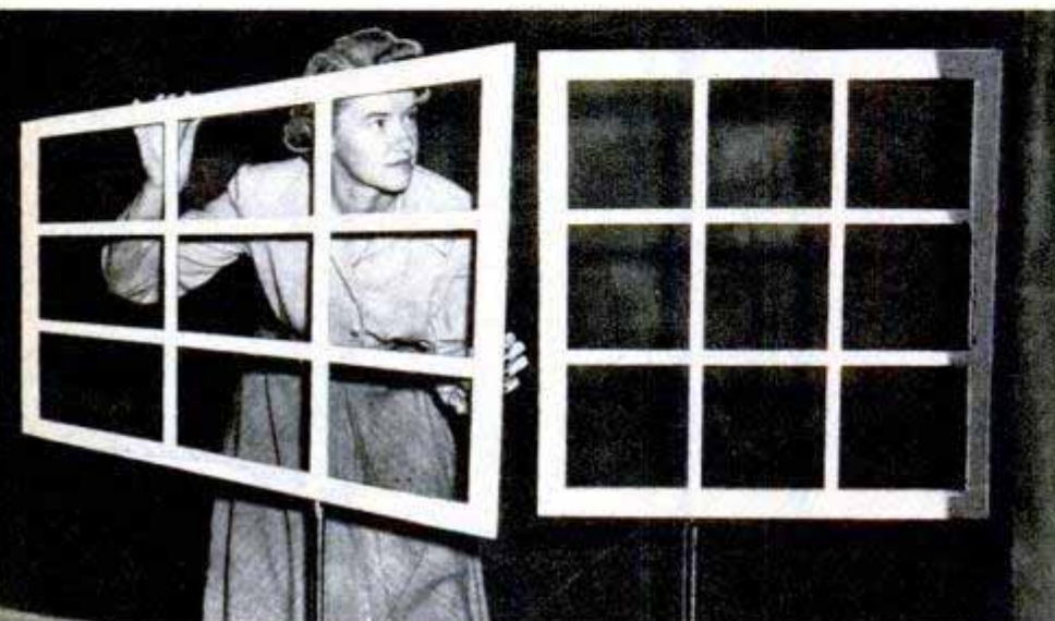
Window at right is square and stationary; window at the left, shaped like a trapezoid, is mounted on a vertical rod and is moved with strings operated by the victim. Problem is to make edges parallel
