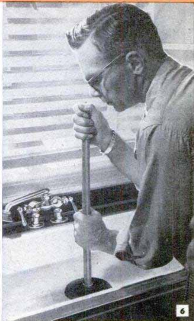
The alternate pressure and suction of a rubber plunger frequently will open a completely clogged drain
