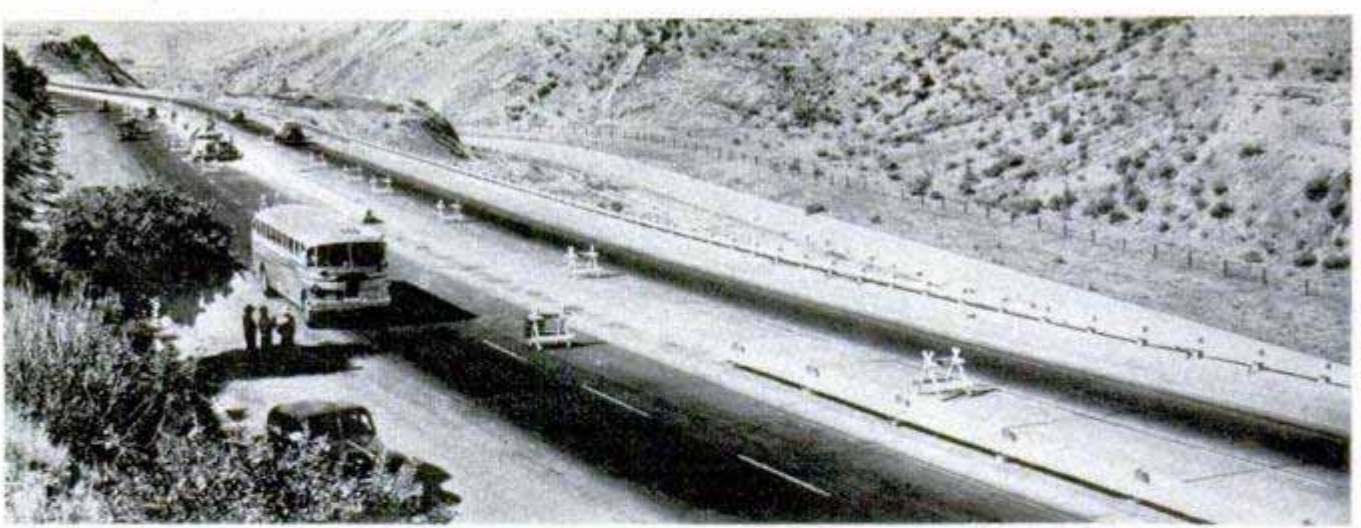
Above, concrete divider in background is replacing wood-steel type on California roads. Right, close-up of the new divider
