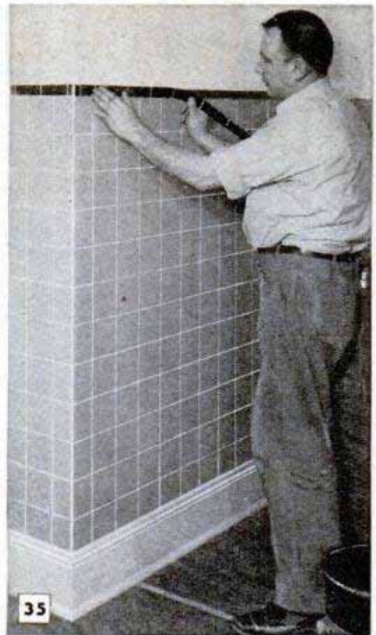
Top of linoleum is finished with cap mold
