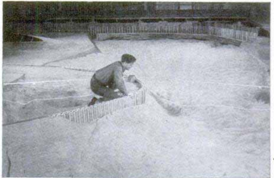
Drawing shows huge dam to be built in India. Below, river model shows points where erosion can be expected
