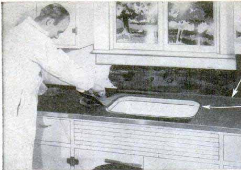
DAMPPROOF CEMENT IS USED FOR BOTH LINING AND LINOLEUM
