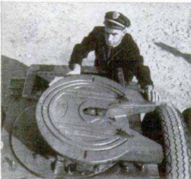
To prevent the tilt, shown at top of page, this new fifth wheel turns with the trailer. Below, the same truck in the same maneuver, but this time there is no tilt because the tractor has the new fifth wheel
