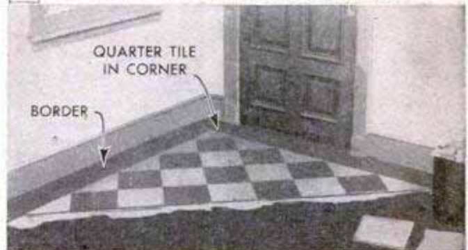
29 DIAGONAL CHECKERBOARD STARTS WITH QUARTER TILE
