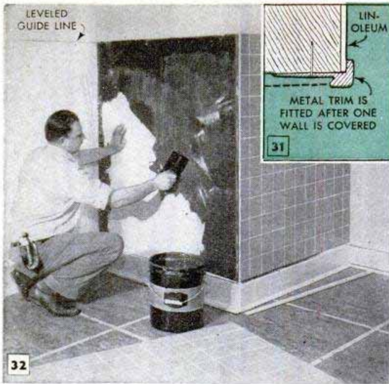
Standard wall linoleum comes 4 ft. 6 in. wide and is cemented directly to the wall, keeping it running level with a guide line marked on the wall. Detail shows how corner molding fits
