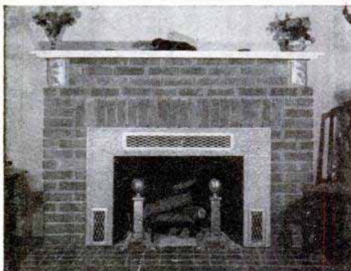
Left, heat circulator in fireplace opening and, right, partially inserted, showing smoke and gas outlets
