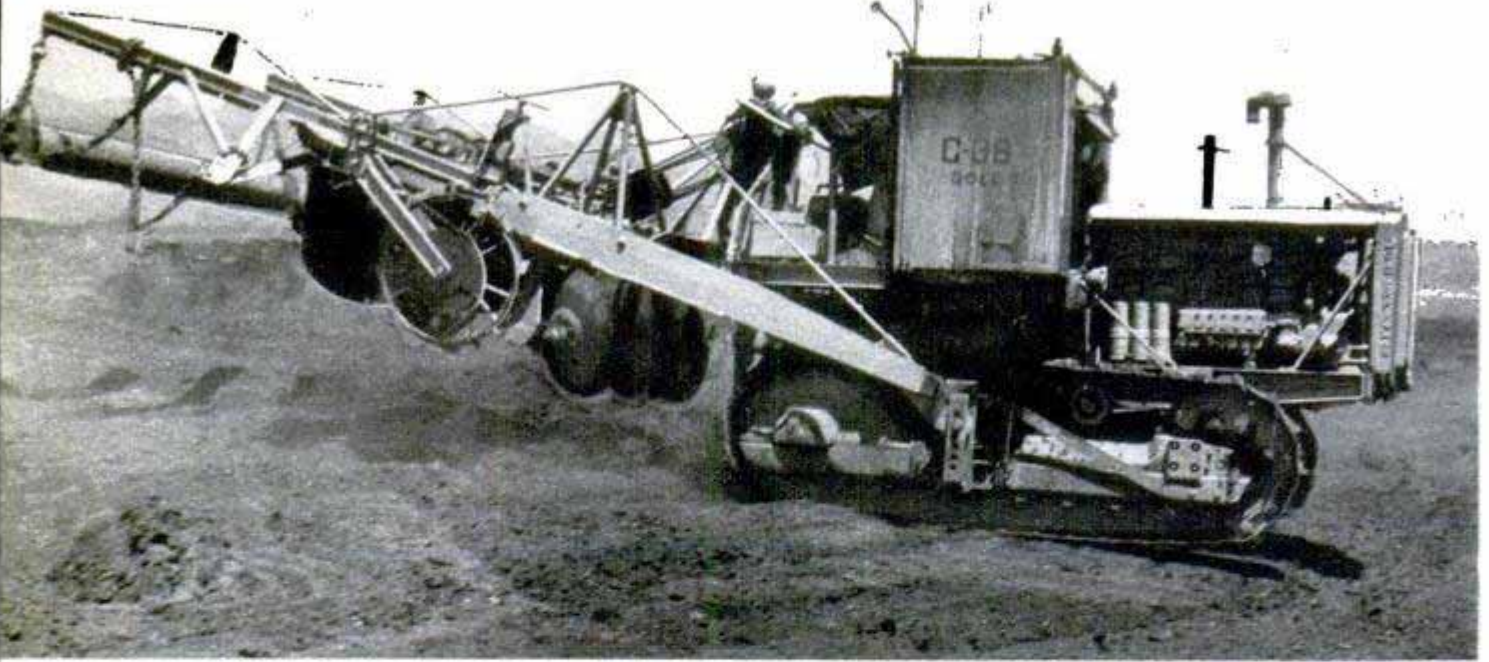
Disks on subsoiling tractor break up the ground to depth of 20 inches; roller on end of boom smooths earth
