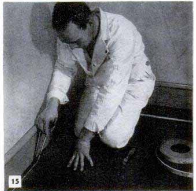
Place the border against field and scribe to wall, making sure strip does not buckle while being scribed
