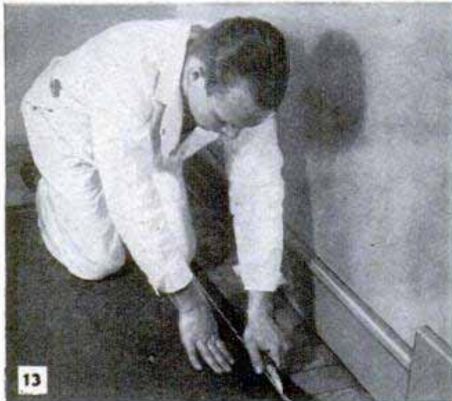
Above, a straightedge is used to trim field linoleum. Below, scribe is set to exact width of feature strip
