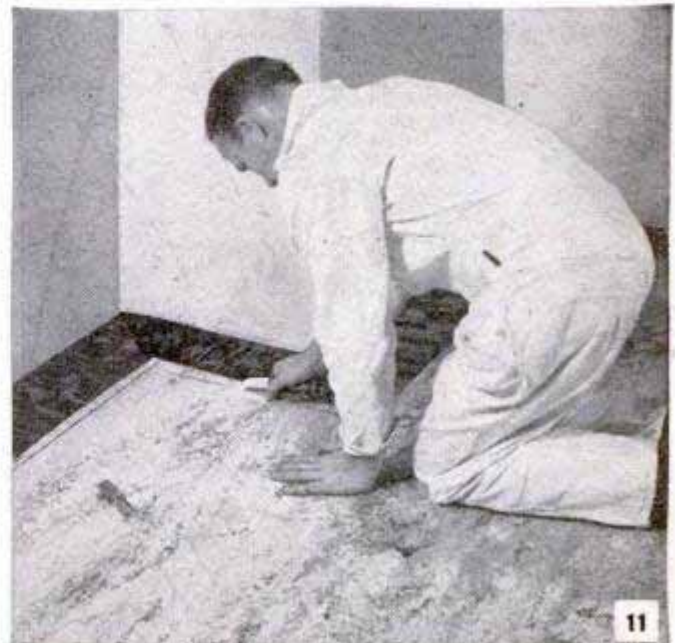
Above, border is scribed to fit contour of the wall. Below, joint is double-cut to produce a perfect fit
