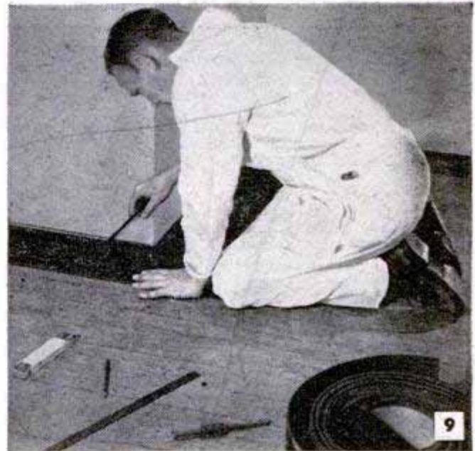
Above, border is scribed to fit contour of the wall. Below, joint is double-cut to produce a perfect fit
