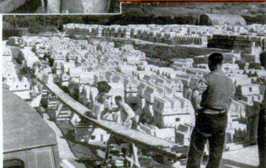
Above, after cement is mixed with clay waste it is deposited in steel molds and pressed into shape. The complete blocks are lifted from the molds by suction
