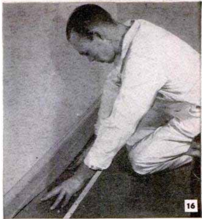
If essential measurements have been properly made, border and feature strip will fit opening accurately
