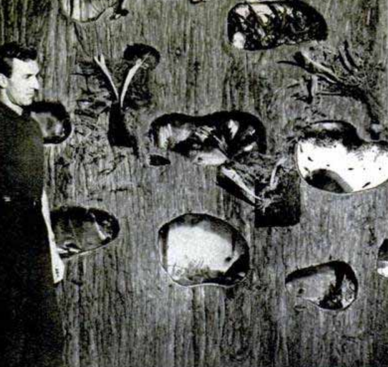
Bark partition above, left, hides wiring and plumbing of fish tanks and swings aside for access to tanks, right
