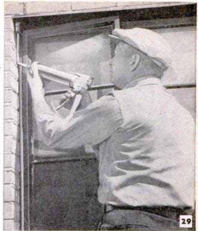
Outside joints between window frames and walls are calked to prevent leakage of air and moisture. Calking should be checked annually for tightness
