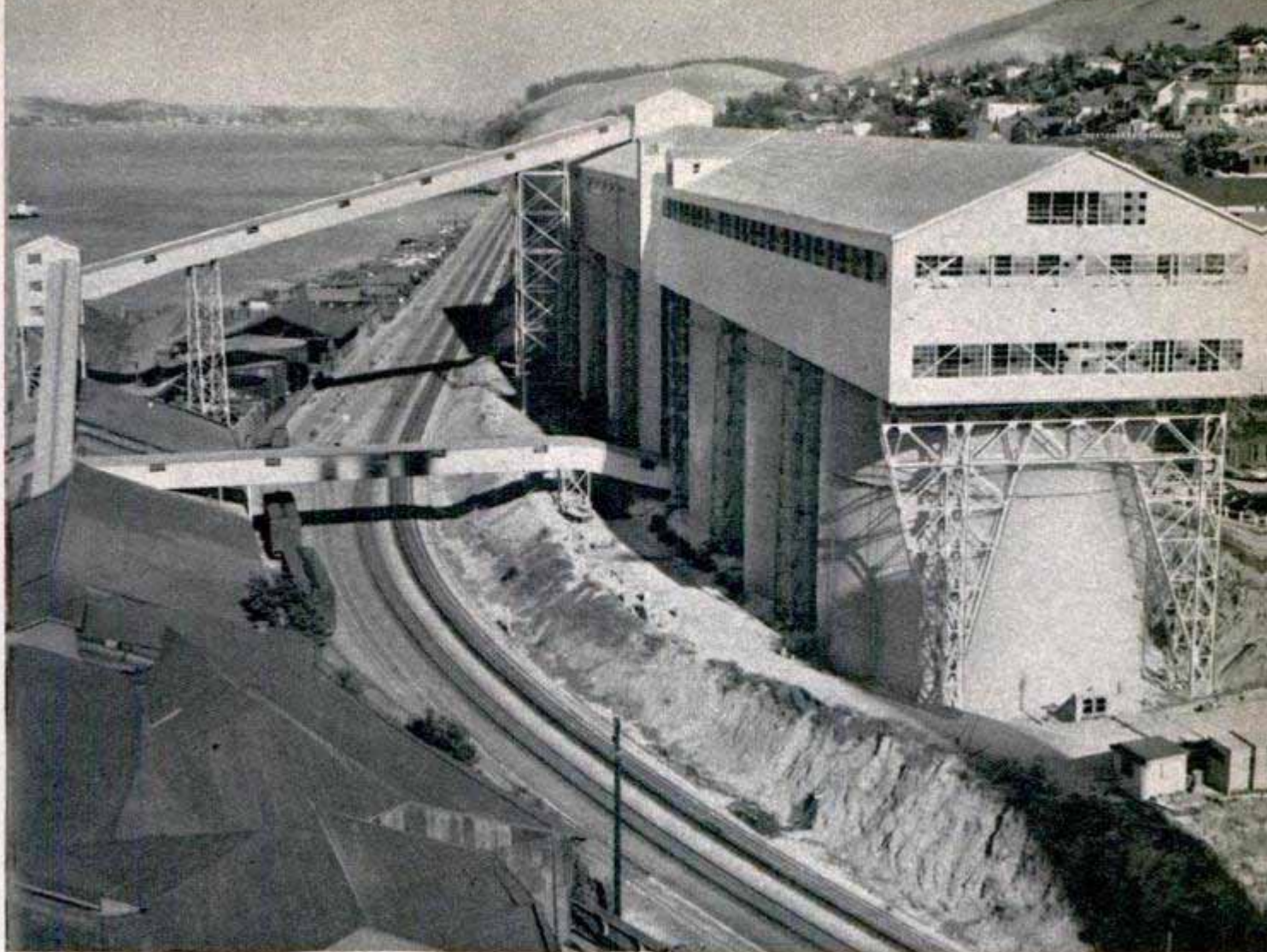
These are the storage silos at Crockett, Calif. Note the ramps inside which conveyor belts move the sugar
