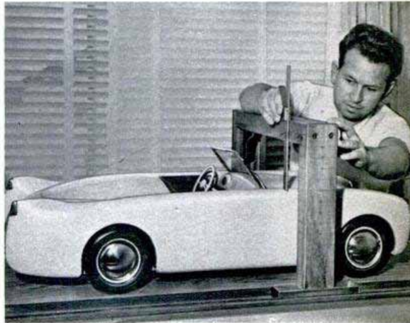
Quarter-scale model of the Edwards car provides full-scale body measurements for the engineers. This model shows top removed and rear seats concealed for use as a sporty low-slung roadster
