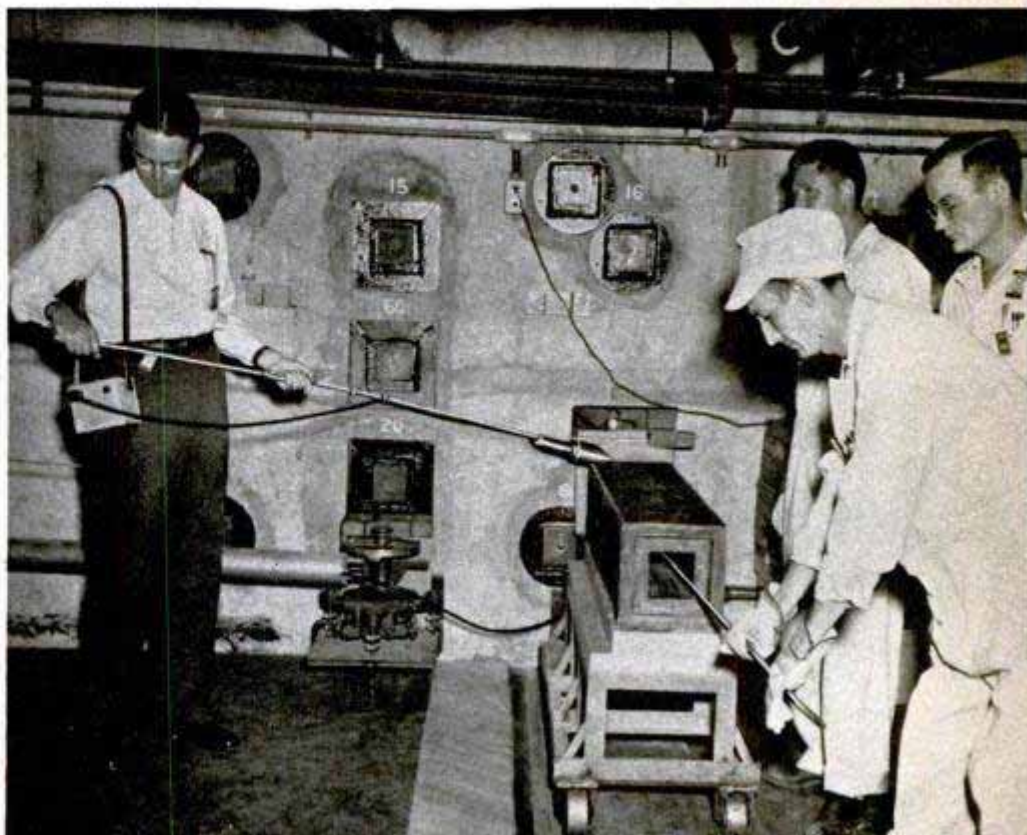
Above, a health sleuth collects an air sample alongside a swing-frame grinder. Caught in a vial of alcohol, the dust in the air is measured on the microprojector. Below, a counter measures atomic radiations of an isotope stringer that is being withdrawn from the pile at Oak Ridge
