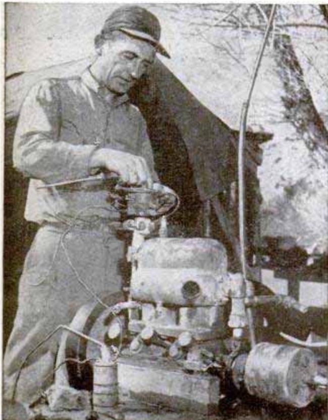
Below, Art installs distributor from their old car on the motor of milling machinery they improvised
