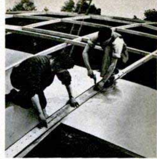
Left, ends of the framework members fit into sockets in the special shoes. Center, the shoes are welded to an outer support ring. Right, after the framework has been built, aluminum sheet is welded to cover it
