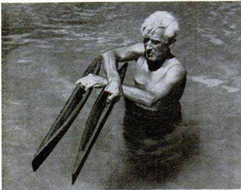
Here Wood has split the boat hull lengthwise and reversed the two halves, placing the curves on the inside. Outside curves cause yawing. Below, he has bridged the split hulls to make them stand up
