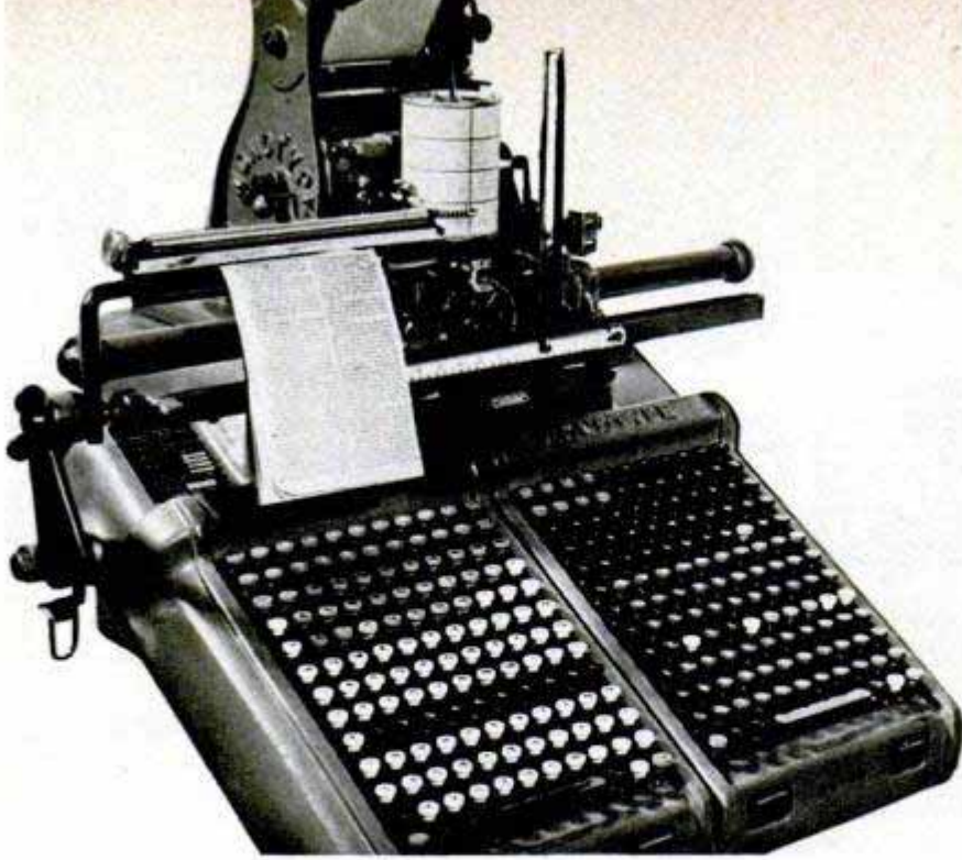
Rotofoto typesetting system starts by making a punched-paper record of the text (right) on keyboard machine
