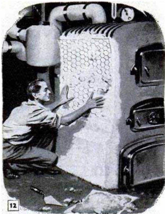
12 Older-type boilers should be covered with a 1-in. layer of asbestos cement which will reduce loss of heat
