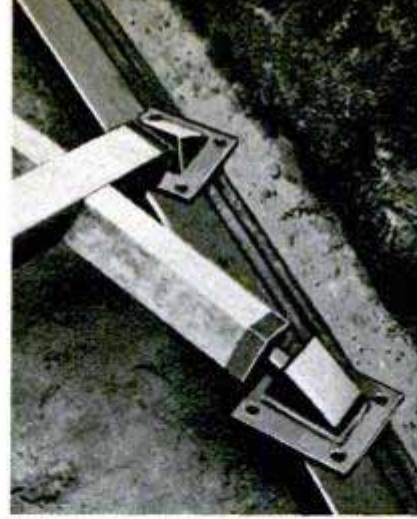
Left, ends of the framework members fit into sockets in the special shoes. Center, the shoes are welded to an outer support ring. Right, after the framework has been built, aluminum sheet is welded to cover it
