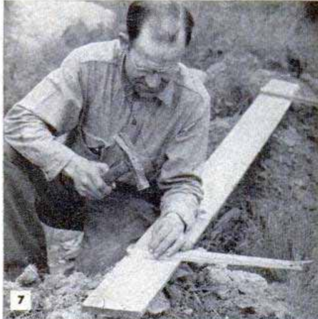
A long guide board fitted with sharpened stakes is an aid in digging a straight trench to correct grade
