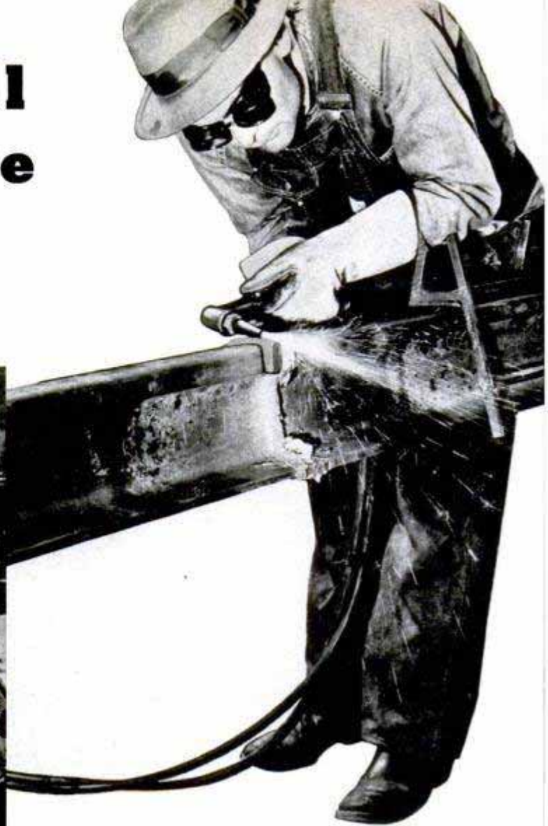
In five minutes, the pressure weld is completed. A hand torch, above, trims excess metal from the weld
