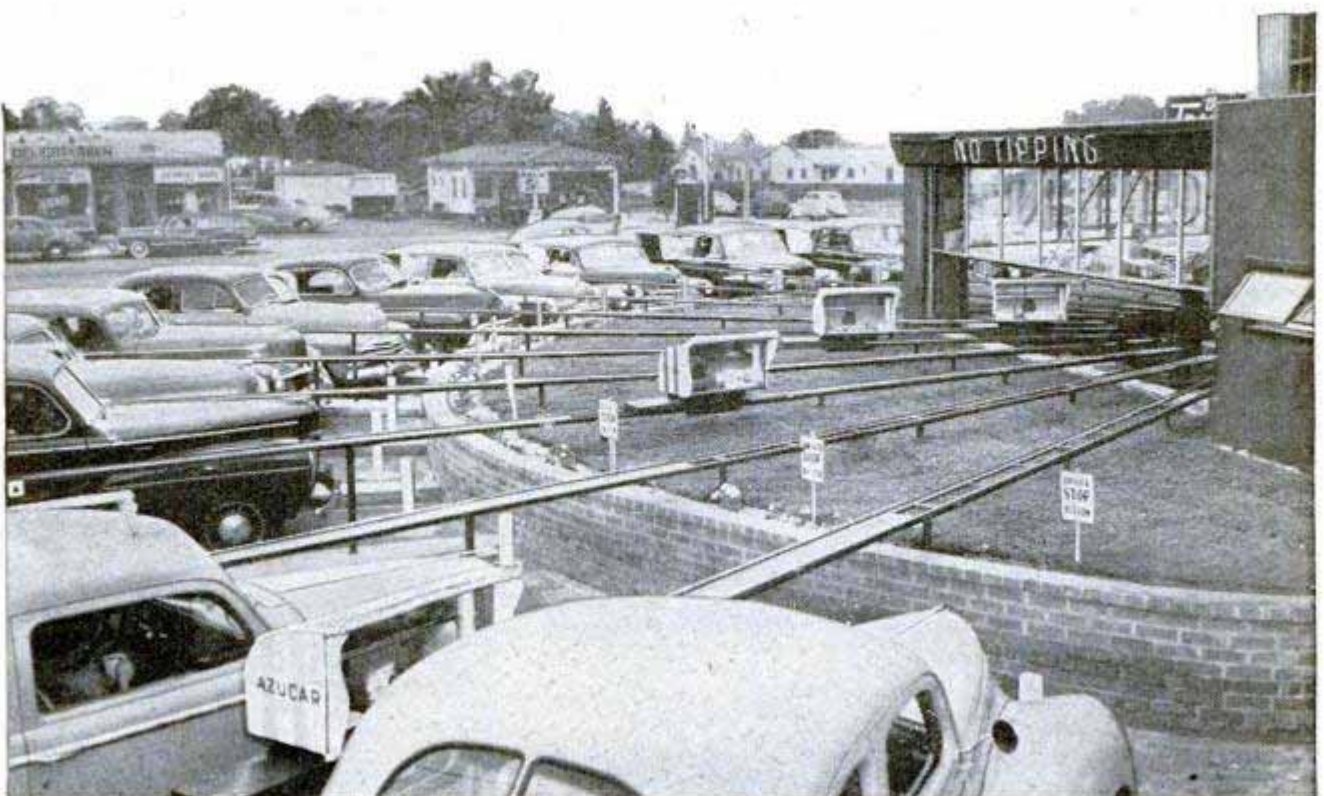
Box-type tray scoots along trestle to fill orders. It can be pulled laterally toward the car window. Below, when all 20 stalls are filled the trays shuttle along tracks continually
