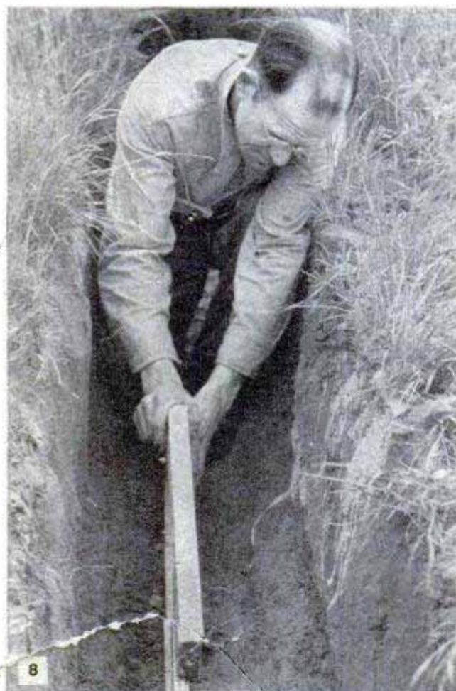
A long guide board fitted with sharpened stakes is an aid in digging a straight trench to correct grade
