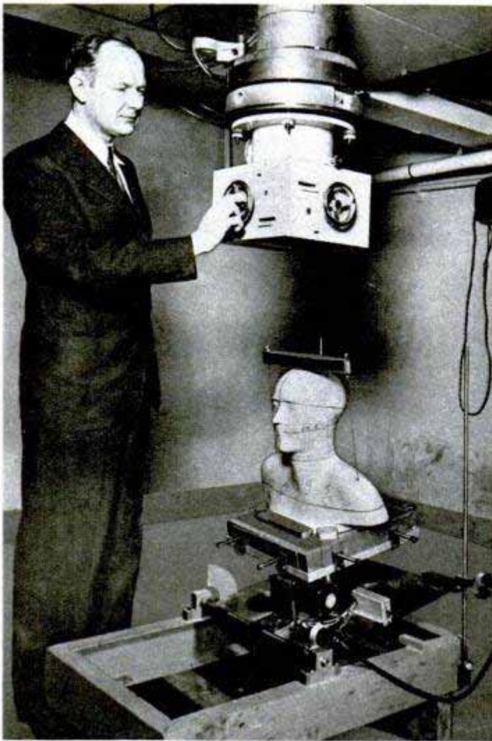
Above, film to record ray penetration goes in the head. Dummy is used to study effectiveness of X-rays in combating diseases of inner body
