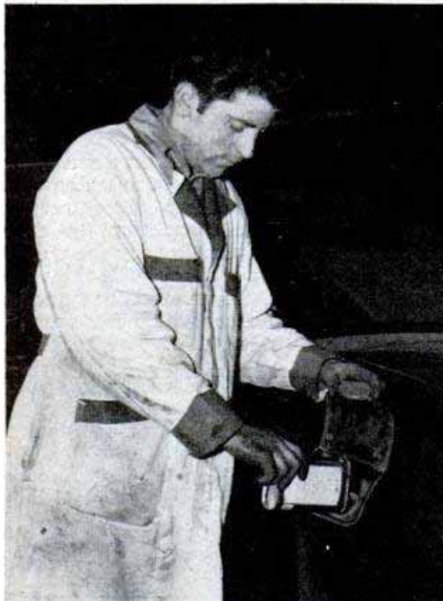
Below, solution can be added to gasoline to absorb water condensation and prevent freezing in fuel line
