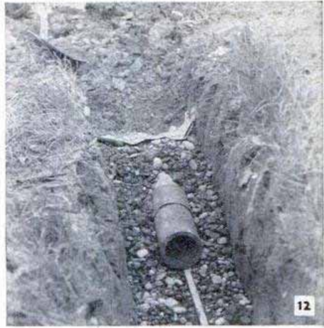
After laying and leveling to grade, tile line is covered with a layer of gravel as shown above and below
