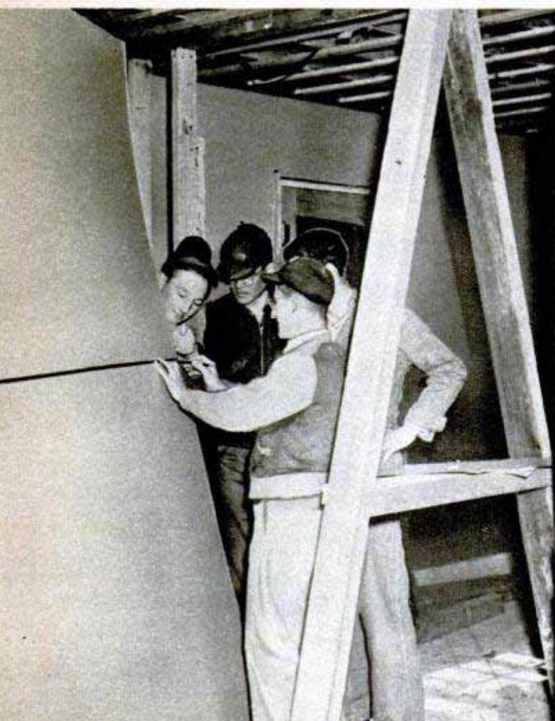
Above, two of the high-school home builders set the first ceiling square in the bedroom. Below, the boys' instructor, Maurice McElhiney, demonstrates the way to measure the wallboard sheet to assure an exact fit
