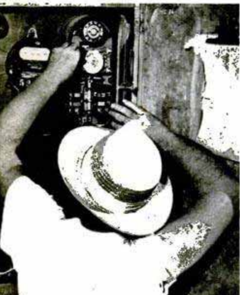
Torque-type clock turns beacon on at sunset, off at dawn, automatically adjusting to seasonal variation. Lee adjusts it, left, then oils the code cam, right. As cam turns, it makes contact for a long flash, two shorts
