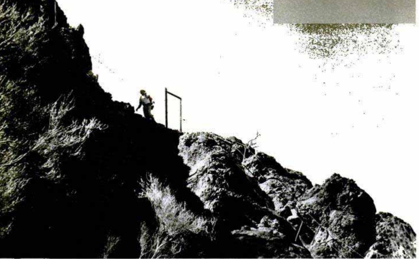
Rugged trail to the beacon is three miles and almost vertical. C.C.C. boys built it and strung the guide ropes
