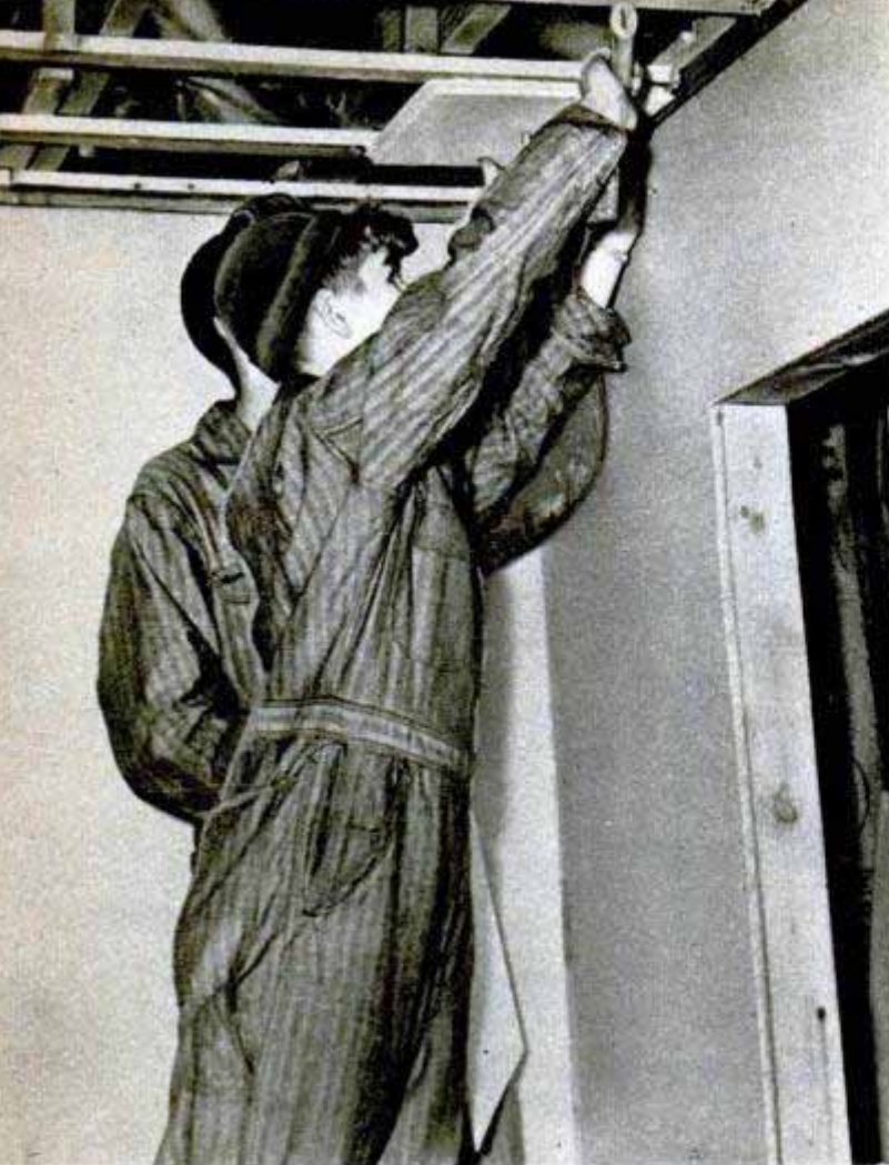
Above, two of the high-school home builders set the first ceiling square in the bedroom. Below, the boys' instructor, Maurice McElhiney, demonstrates the way to measure the wallboard sheet to assure an exact fit
