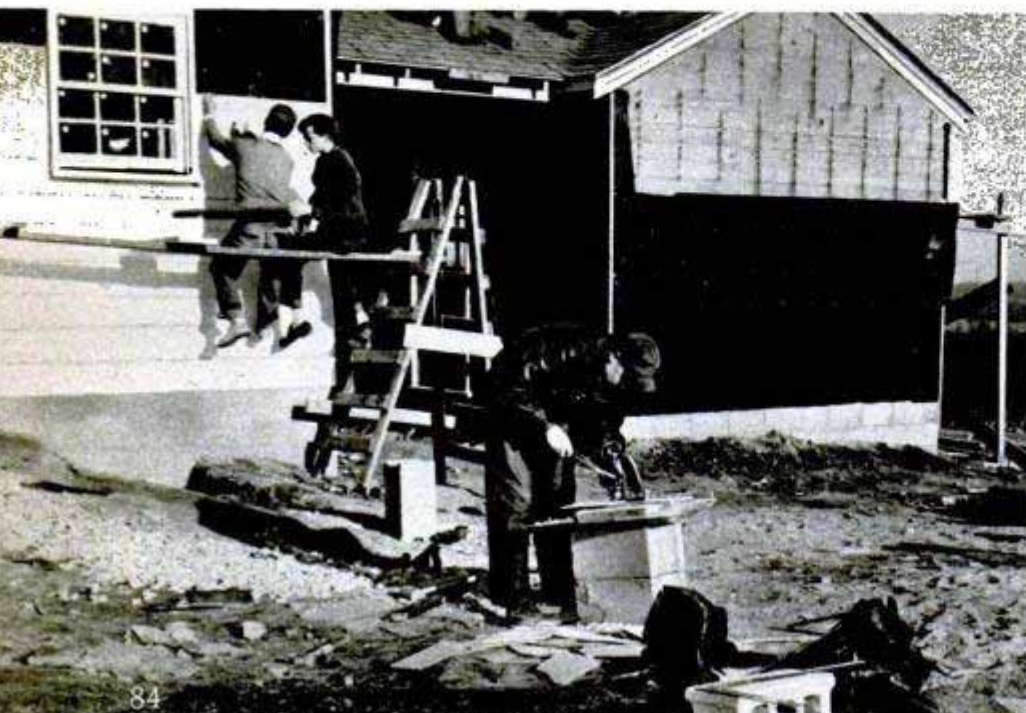
Above, roofing goes on fast with a half-dozen hammers pounding. Here, the high-school students nail down the shingles on the breezeway roof. Below, as the crew puts up siding, a helper cuts the shingles to size
