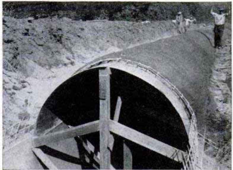
Above, concrete is sprayed on mesh to form lower half of pipe. Above, right, when lower half has set, wooden forms are built to support steel plates. Right, the completed pipe before inner forms have been removed
