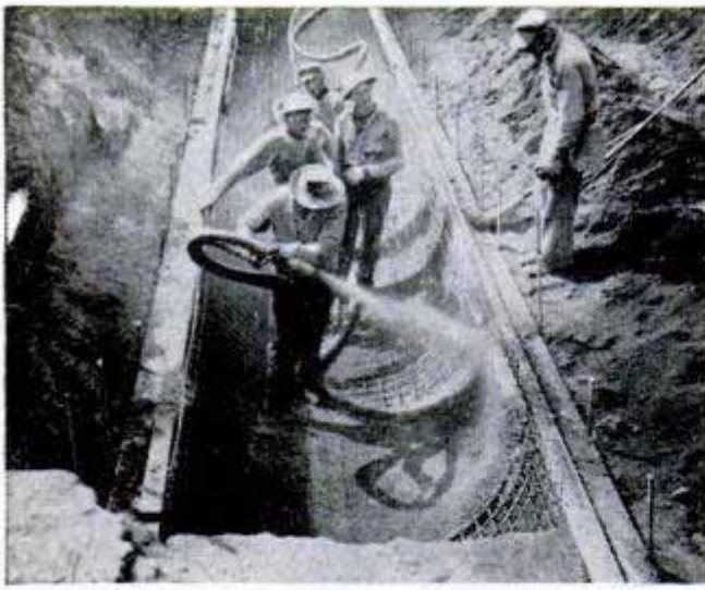
Above, concrete is sprayed on mesh to form lower half of pipe. Above, right, when lower half has set, wooden forms are built to support steel plates. Right, the completed pipe before inner forms have been removed
