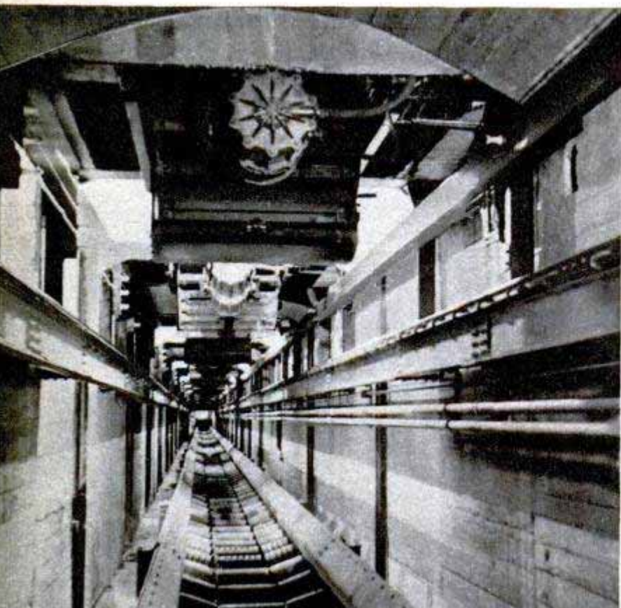
As efficient as a section of the New York subway, the underground conveyor system carries ore to the river loading bridge
