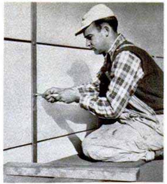
Left, two men can handle a roof plank of wood-aggregate concrete. Right, an aluminum batten seals wall joint
