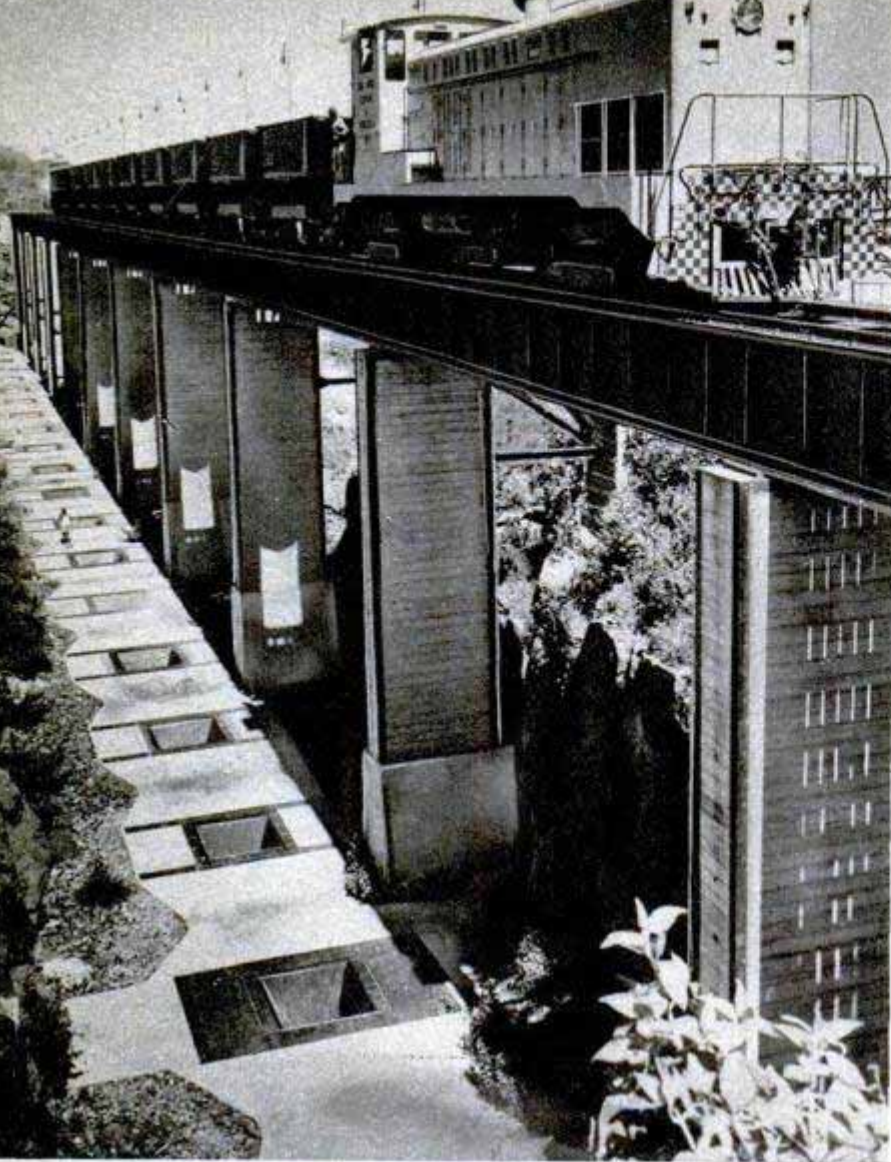
Diesel locomotive pulls ore cars along the top of the dumping structure. Chutes at the base drop ore into a conveyor tunnel
