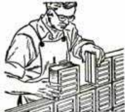
2. Glass Blocks fit into framing, using prefabricated wood strips.
