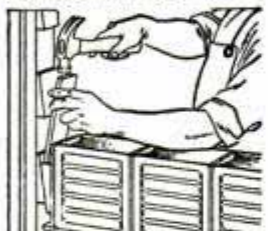
3. Wedges anchor each row firmly. Simple tools are all you need.
