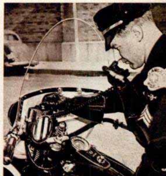
Transmitters on motorcycles are distributed between two boxes flanking rear wheel to equalize the weight
