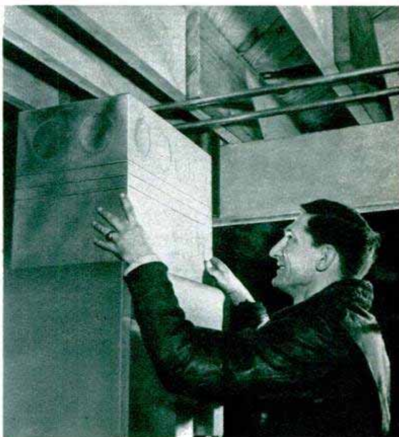
Above, fitting the plenum chamber to the top of the furnace. Circles near top are punched out to take the stovepipe ducts. Top left, installing a register between studs, showing the use of four-inch stovepipe. Left, completed installation of wall register
