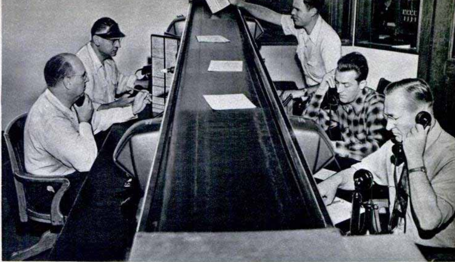
Incoming calls for police assistance are received at complaint telephone board. Messages are then put on endless belt and carried to dispatcher in microphone room next door, the "radio central" of the system
