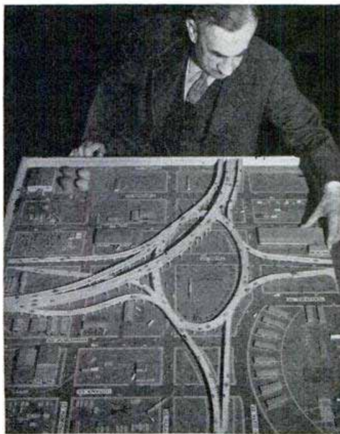
Model of the rotary system shows how traffic will be collected and distributed for the southern crossing. Elevated roadways will eliminate the local traffic
