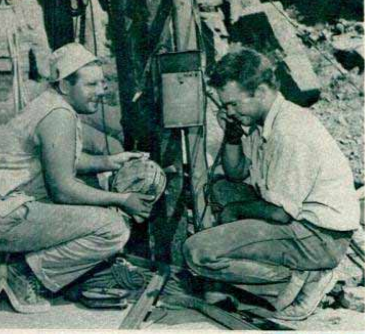
Army-surplus telephones connect all points on guano transportation system. Right, entrance to cave is a slit 10 feet wide and 30 feet high. Workers climb the ladders in foreground to scale 100 feet of vertical cliffside
