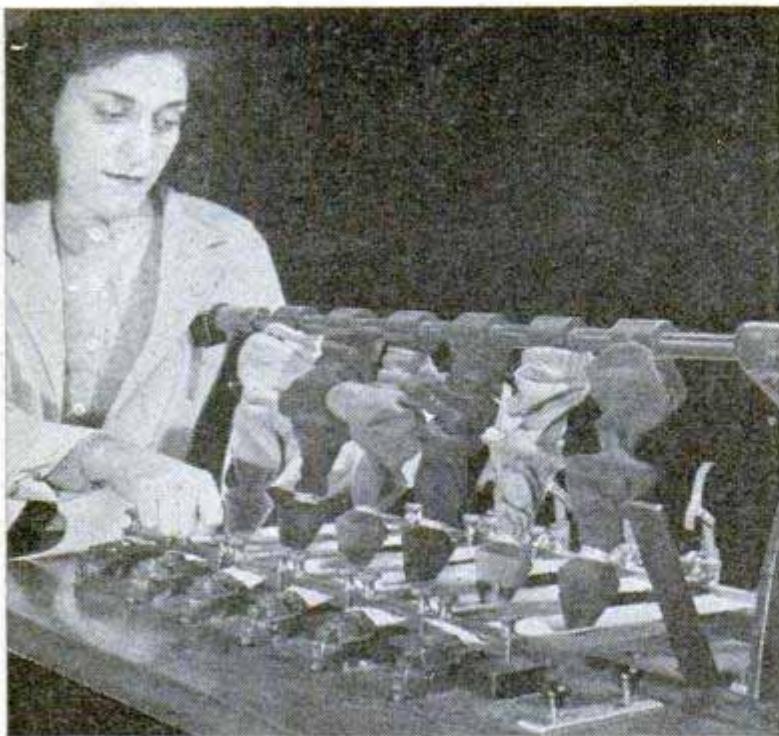
This machine rubs socks 20,000 times to test their durability
