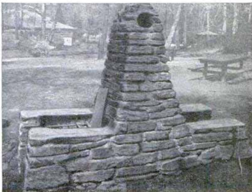
No previous experience in bricklaying is necessary to build a serviceable fireplace like the one shown in the lower left-hand picture. The double fireplace, below, right, has two separate fireboxes, both using a single flue. Built of stone, it is economical for small camps where it serves the purpose of two fireplaces
