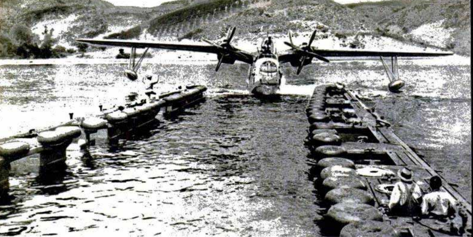
Water jets on each side of the entrance "steer" a flying boat into the submerged dry dock for hull repairs
