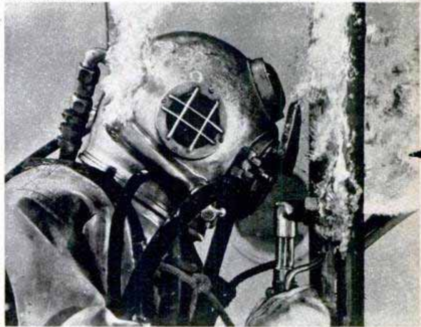
Diver stands on stage ready to be lowered to sub's deck for first physical contact with the disabled craft. Below, when wreckage holds up rescue work, divers cut it away with hydrogen underwater torches U. S. Navy photo
