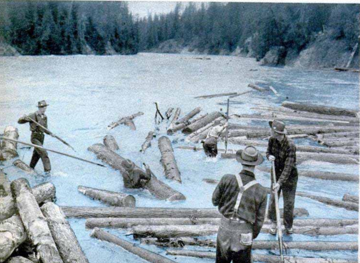
When the riverjacks can't break up the jam with their peavey hooks, a dynamite charge blasts the logs loose. Below, two of the crew are in the icy water as they start the logs moving on the down-river end of the jam
