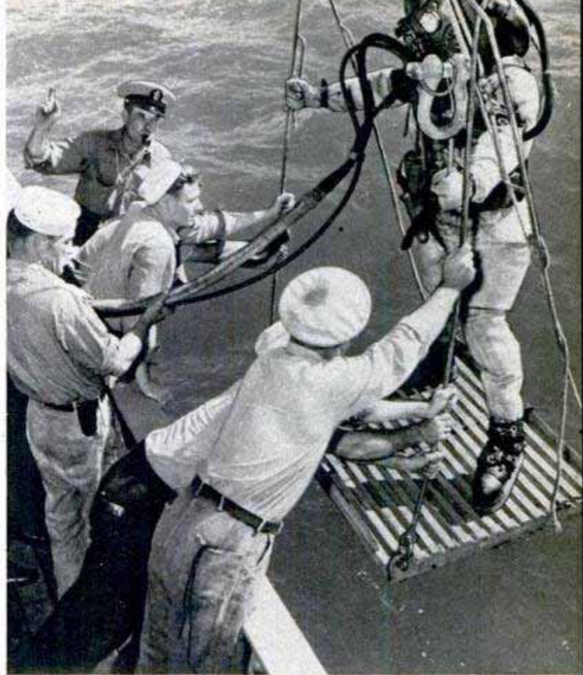
Diver stands on stage ready to be lowered to sub's deck for first physical contact with the disabled craft. Below, when wreckage holds up rescue work, divers cut it away with hydrogen underwater torches U. S. Navy photo
