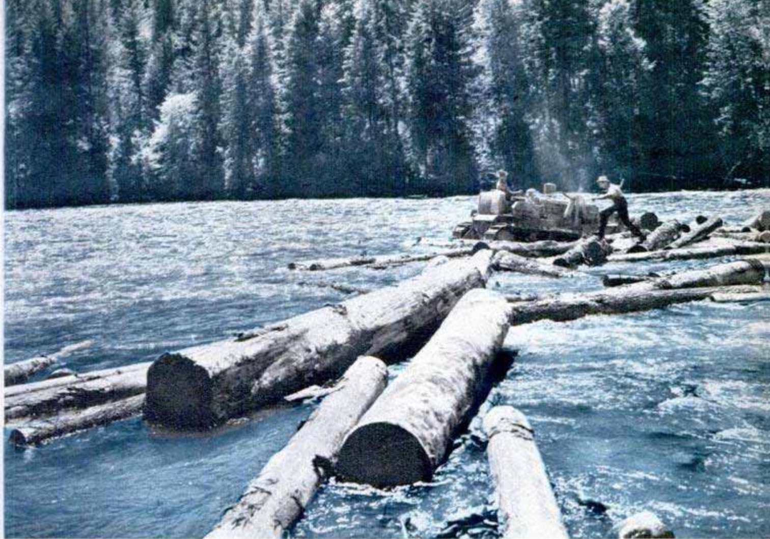
Downstream where the riverbanks are not steep, a bulldozer is used to break up the log jams near the shore
