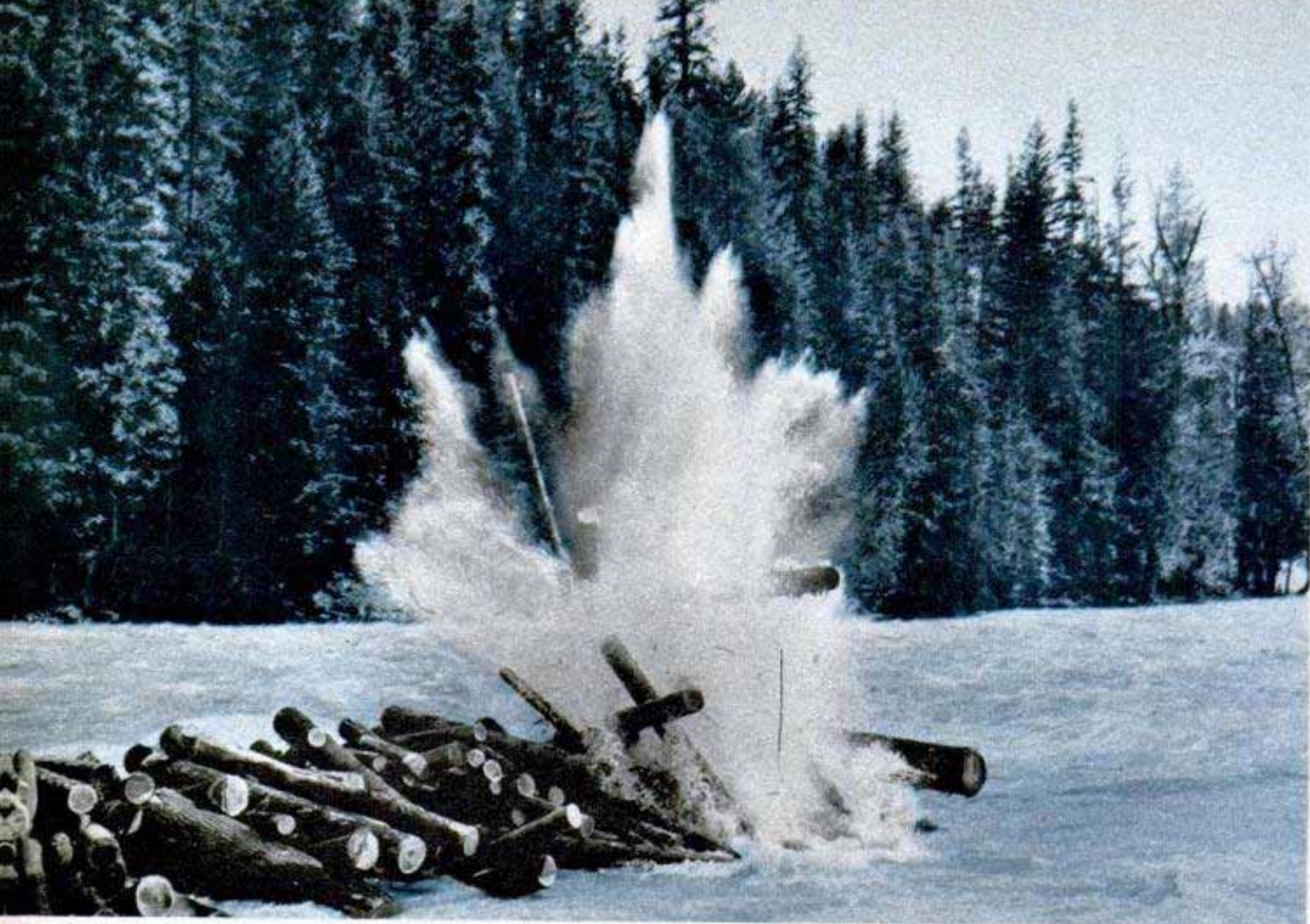
When the riverjacks can't break up the jam with their peavey hooks, a dynamite charge blasts the logs loose. Below, two of the crew are in the icy water as they start the logs moving on the down-river end of the jam
