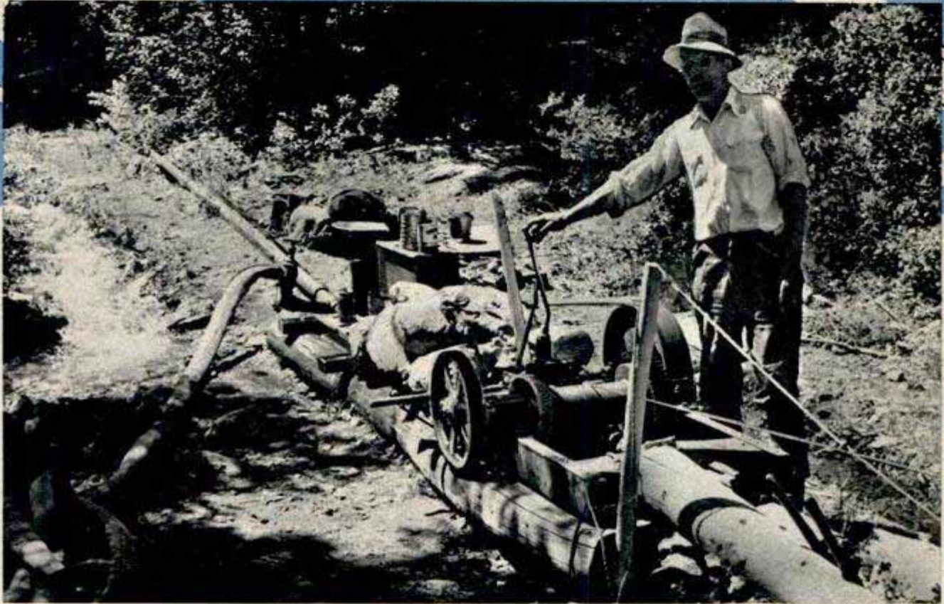
Top, sketch shows over-all plan of Sweet's homemade gold mine. Above, winch-and-gear system was built around old Chevrolet transmission. Below, water wheel is turned by gravity-flow stream piped from creek
