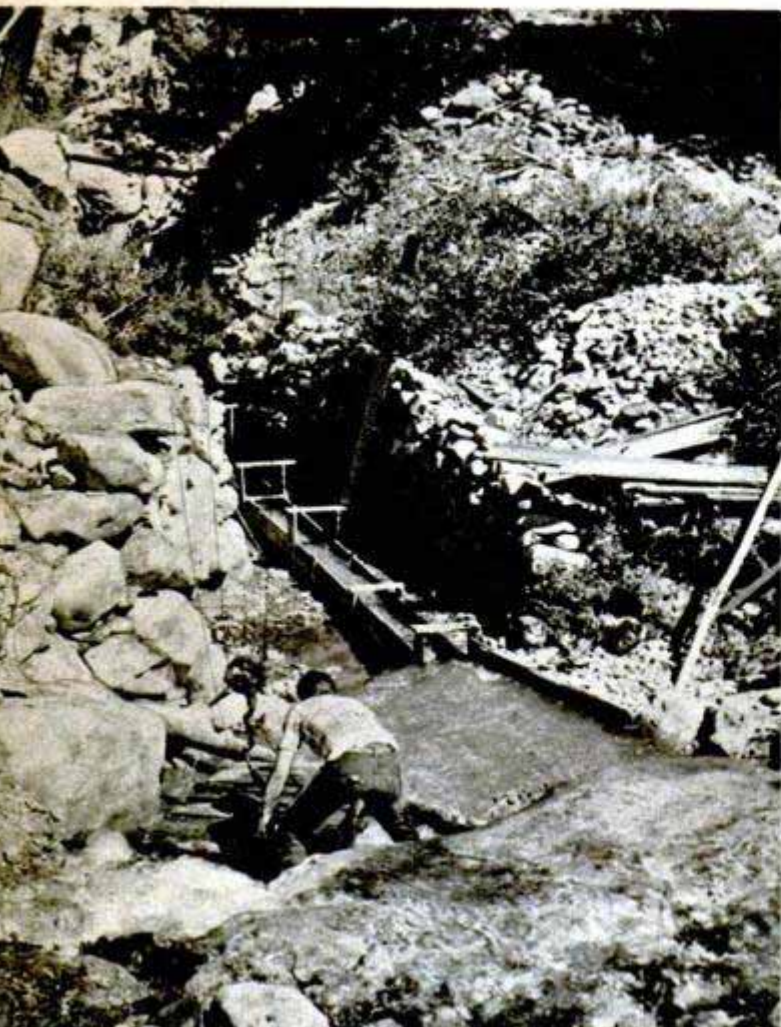
Jib crane operated by water-power system can lift a ton of boulders out of the diggings. Below, sluice box, lined on bottom with burlap and cleats, catches the gold as rushing waters wash the metal into it
