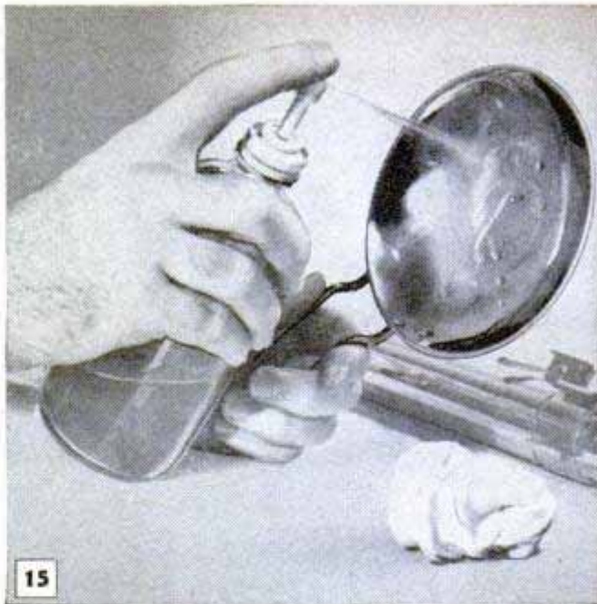
15 Reflectors can be kept clean and bright with carbon tetrachloride. Polish the surface with a soft cloth
