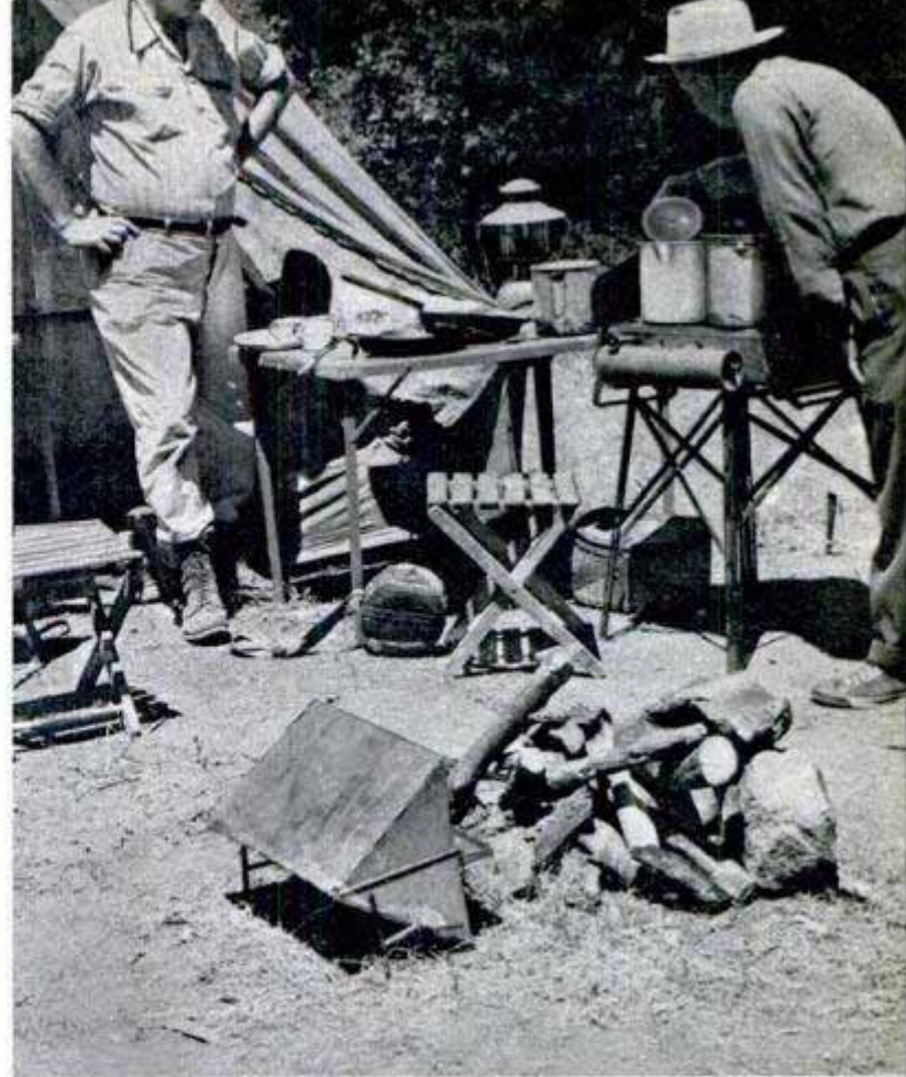
Compact camp kitchen provides most of the comforts of home. Note reflector oven in front of the fire
