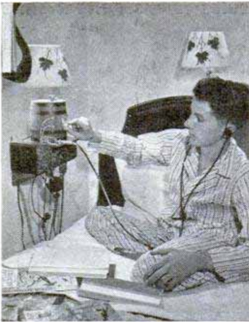
Left, Jimmie tunes in a program on the radio he built from an old keg, a crystal, wires and earphones. He contrived the automatic timer, right, to turn on hen-house lights early to give chickens longer working day
