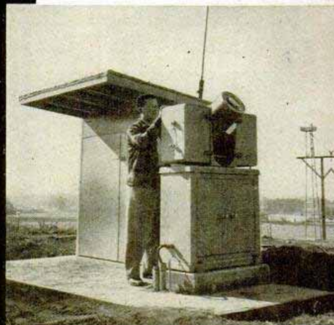
Each of the diagonal units of the slope-line lighting system pierces the sky with ten 500-watt landing lamps. Above right, diagrams show appearance of the slope lines to an incoming pilot when he is above, on and below the glide path
