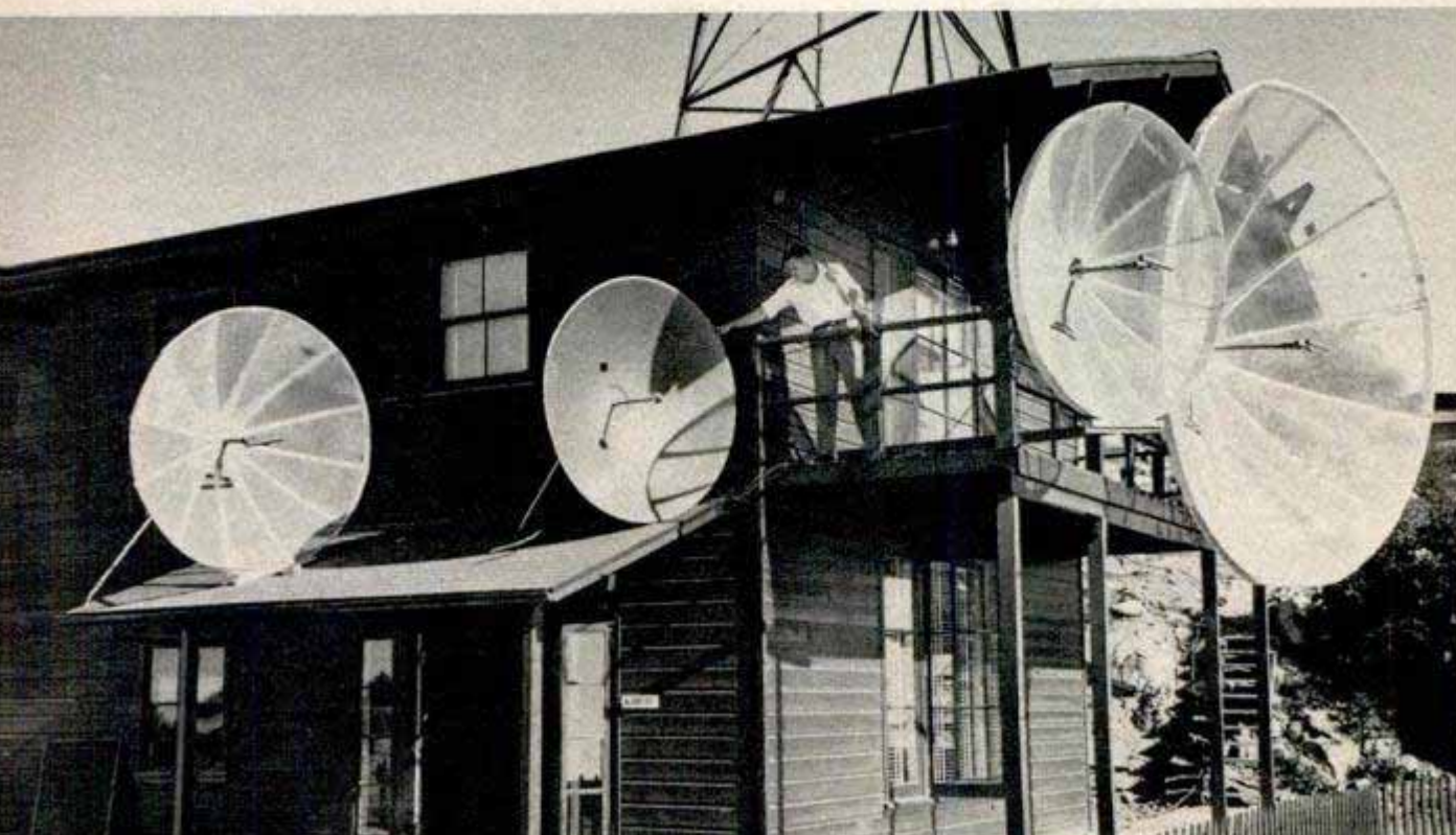
Above, turnstile tower has 20 "batwing" elements (half at right angles). Below, left to right, four dishpan antennas pick up incoming sound beams, studio picture beams and pictures from two mobile transmitters
