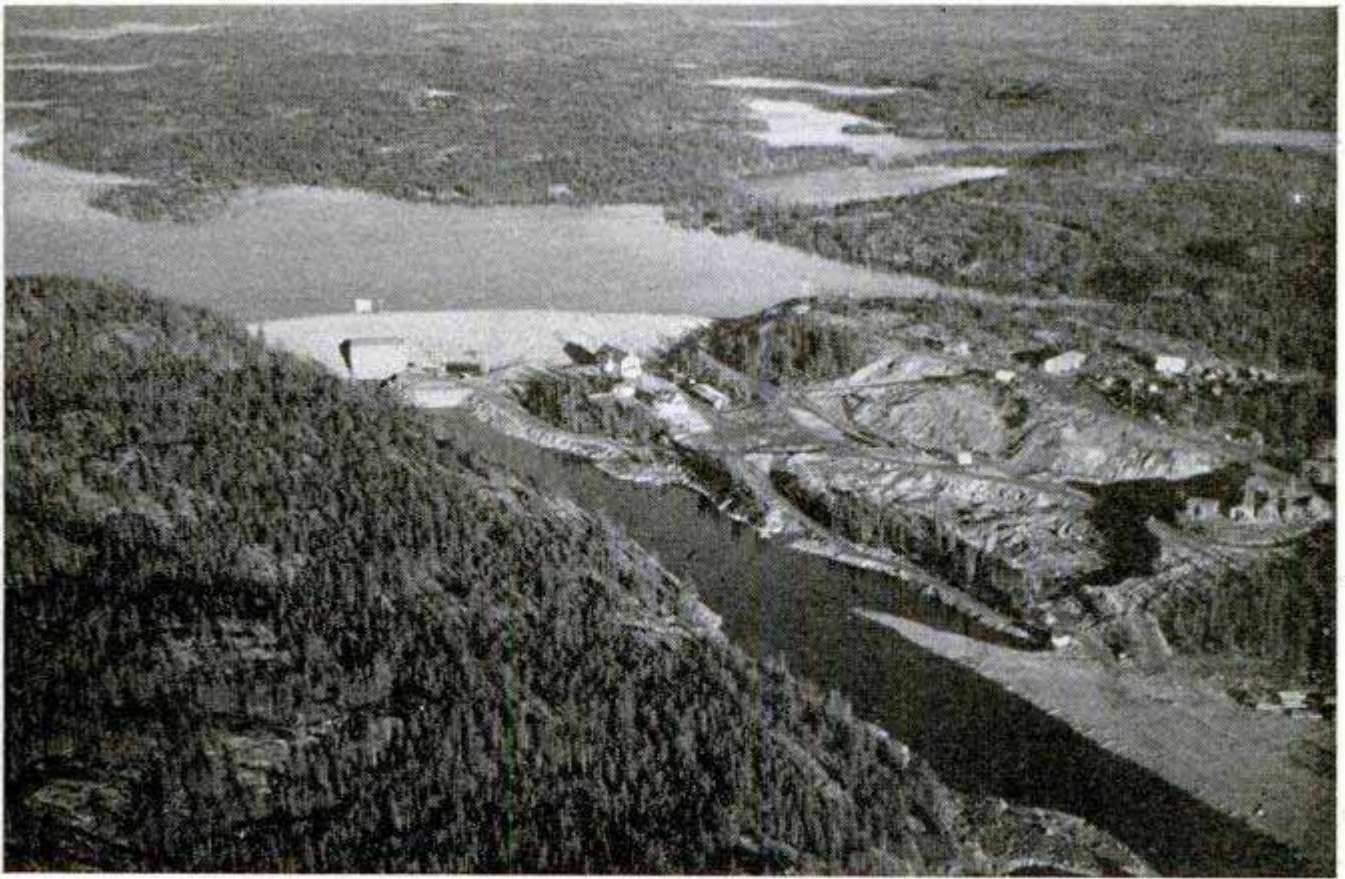
Marking the frontier of industrialization in Canada's northland is this dam and power station at Snare River
