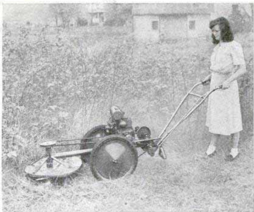
Above, one of many attachments for handy power unit cuts weeds and thick brush. Other attachments at left from top to bottom are rotary hoe (hopper holds weights), buzz saw, power lawn mower
