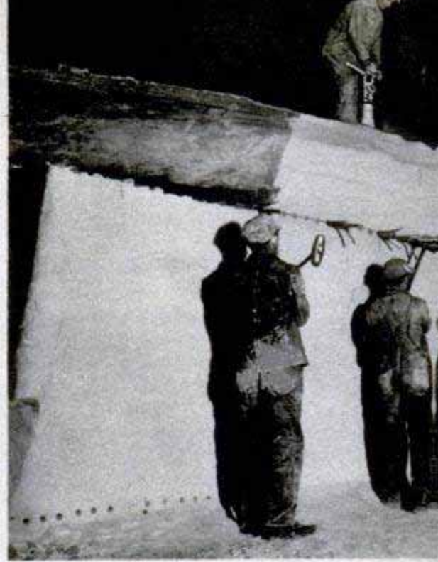
Above, quarrymen pound wedges into holes in the marble to loosen the layer of waste rock on top. Left, big block of marble leaves quarry on its way to the mill
