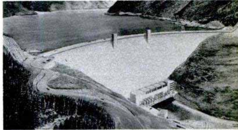
Sketch of Hungry Horse Dam, being built in Montana. It will contain three million cubic yards of concrete. Below, earthmovers peeled back the earth's surface in digging this 200-foot pit which exposes vein of coal
