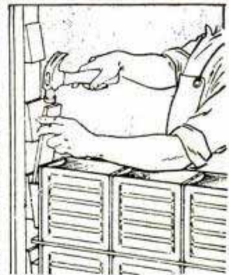
← Blocks set in tiers are separated by wood strips. Above, vertical strips are inserted between blocks. Right, glass wall is anchored in place with wedges
