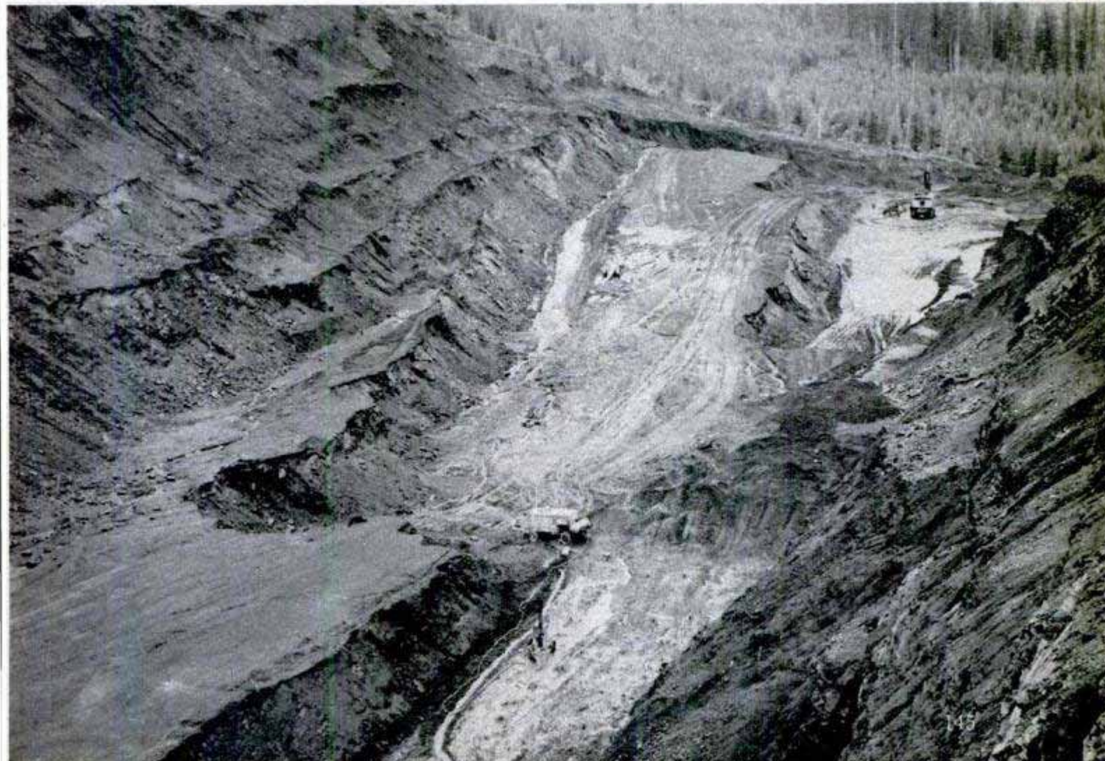
Sketch of Hungry Horse Dam, being built in Montana. It will contain three million cubic yards of concrete. Below, earthmovers peeled back the earth's surface in digging this 200-foot pit which exposes vein of coal
