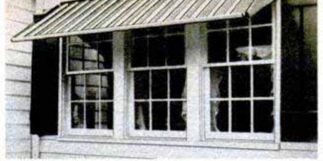
ALUMINUM AWNING can be made to fit any width. You assemble six-inch sections on the job (below)
