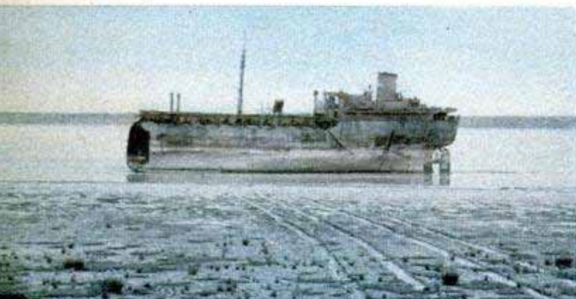
Anchorage, Alaska, needed additional power so M-K engineers moved section of broken tanker into place and used ship's engine to generate electricity. Below, this 1500-bed hospital was built in Honolulu
