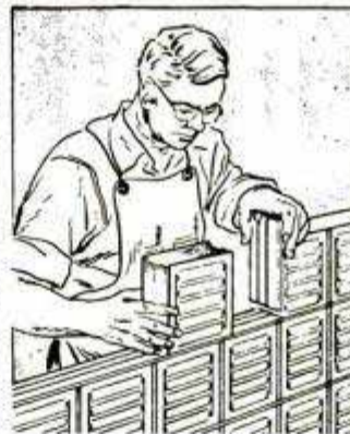
← Blocks set in tiers are separated by wood strips. Above, vertical strips are inserted between blocks. Right, glass wall is anchored in place with wedges
