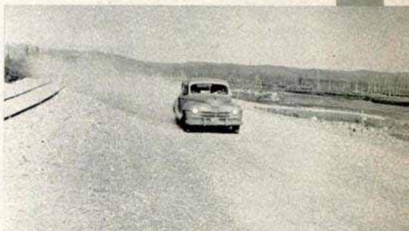
Projected paving of the final 70 miles, next year, will eliminate hazardous dust clouds shown above
