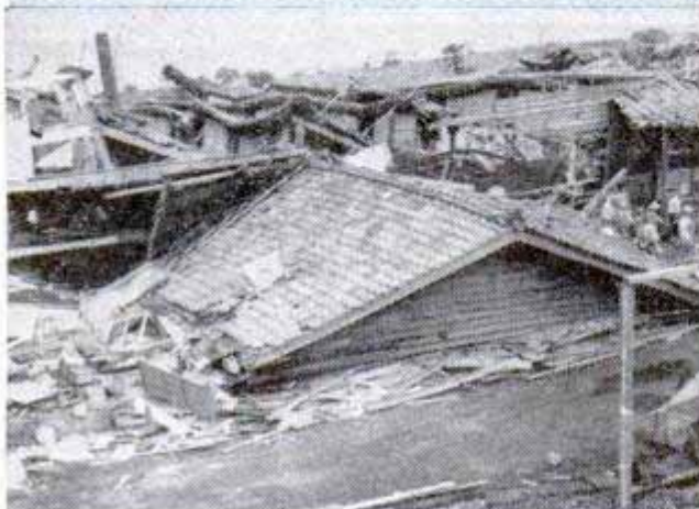
Below, top-heavy Japanese houses were flattened by the earthquake. The cheaply constructed buildings stand little chance when a big shake occurs. Right, Japanese train was flipped over like a toy
