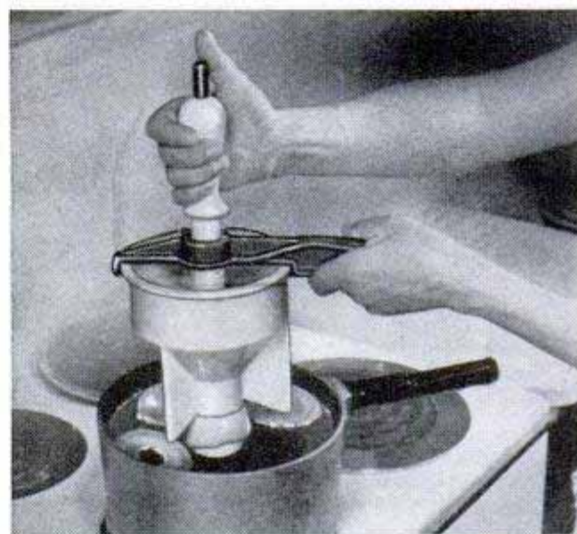
DOUGHNUT MAKER eliminates rolling and cutting. You pour batter in base of utensil, doughnuts are formed as you push plunger
