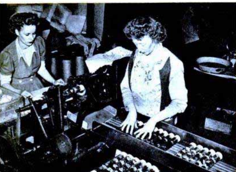
Crimping machine designed by Fred V. Richardson and built in his shop puts the crimp in sheets of crepe paper used in making the crackers. Below, "squeeze" machine puts the final touch on these party favors
