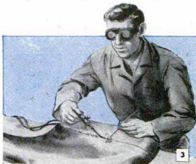
Finally, the repair part is welded to the fender and hammered to conform to shape at the lower edge
