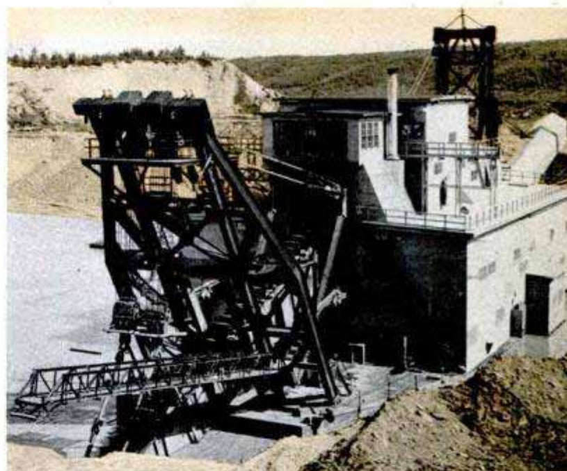
Modern counterparts of the old prospectors are the enormous gold dredges working north of Fairbanks. Gravel is scooped up and carried inside where the ore is separated, and waste is expelled at the rear
