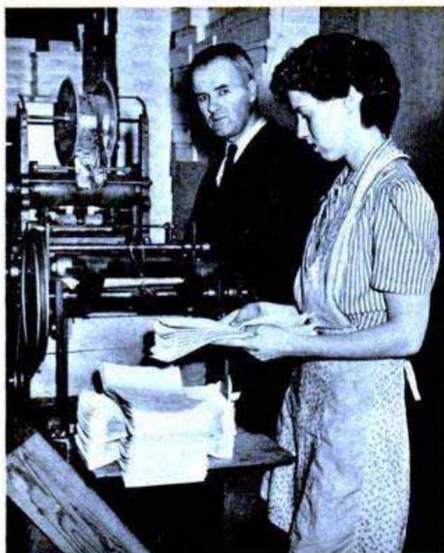
Crimping machine designed by Fred V. Richardson and built in his shop puts the crimp in sheets of crepe paper used in making the crackers. Below, "squeeze" machine puts the final touch on these party favors
