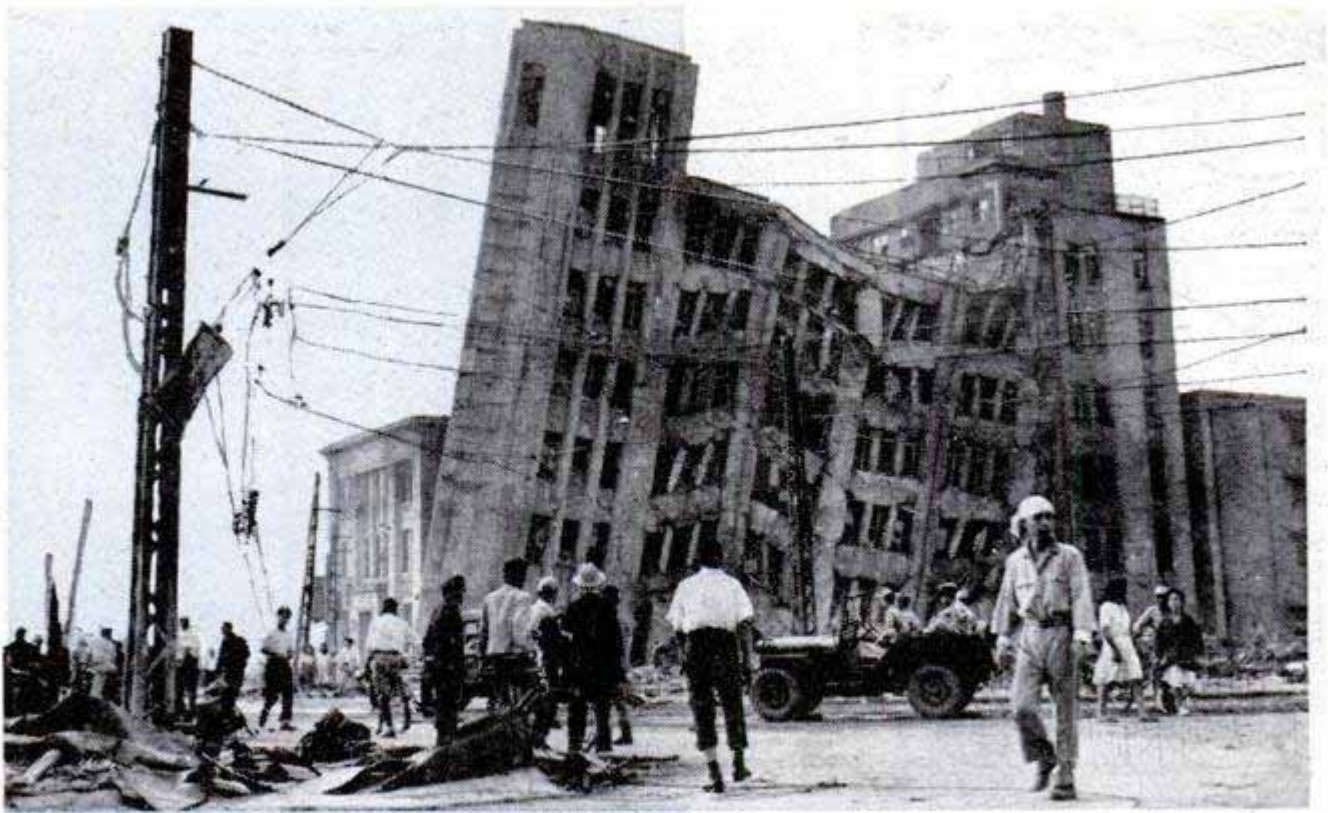
Above, these photos of devastation of the recent earthquake in Japan show how poorly constructed building crumbled. Below, the sturdy structure built years ago withstood the sharp vibrations
