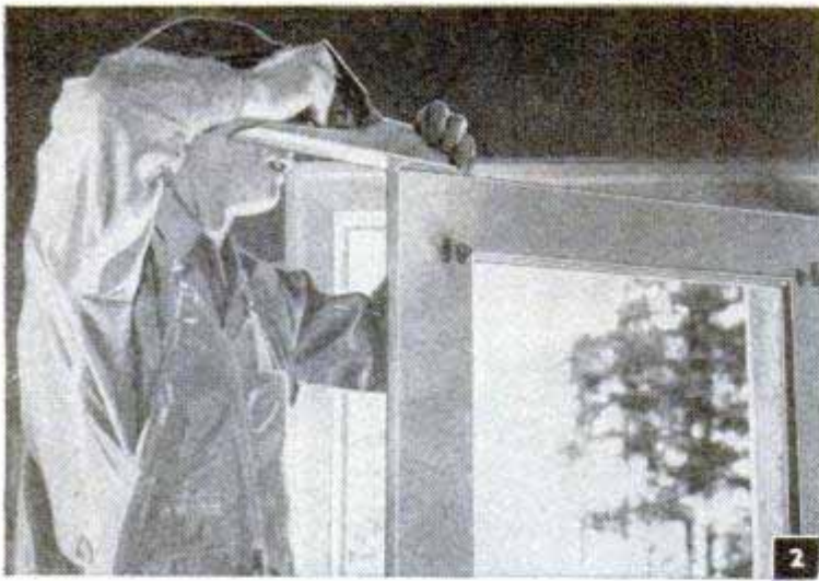
Before weather-stripping a door, true it up to assure uniform clearance between door and jamb. Be sure to plane edges square
