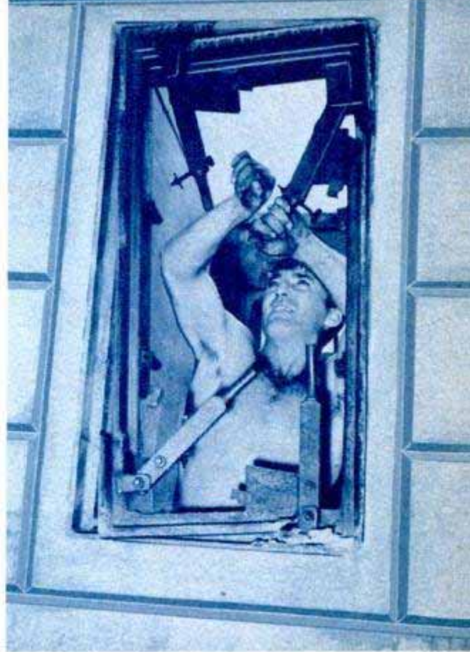
Left, removing the interior form from the living room. Right, collapsible forms are used for the windows
