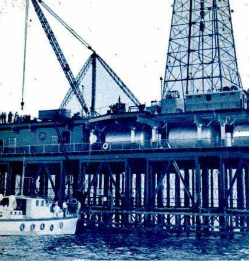
Crane lifts equipment and supplies aboard the platform. The tanks in the foreground hold fresh water
