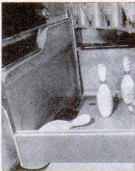
Front view of automatic spotter, after pins have dropped into place. Right, sweeper shoving pins off alley
