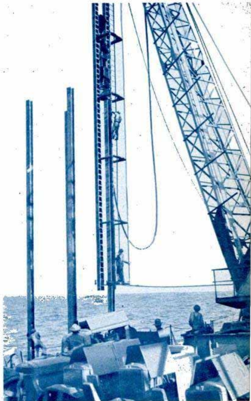
↓ Crane swings a template into place. A network of 25 of these templates forms foundation for platform. Right, pilings are inserted into templates and then sunk deep into the ocean floor to give firm support
