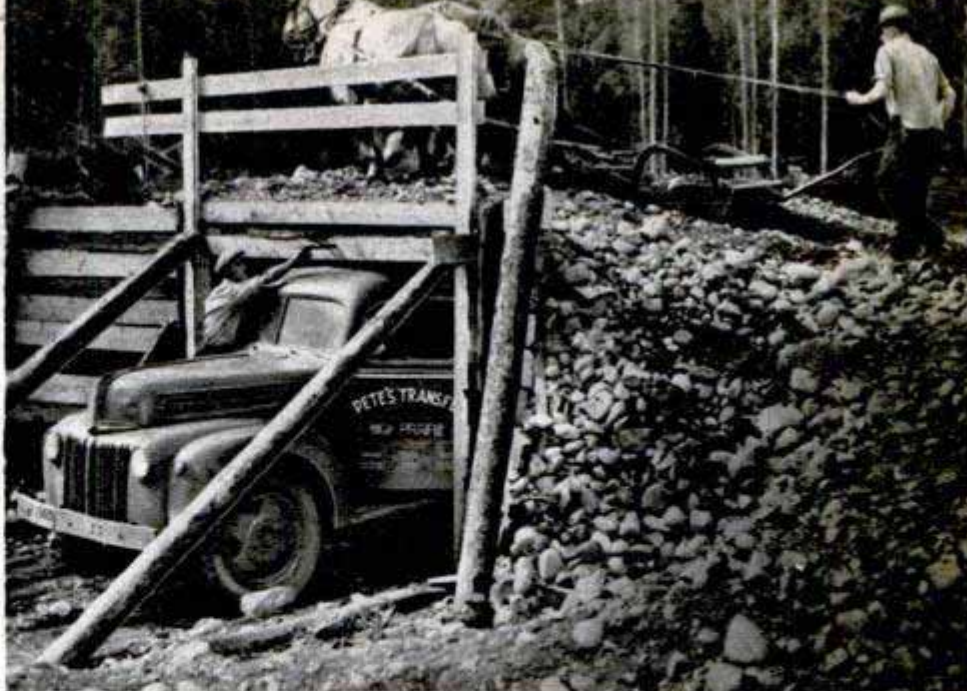
Pete Elder's homemade gravel loader, in use near High Prairie, Alta., typifies the pioneer ingenuity demonstrated along the way
