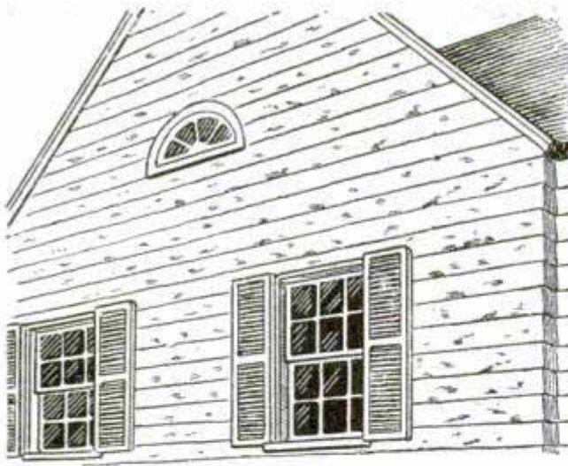
3 Blistering and peeling of paint are more often due to dampness within the walls than to any other common cause
