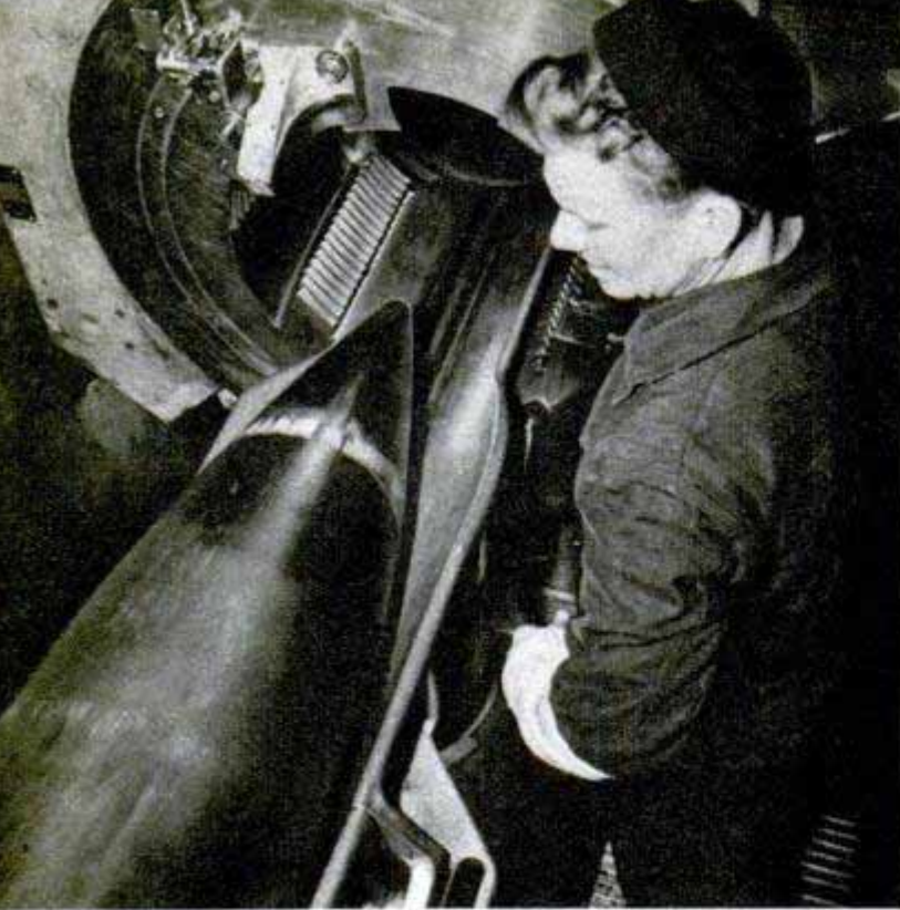
One-ton shell slips easily into the breech of 16-inch gun. The effective range of the missile is 20 miles
