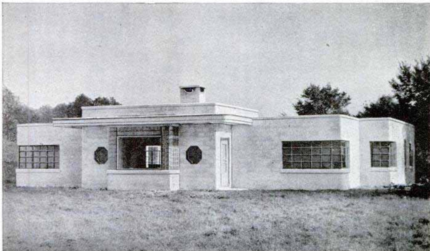
Above, Celocrete units made of slag-concrete are fireproof and have excellent insulating qualities as this photograph proves. Below, a modern one-story home near Cleveland built with blocks of Celocrete
