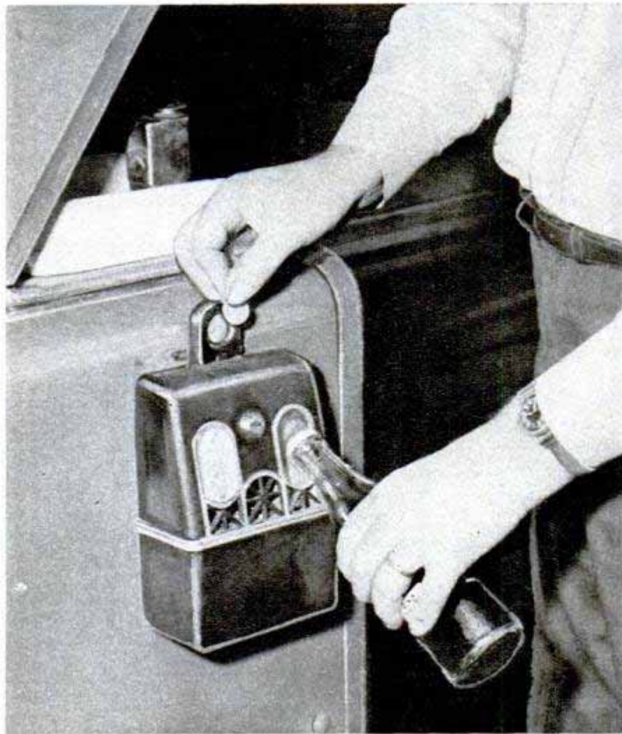
Staff member delves into the problem of developing a high-intensity ignition system for combustion engines that will operate on a vacuum tube. ↓ Coin-operated bottle opener is one of the institute's developments. It foils the customer who helps himself to a soft drink but forgets to pay
