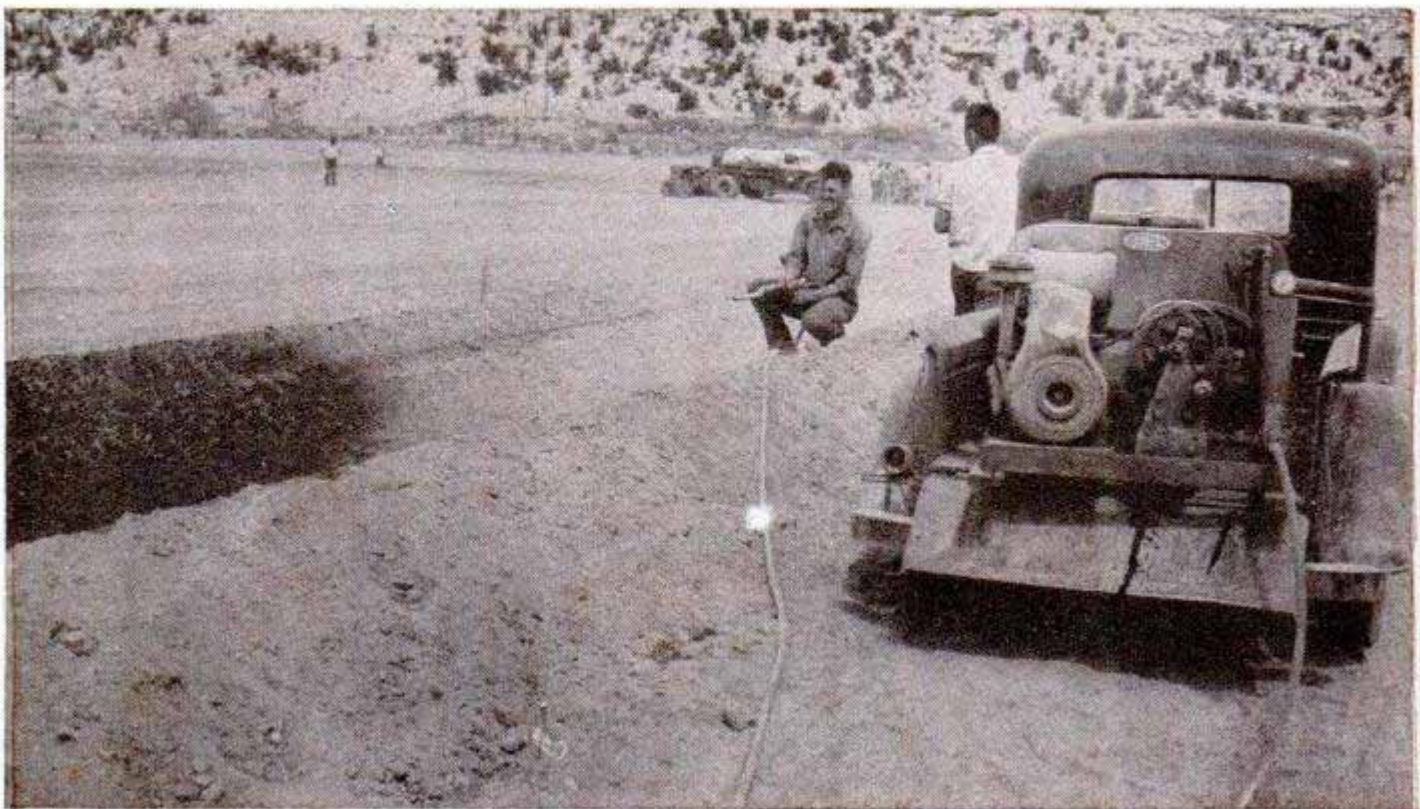
Unlined irrigation ditches are sprayed with heavy oil which forms a crust to prevent ditch-bank erosion
