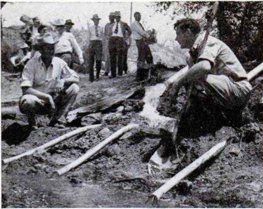
Aluminum siphon tubes shift water from main channel to smaller ditches. They eliminate need for headgates, are inexpensive and primed by hand
