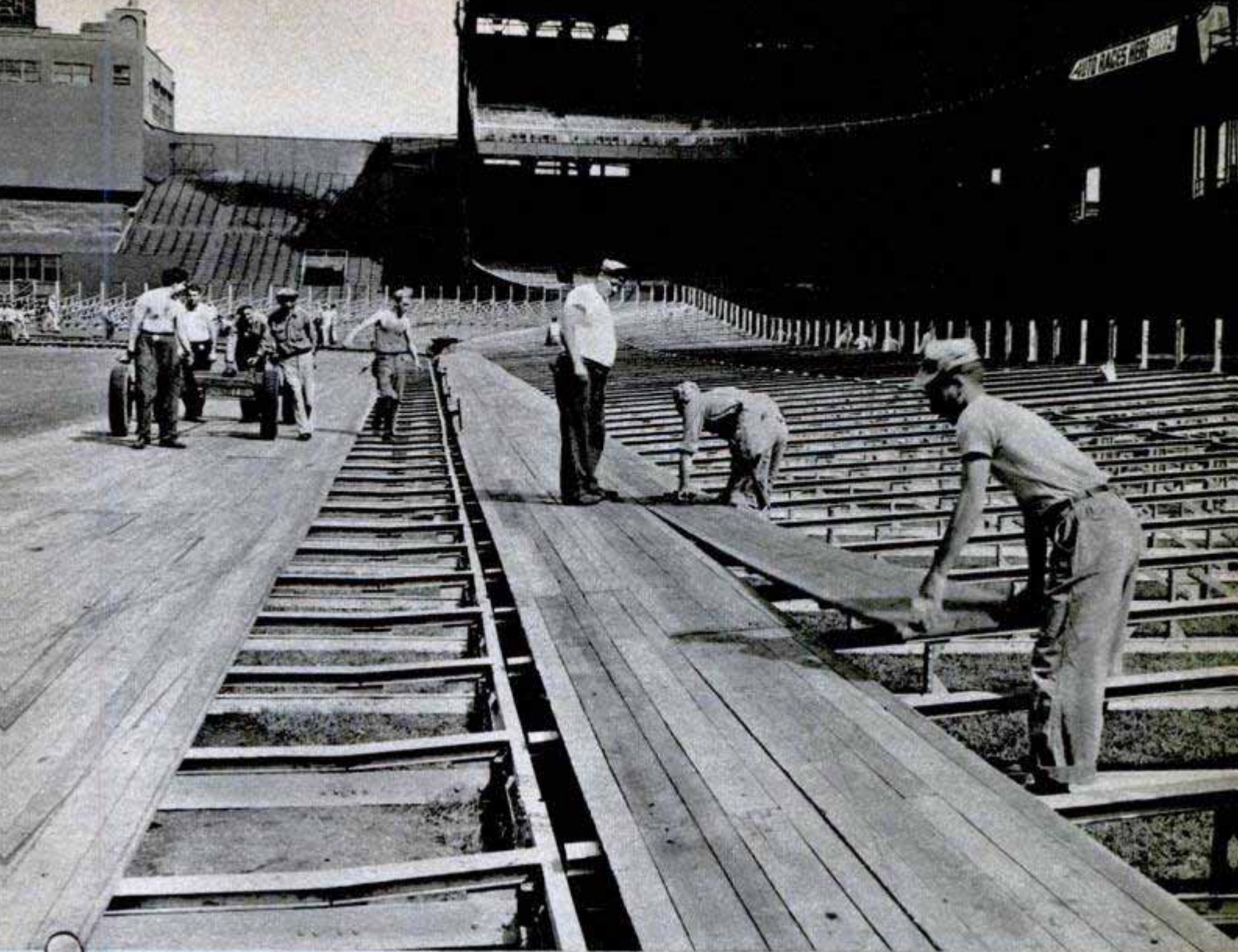
Pine boards locked together with tongue and grooves and cleats form the racing surface. Pine gives excellent traction and absorbs the oil
