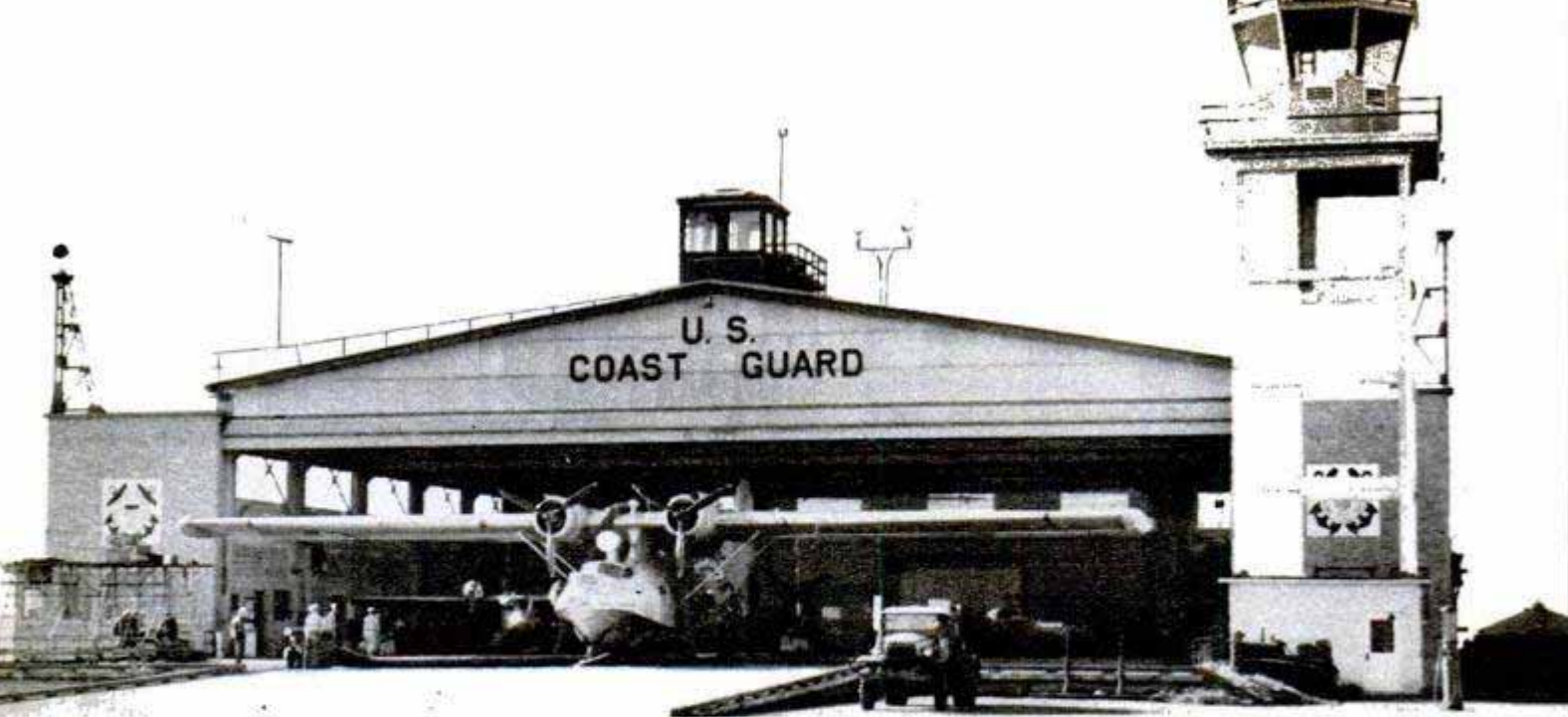
Combination lighthouse and airport beacon is mounted on top of tower at right of hangar. Below, adjusting astronomical clock that turns light on at sunset, off at sunrise. Sun relay at right does the same thing
