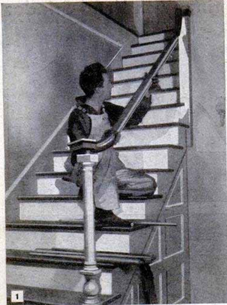
Above, stair rails of the type shown consist of a number of precut parts made from selected hardwoods. Below, layout of stair is based on normal length of step on a level floor
