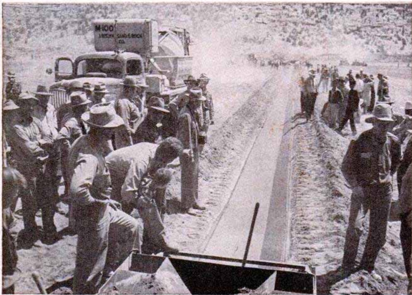
Ditch-lining machine feeds ready-mixed concrete from barrel trucks into the sides and bottom of the ditch. Below, this is the scene 18 minutes after the ditch was started. About 600 feet have been lined with concrete
