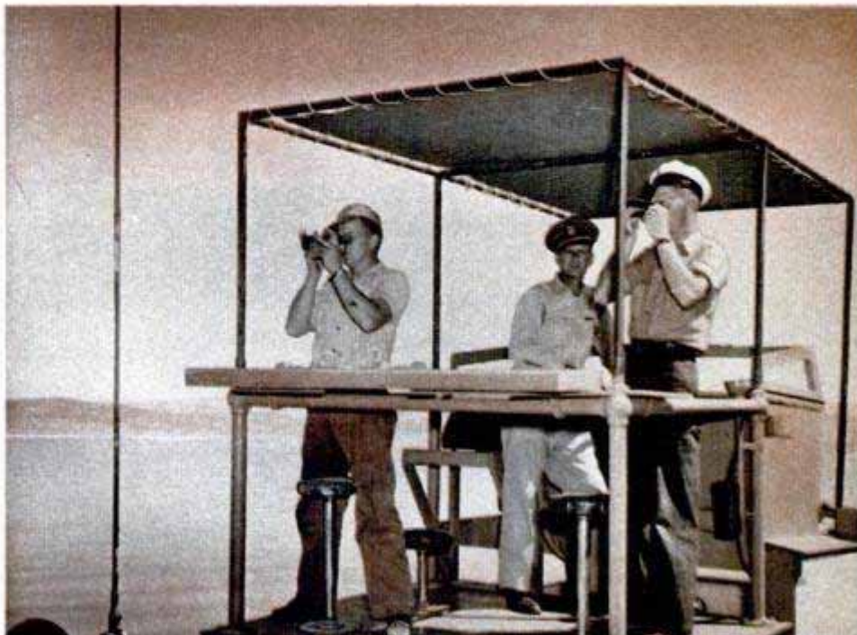
Sounding boat used in silt survey carries sensitive fathometer and when reading is made sailors (right) take bearings on two shore markers to determine their exact location on lake. The Navy is cooperating in survey
