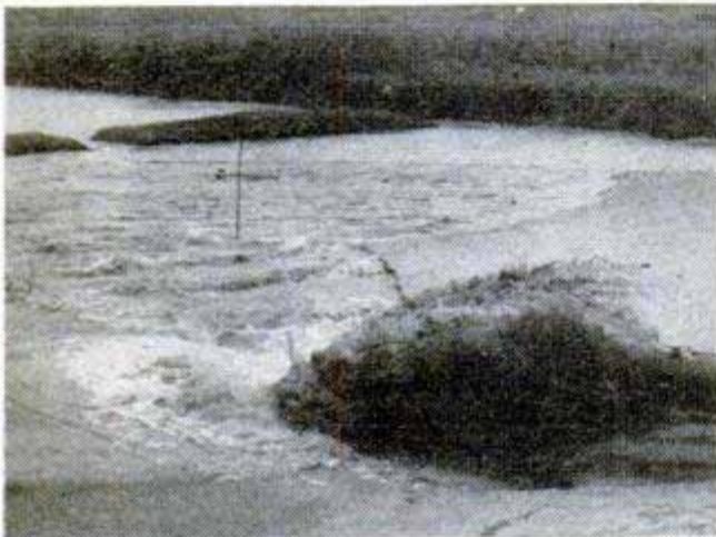
Above, about 850 cubic yards of silt an hour gush from end of pipe. Below, locations of dredge, pipe, shoulders and drainage ditch are shown on the map
