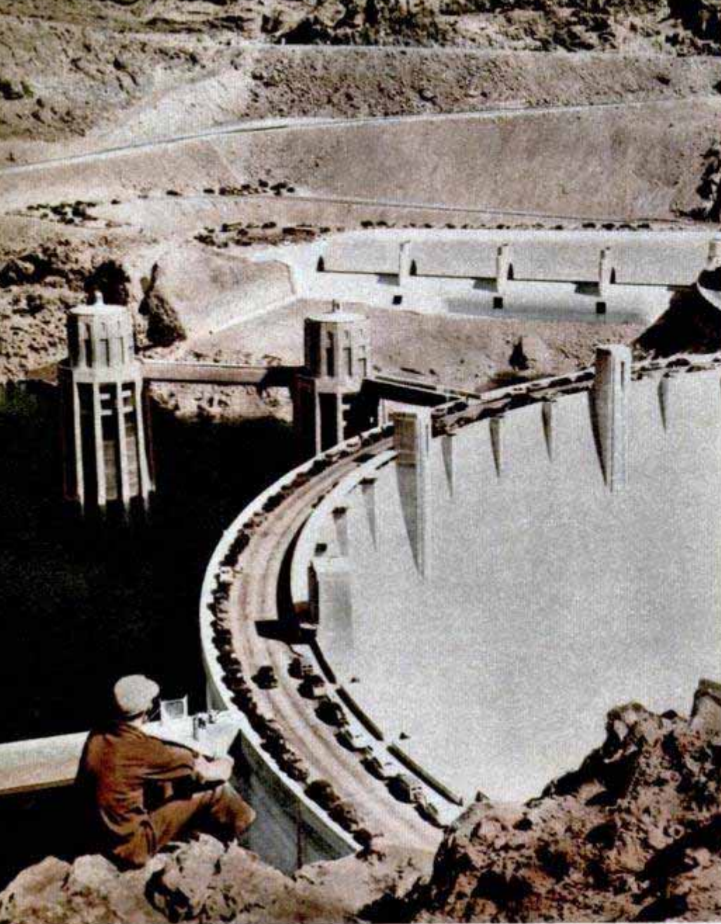
Some day silt may clog intake towers behind dam which supply turbines
