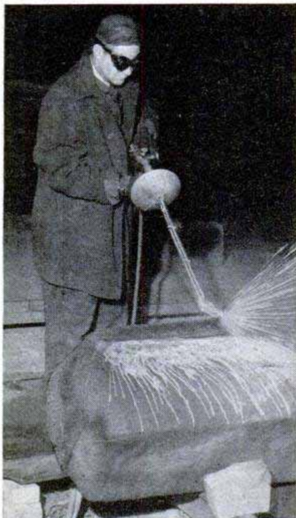
Left, hand-operated powder torch cuts stainless steel in foundry. The hilt on torch protects worker against intense heat. Right, machine cutting torch with the powder dispenser (foreground) connected to it by hoses
