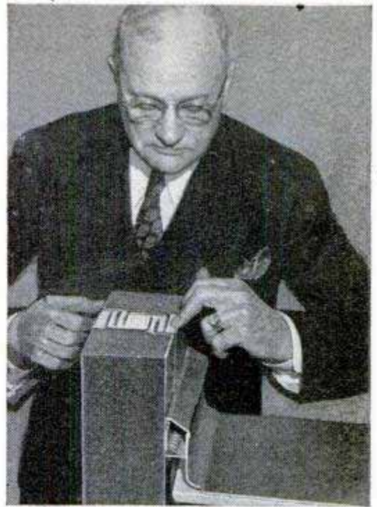
Fireproof plaster seals joint. Note BX channel in baseboard →
