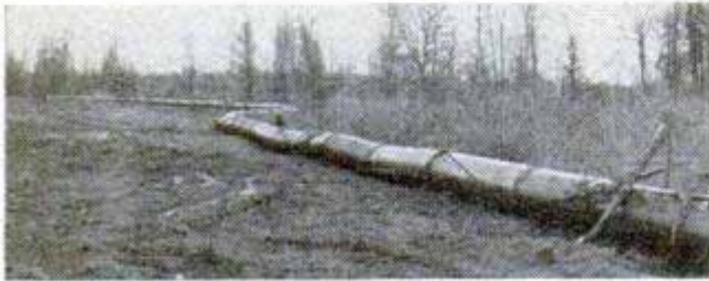
Reversing normal erosion, this dredge sucks silt from river bed to form shoulders for highway. Pipe that carries silt floats in foreground. Below, pipe snakes across fields carrying its load of silt-laden water
