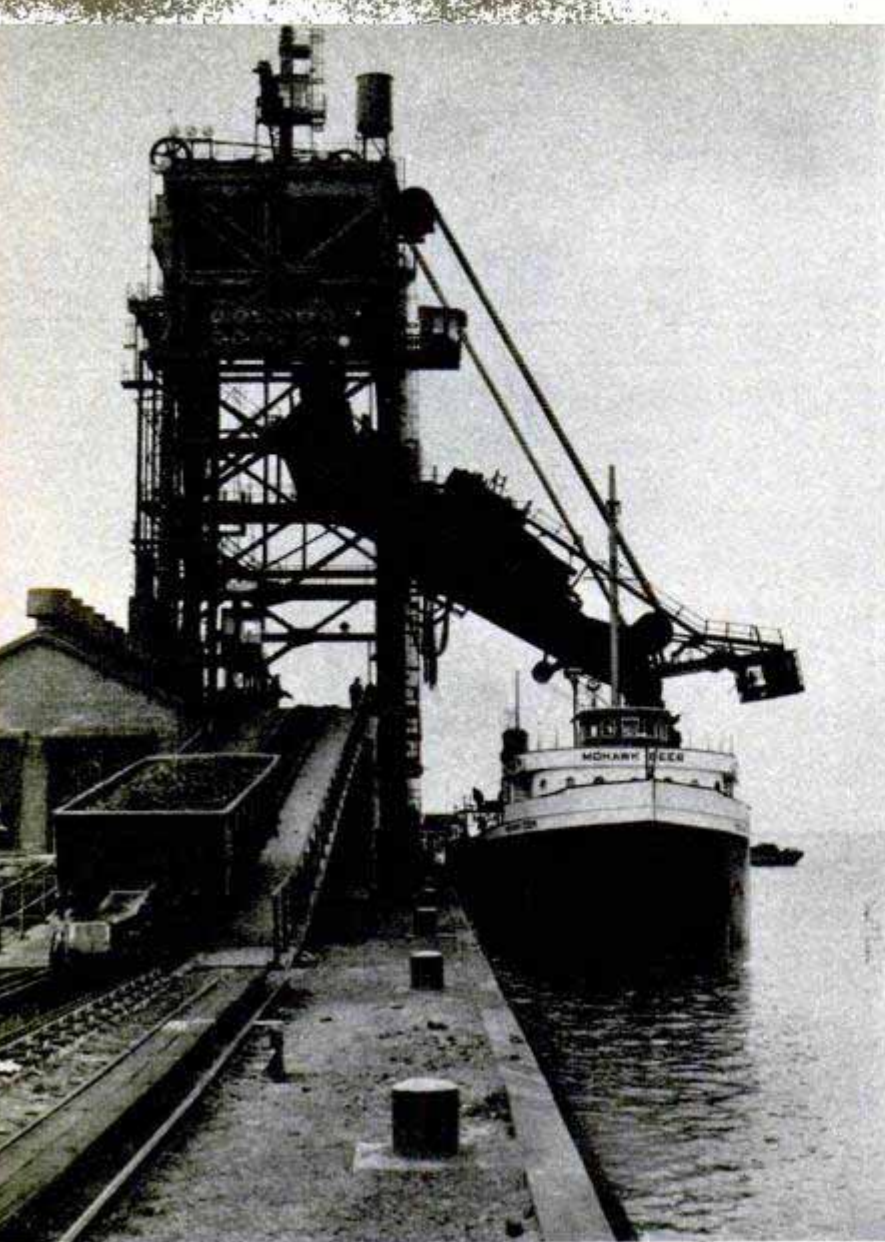
Carload of coal is pushed up the ramp to the dumper by pilotless barney locomotive. Below, the cable-operated barney comes up from its pit between rails to start car up the ramp
