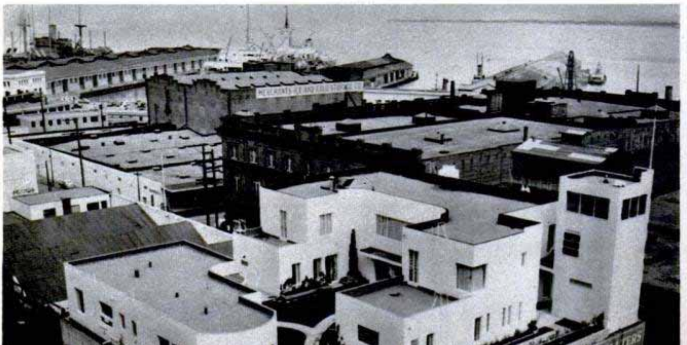
PENTHOUSE DELUXE has everything a country estate has except a garage. A luxuriant lawn separates the two buildings. Overlooking San Francisco's waterfront, it has a patio, sun deck, swimming pool and gardens
