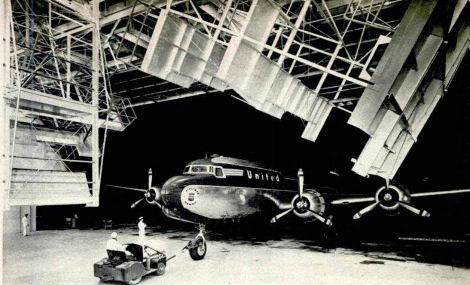
Halves of tail dock, upper right and in left background, drop into position when plane moves forward
