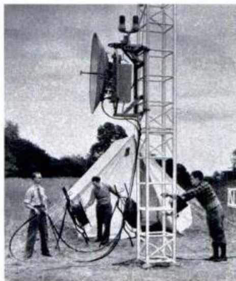
Left, tower being raised by hand winch. Section behind winch bar will be added when lifting is completed. Center, antenna carriage begins its trip to the tower top. Right, the 200-foot tower with antenna in place
