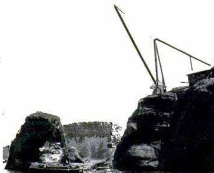
Long arm of a derrick hoists supplies to the lonely lighthouse on Tatoosh Island near Cape Flattery
