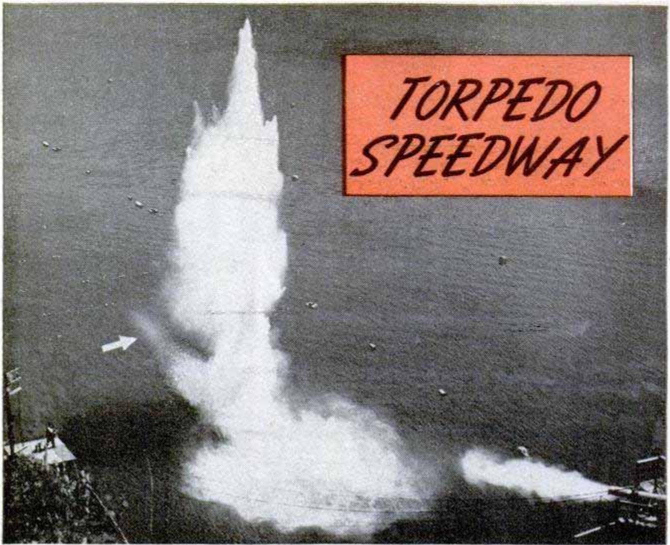
Arrow marks a torpedo launched from 300-foot tube running down a hillside at Morris Dam range
