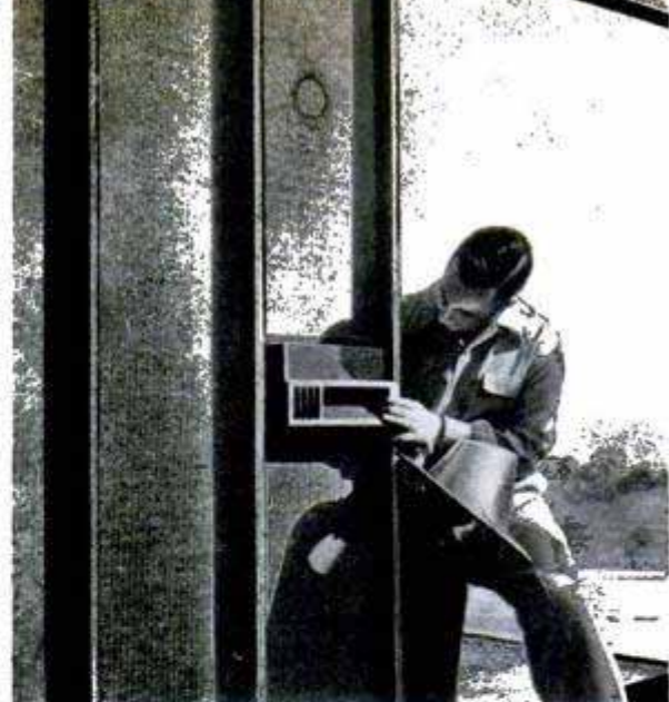
Above left, steel panels interlock to form the exterior walls. Above right, mailbox and door chimes are installed at the plant and go up with the walls. Left, close-up shows layer of Fiberglas laid above ceiling as insulation
