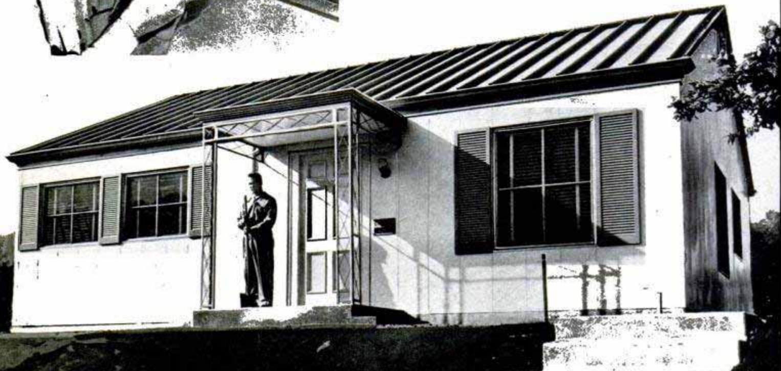
← Steel window sash fits into frame of extruded aluminum ↓ Completed bungalow, erected in two days, has a large living room, two bedrooms, kitchen, service porch and bath
