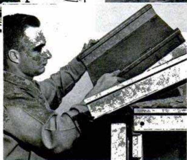
Above left, steel panels interlock to form the exterior walls. Above right, mailbox and door chimes are installed at the plant and go up with the walls. Left, close-up shows layer of Fiberglas laid above ceiling as insulation
