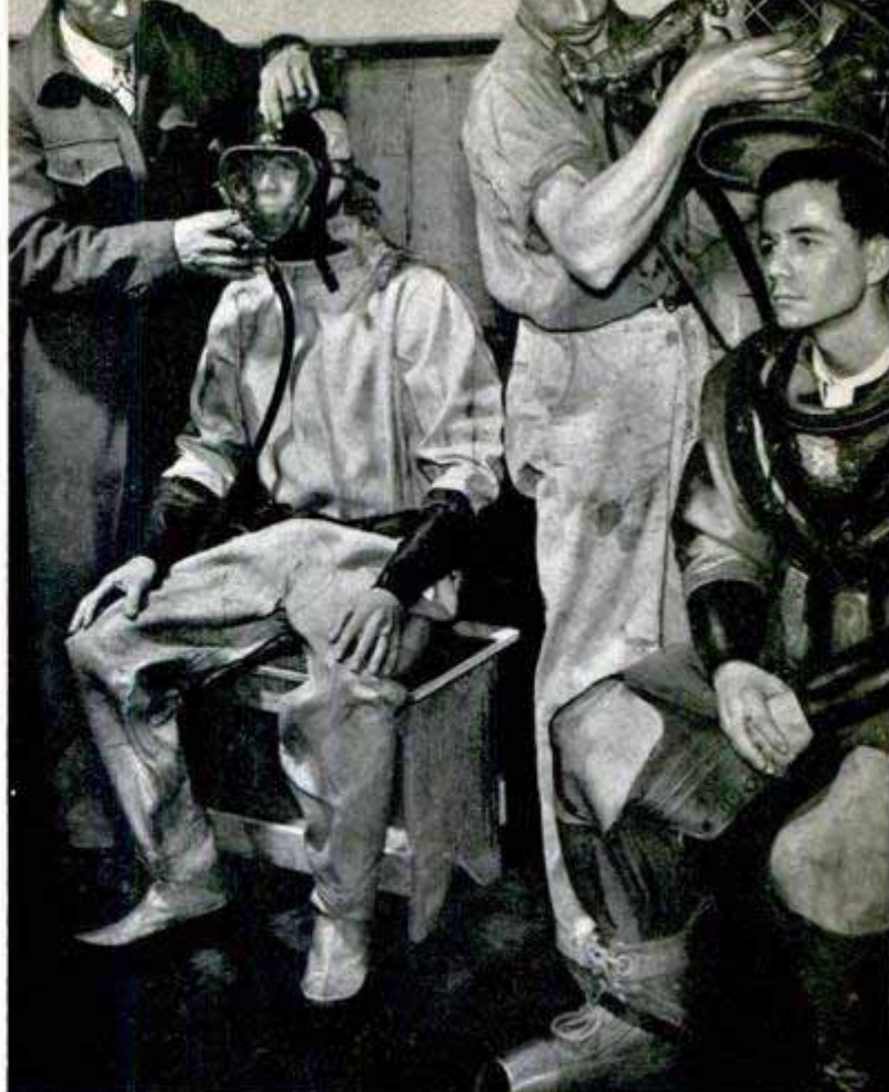
Student at left wears light suit for shallow work, while "deep sea" man at right wears 190-pound rig. Diver is given final instructions on the use of oxy-hydrogen underwater cutting torch for salvage work.
