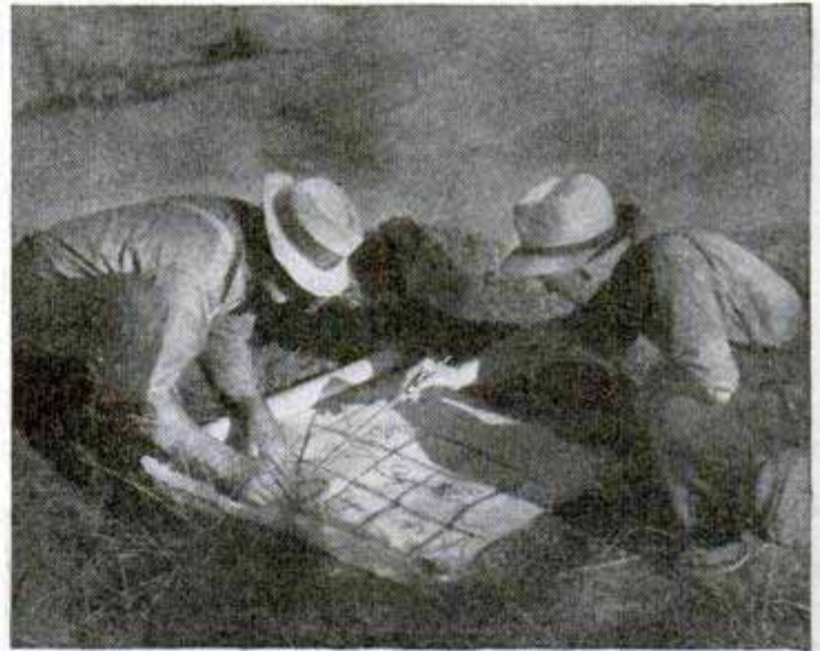
On a map of the area prospectors mark the spot where each sample is found. If assayer's report is favorable, area is searched for ore bodies. Below, streams may carry minerals, so water samples are collected
