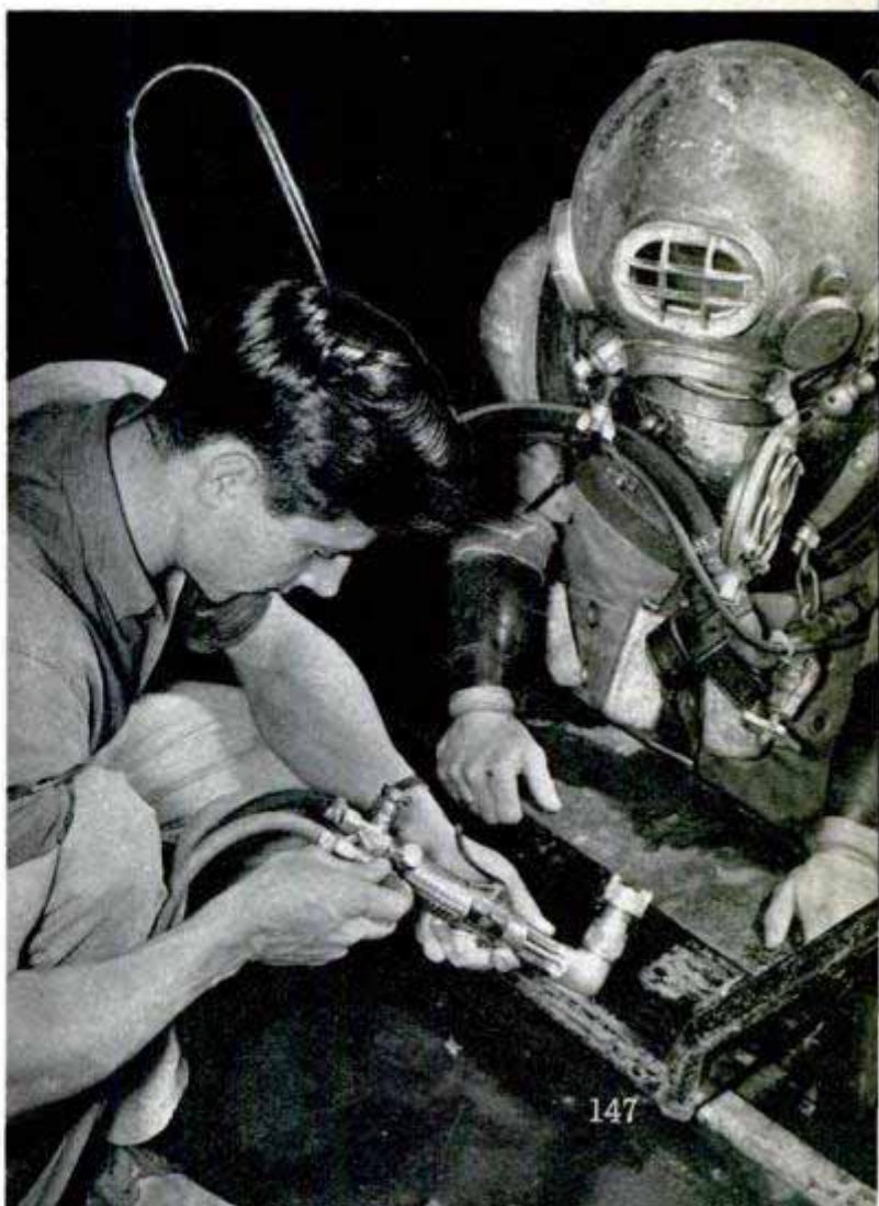
Student at left wears light suit for shallow work, while "deep sea" man at right wears 190-pound rig. Diver is given final instructions on the use of oxy-hydrogen underwater cutting torch for salvage work.
