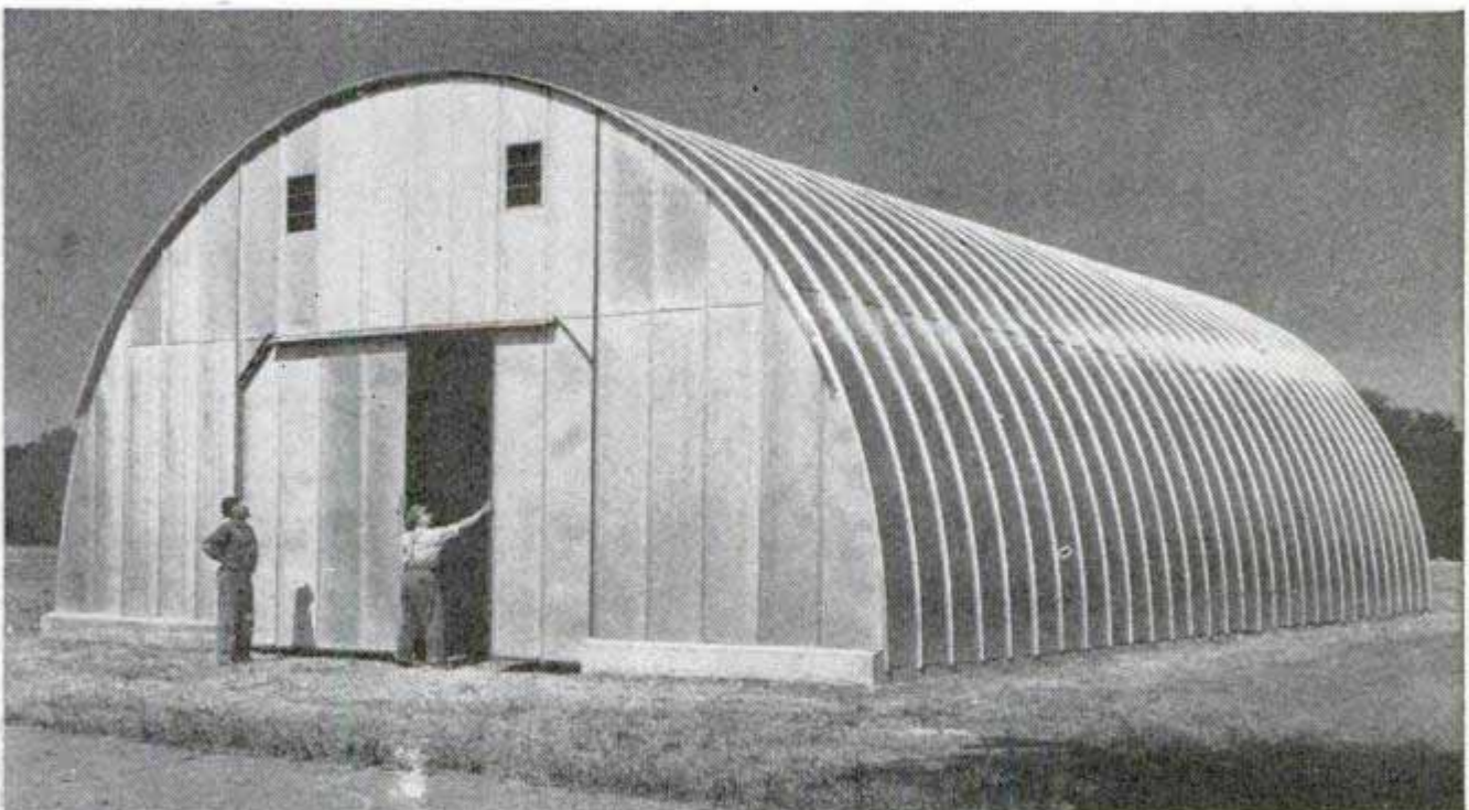
Completed aluminum building, erected in 150 man-hours, has big doors, over 2000 square feet of floor area
