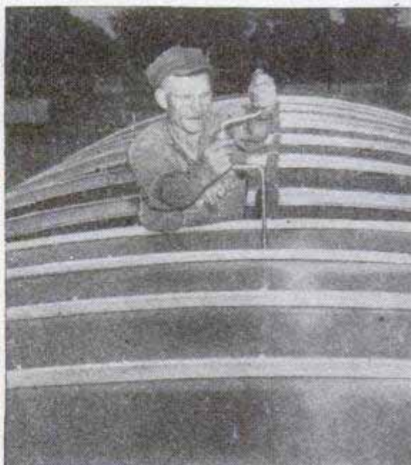
Right, builder tightens bolts across arch of roof. Below, same arch in cross section showing: A, bolt holding assembly together; B, arch cover called the "hat"; C, flanged sheet; D, arch frame; E, support member
