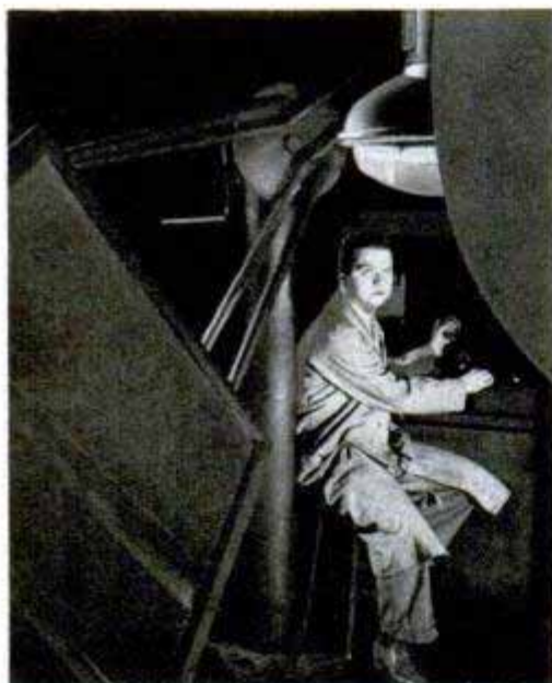
Street lights have to operate during all kinds of weather. A new model is tested for waterproofing under roof-top shower
