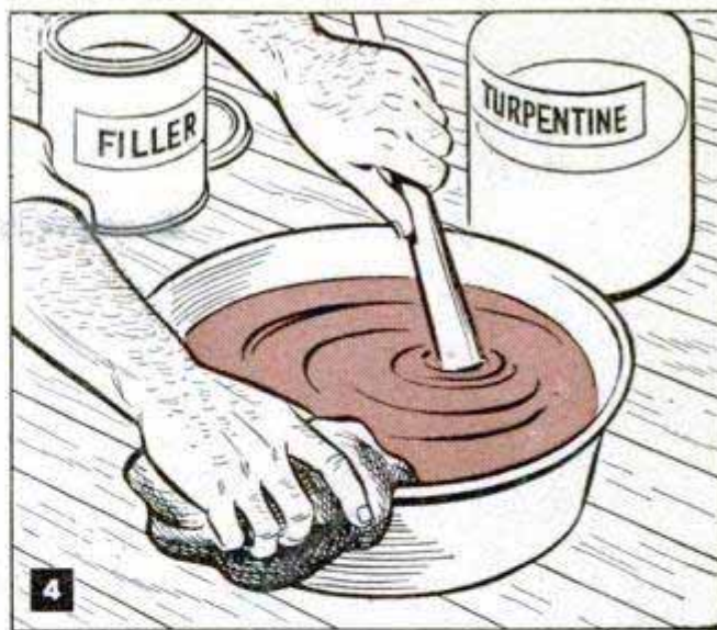
The filler should be reduced with turpentine to a light, creamy consistency. Stir thoroughly to dissolve all lumps, and stir the mixture occasionally while using
