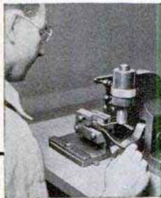
This shows how Crestoloy Pliers are individually tested for cutting ability before being boxed for shipment.
