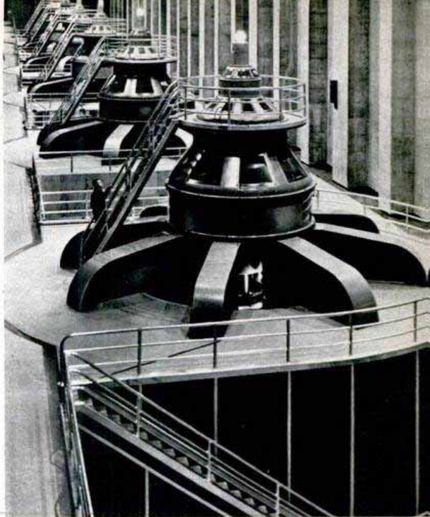
Big as a house, each 144,000-hp. generator at Grand Coulee turns water power into electricity. Boulder switching yard (below) is striking symbol of power
