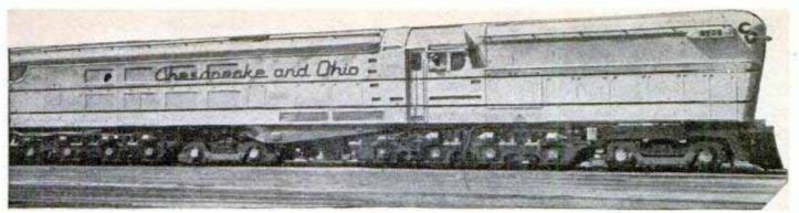
Top, the 154-foot "Chessie" sets a new style in steam engines. Forty wheels are needed to support its tremendous weight
