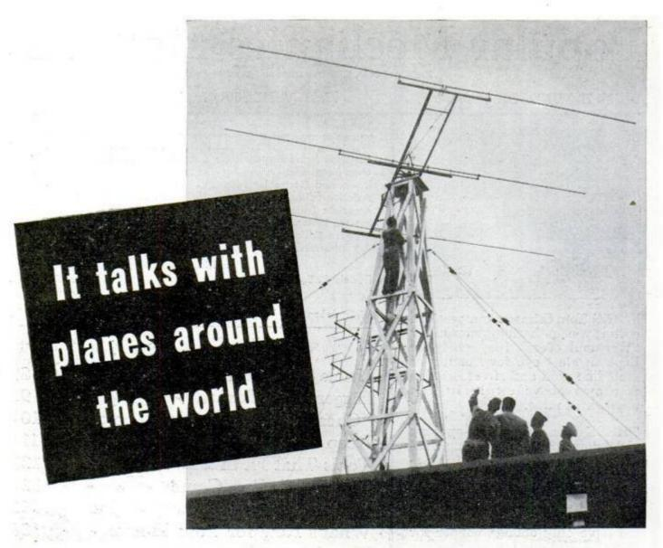
You're looking at a "rotary beam parasitic array antenna." What it does is big as its name. By high-frequency continuous-wave transmission, the Air Force can talk to planes anywhere on earth.
