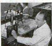
This student is testing for accuracy a Turn and Bank Indicator against time, using a stop watch, and against another instrument of known accuracy.
