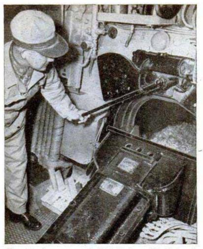
Above, the fireman opens the butterfly door of the firebox to show how stoker feeds coal onto table. Steam jets spread coal over fire automatically. Three holes in stoker tube enable him to watch flow of coal when door is closed. Below, loading arm is lowered into opened bunker during coaling at Clifton Forge
