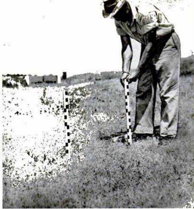
These two channels were exposed to the same flow of water, yet a gully a foot deep was scoured in the weeping lovegrass at the left, while the Bermuda grass at right shows no signs of damage from flowing water
