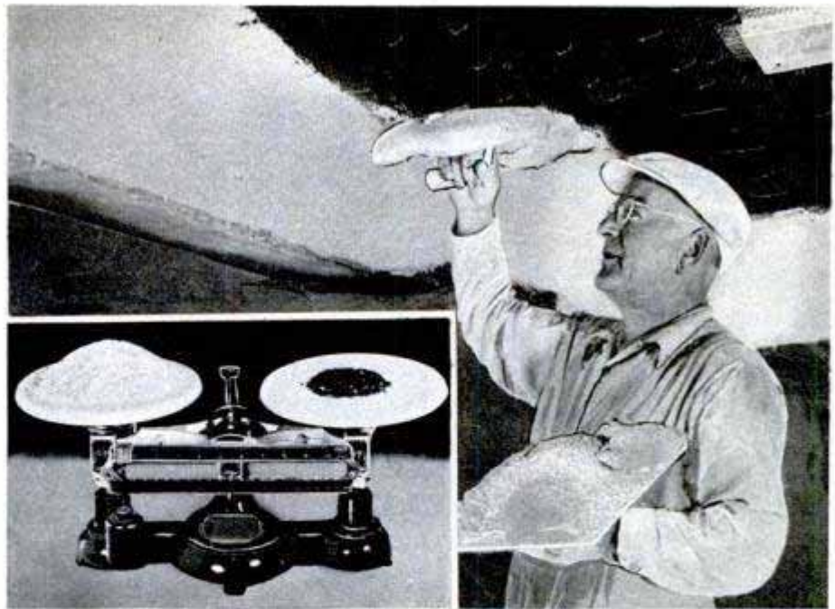
Insert shows how "popping" expands and whitens ore for mixing with plaster
