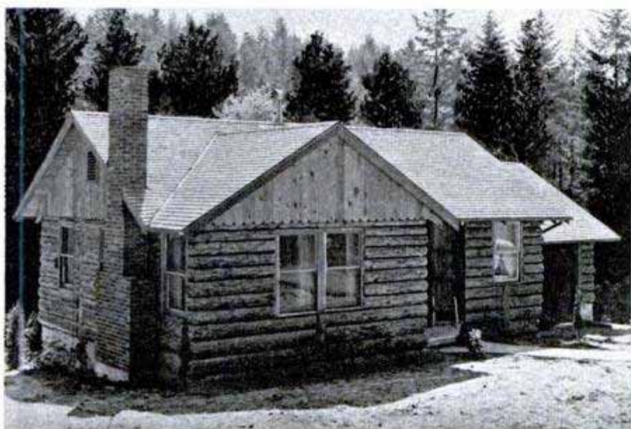
Top right, logs, squared on three sides, are held together by narrow wooden keys. Above, walls are erected quickly. Below, completed cabin
