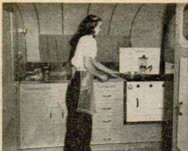
Left, all-metal kitchen has a built-in range, icebox and cupboards. Right, front view shows clearly the absence of heavy steel framework
