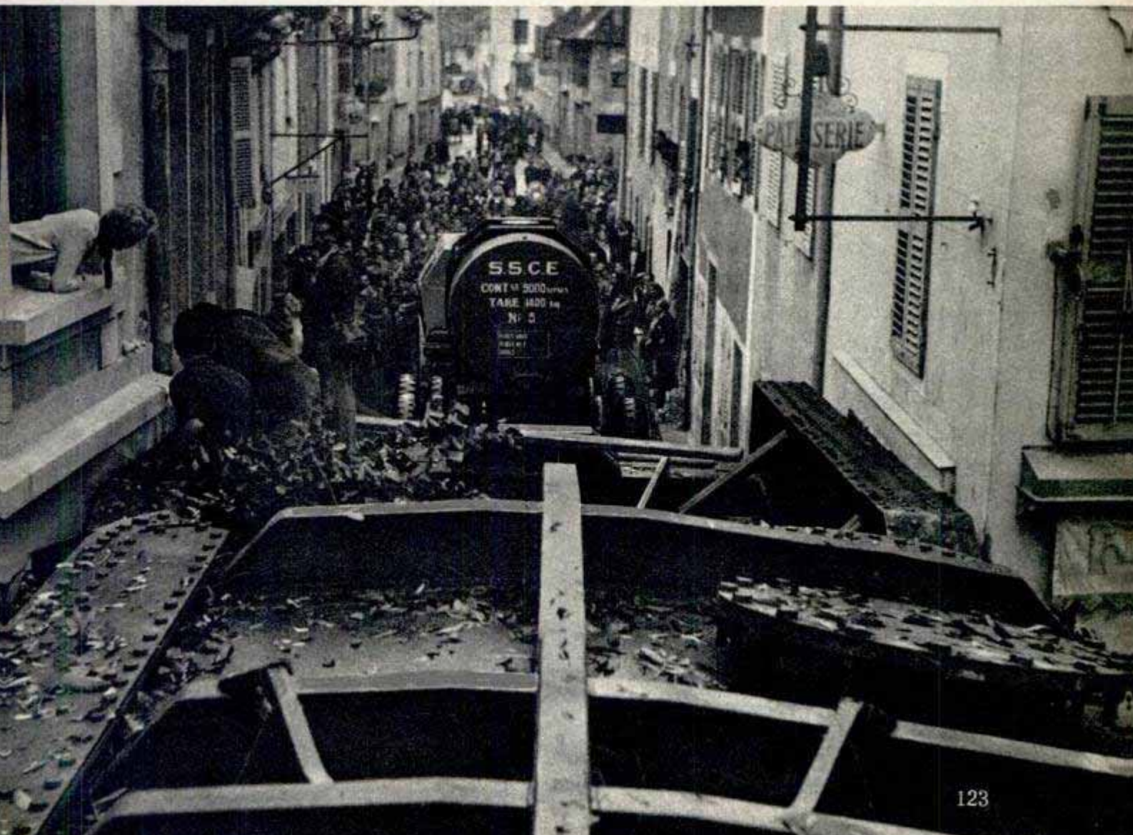
The tremendous weight caused this single-span bridge across the Rhone to sag only a fraction of an inch. With only one inch of clearance in this narrow street at Yenne, the expert drivers got the huge generator through without damage. A drainpipe on one of the houses was the only thing that was removed by the crew.
