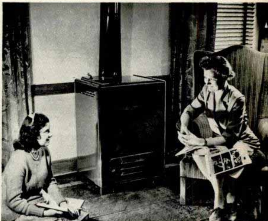
Even old-fashioned heating stoves are studied carefully to learn ways of bettering new designs. Right, the smokeless stove is another Battelle contribution. Smoke is burned to colorless gases before entering the flue
