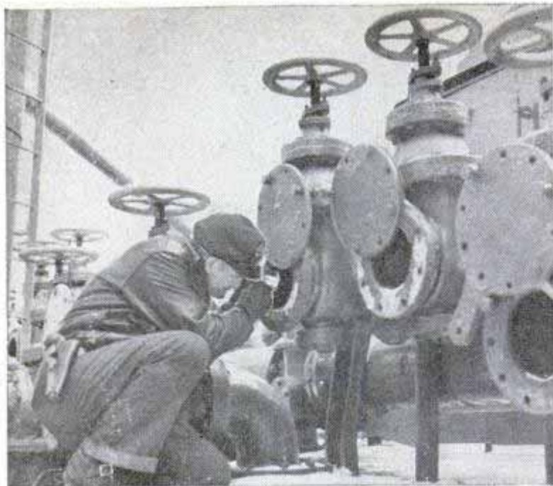
No nook is beyond the prying eyes of an inspector. Here the interior of a tanker's huge valve is checked for narcotics
