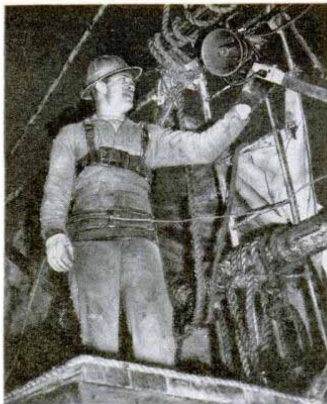
Despite the noise, a derrickman on his lofty perch can use the inter-com system to talk to the driller (below) who is shown flipping switch to give order
