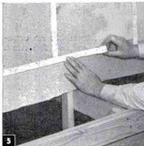
Above, foam rubber is held in place on vertical surfaces with linoleum cement. Abutting edges of sheets are held with 1-in. adhesive tape as shown below. This permits small pieces to be used
