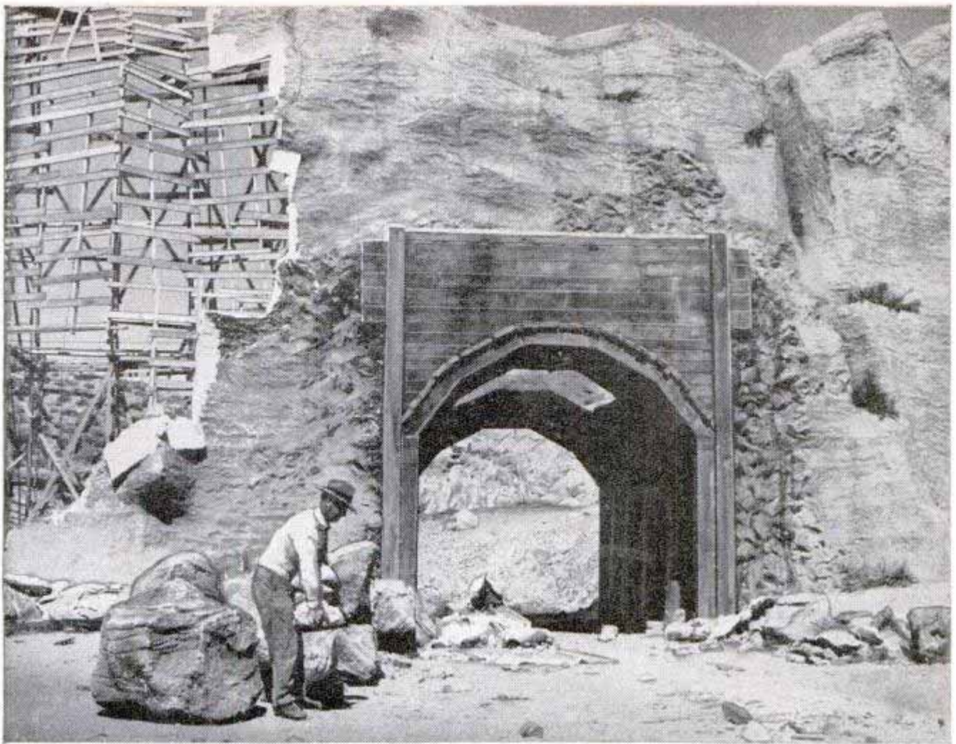
Windstorm damaged movie "mountain" revealing its flimsy wood framework covered with burlap and plaster
