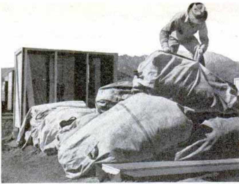
Workman unpacks fireproof canvas roofs for two-room sleeping tents
