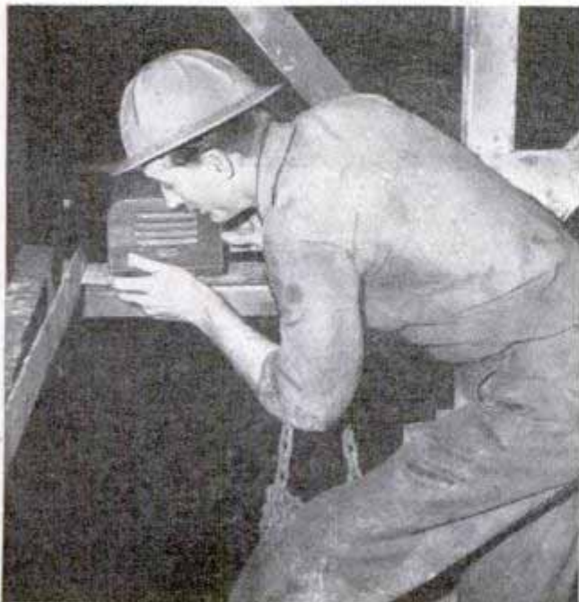
The engineman's speaker is on a long cord so it can be kept handy to receive driller's instructions. Below, speaker in cellar helps prevent many accidents
