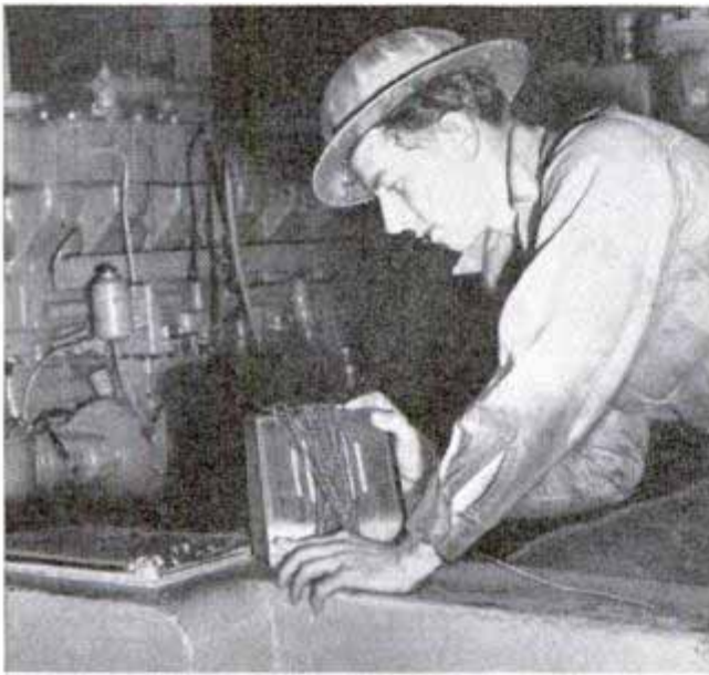
The engineman's speaker is on a long cord so it can be kept handy to receive driller's instructions. Below, speaker in cellar helps prevent many accidents
