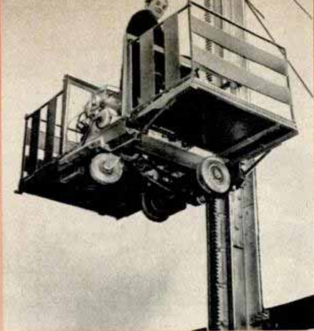
← Powered by a gasoline engine, the test model lifts inventor Bennett to the top of the vertical I-beam
