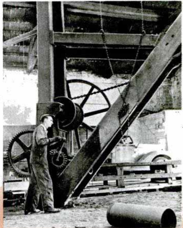
V & T shop equipment includes (left) steam plant kept in stand-by status in case of electric power failure, and (right) 75-year-old hand-operated wooden crane still in use; only base of the crane is shown in the photo
