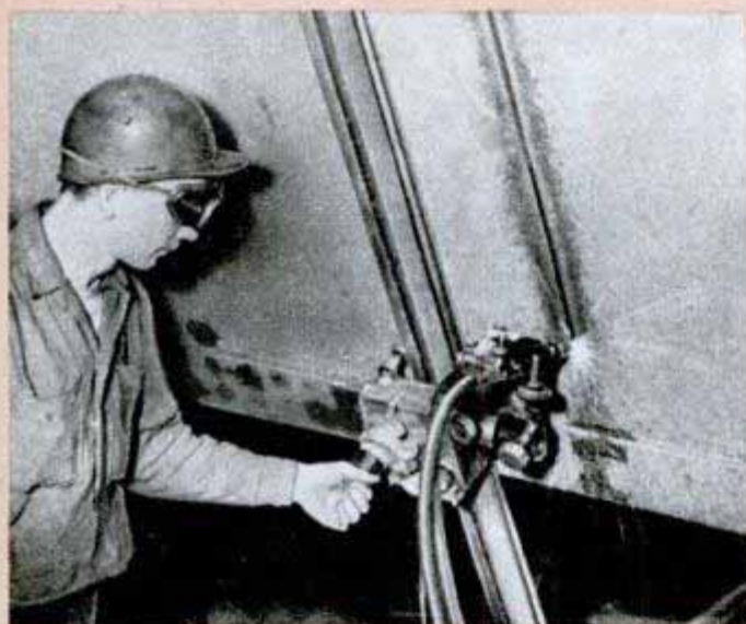
After a ship "can opener" (left) sears its way through the tough hull, a crane (right) removes the last severed section. Then the two halves are floated together (below, left), and the sections are welded together
