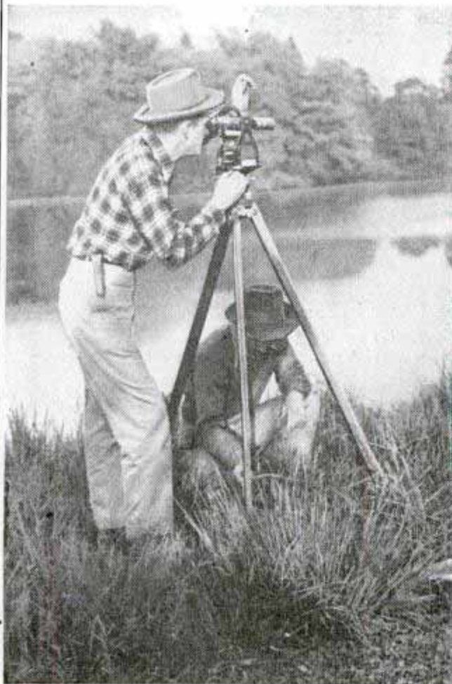
Photo at left shows the surveyor standing at point A shown in sketch above. Line AB is 2000 feet. After reading angle ABC, surveyor uses mathematics to compute line AC across river. Distance is 1773.9 feet
