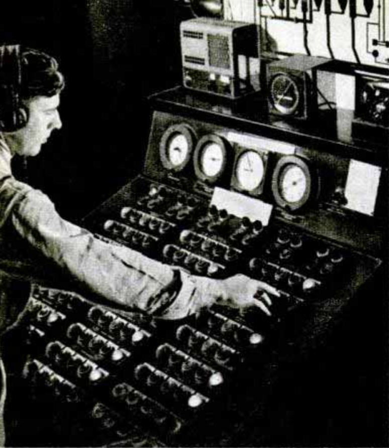
A large array of switches (left) control compressors and 24 valves of $2,000,000 supersonic wind tunnel at Aberdeen. Engineers at right are adjusting test missile in the model-working section of the big tunnel
