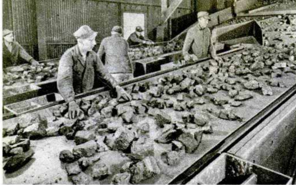
Above, workmen remove slate and other refuse from the coal as it moves on to the screen breakers where it is reduced to three inches or less in size. Below, conveyor belts distribute the coal into blending bins which mix it to insure the chemical uniformity needed for producing metallurgical coke
