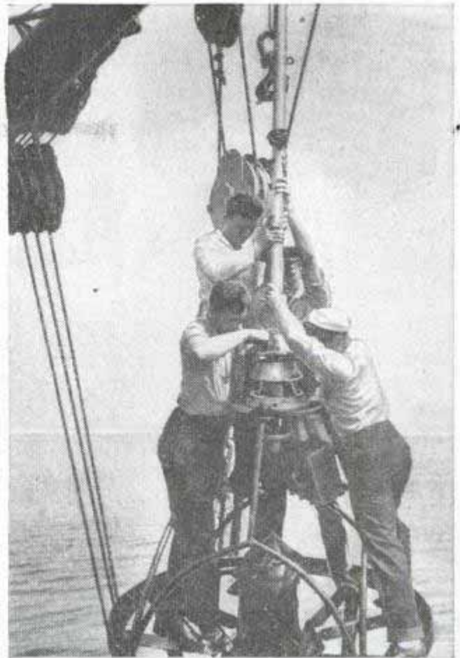
Installing antenna (above) and batteries (below) on radio-equipped buoy which aids navigation in fog
