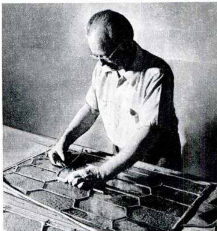
Placed in front of a light, the assembled sections are painted by Somers. Any mistake is costly as the pigment cannot be painted over. Below, after paint is baked, the sections are fixed in place with strips of came lead
