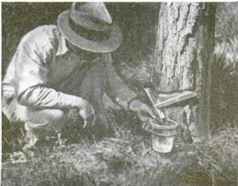
New bark-chipping hack was devised by Keith Dorman at the Olustee Experimental Forest in Baker County, Fla. Below, glass cup shaped like flowerpot catches oleoresin, or gum, from tree
