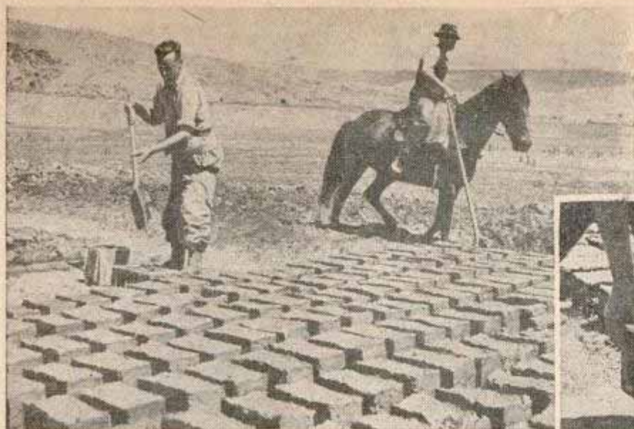
← Mud solves New Zealand's housing muddle: Farmers are building homes of mud bricks in a local process 70 years old. The field is plowed, watered. Then horses are ridden across it for two hours making a dough which (below) is molded into bricks
